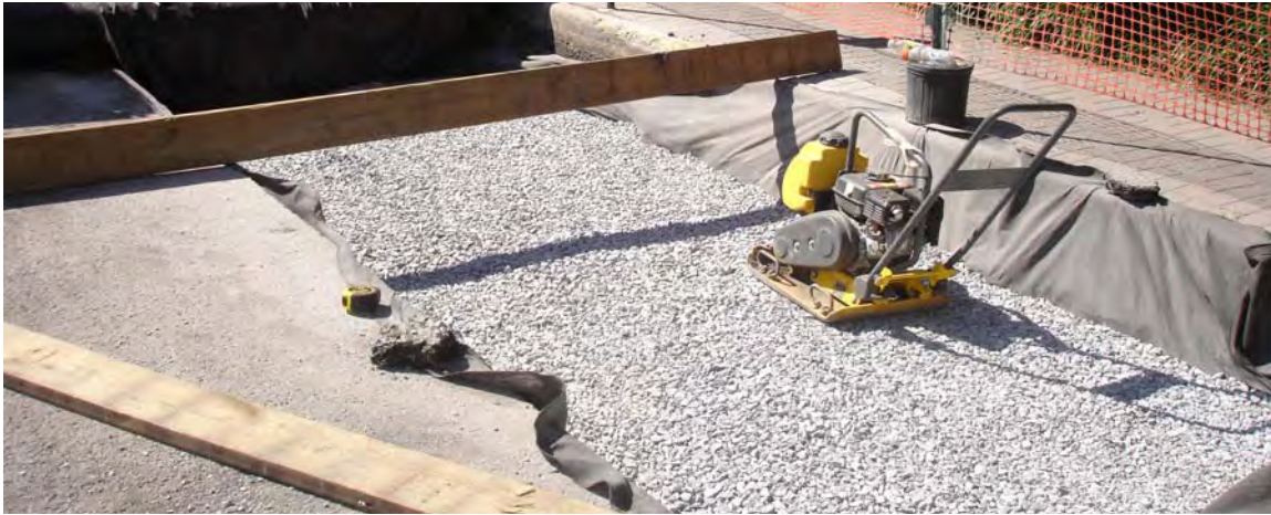
Figure 3-14: Mechanical tampers were used to install the gravel bed below permeable pavers at DPR's Olmsted Center in Queens.
