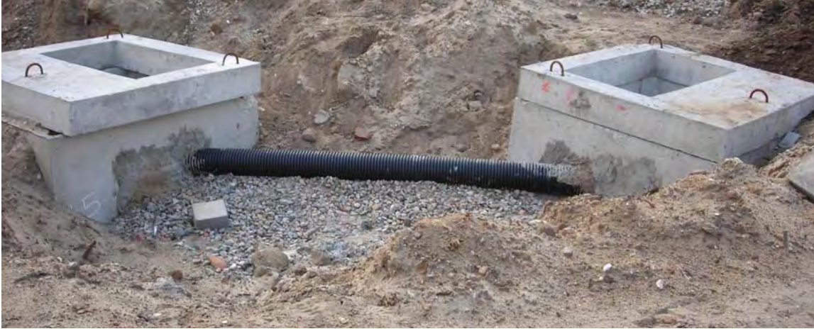
Figure 3-13: Catch basins installed to convey runoff to subsurface systems at Nehemiah Spring Creek Homes at Gateway Estates Phase 2 in Brooklyn.
