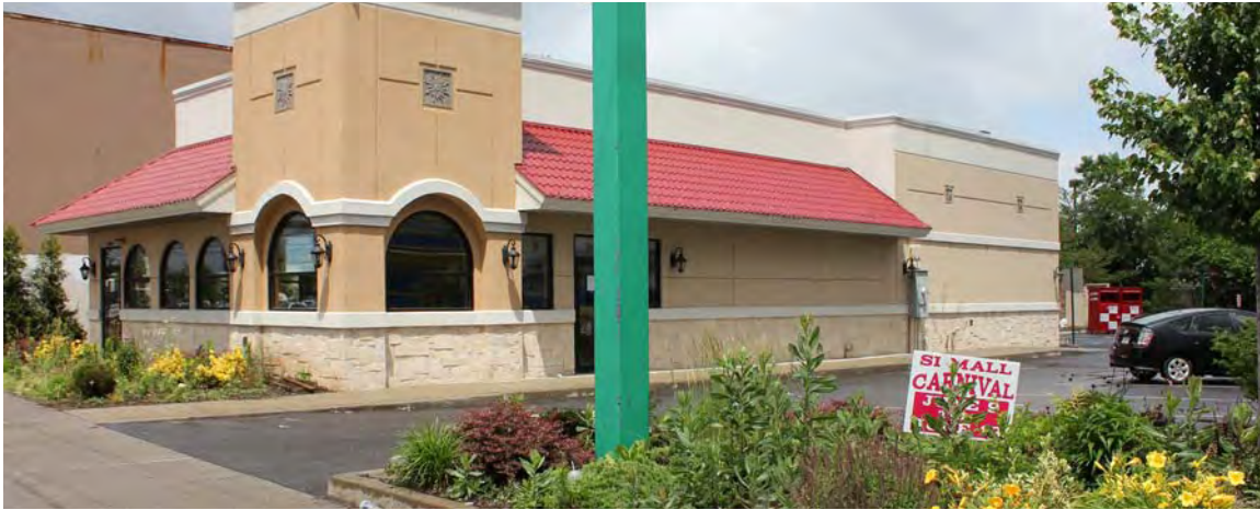
Figure 4-23: DCP's Parking lot requirements and impervious surface reductions may allow for smaller required storage volumes.
