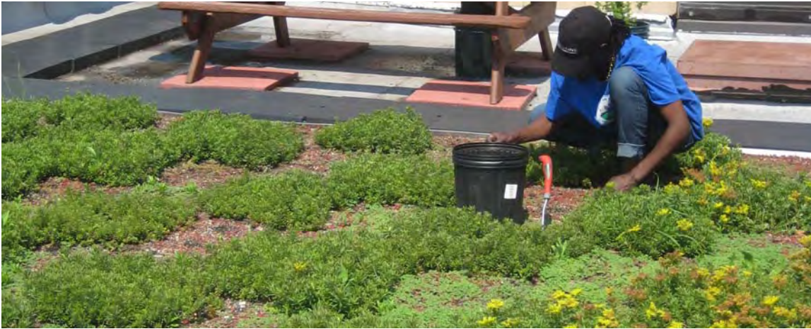
Figure 4-22: Staff performing maintenance on DPR's Five Borough Building green roof.
