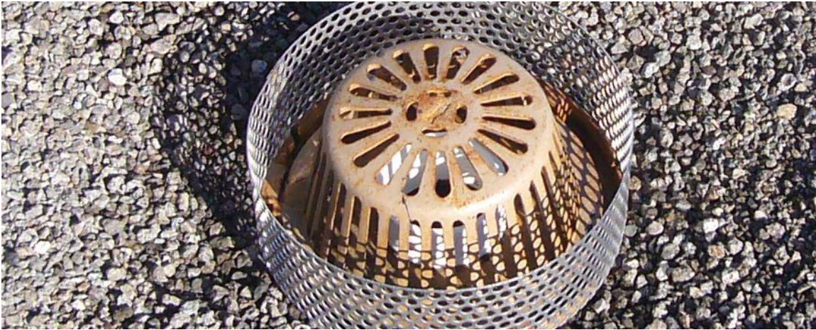
Figure 4-16: Roof drain screens and covers help prevent leaves and other debris from entering and clogging roof drains.
