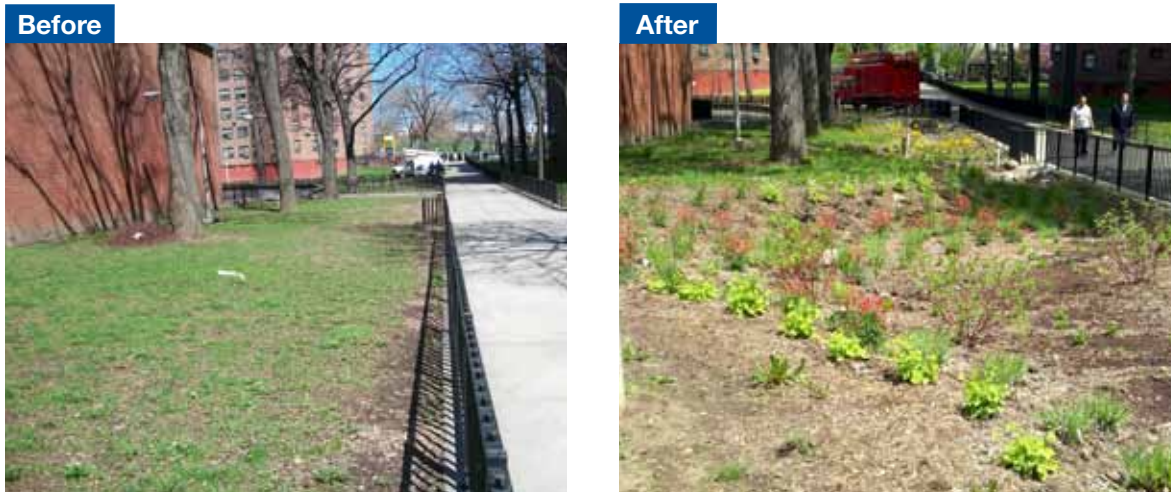
Figure 1-3: Pre and post-installation photos of open space converted to rain gardens at NYCHA's Bronx River Houses.
