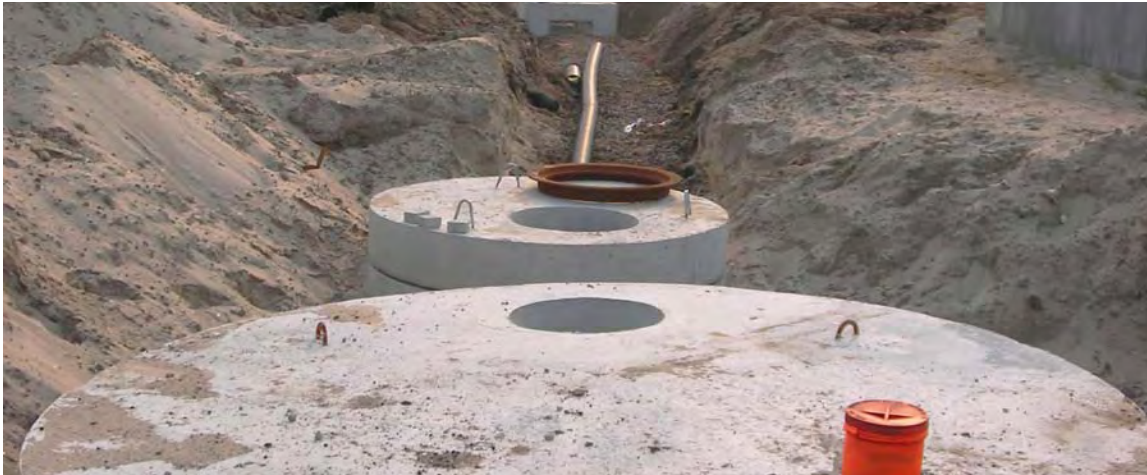
Figure 3-1: Subsurface storage vaults installed at Nehemiah Spring Creek Homes at Gateway Estates Phase 2 in Brooklyn, an affordable housing development sponsored by HPD and the Nehemiah Housing Development Company.
