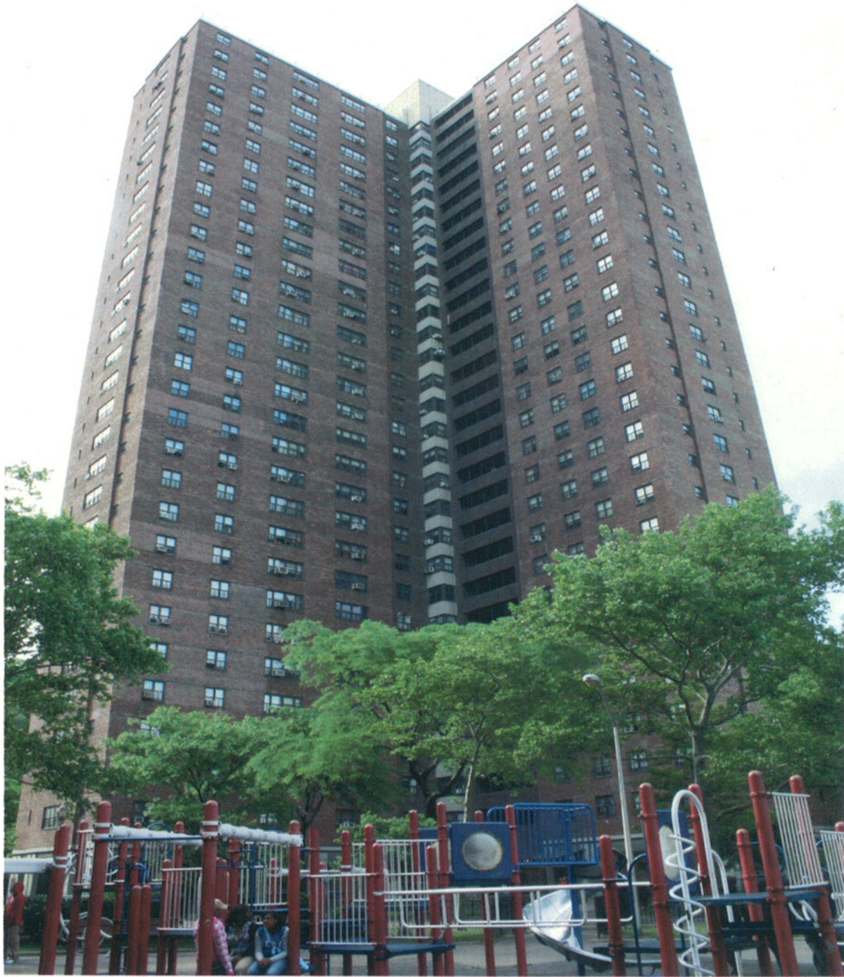
Polo Grounds Towers, Borough of Manhattan
