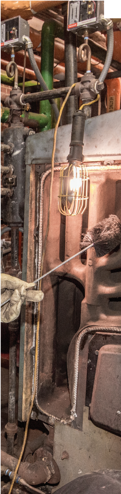
Boiler Maintenance at Brooklyn War Memorial Source: DCAS
