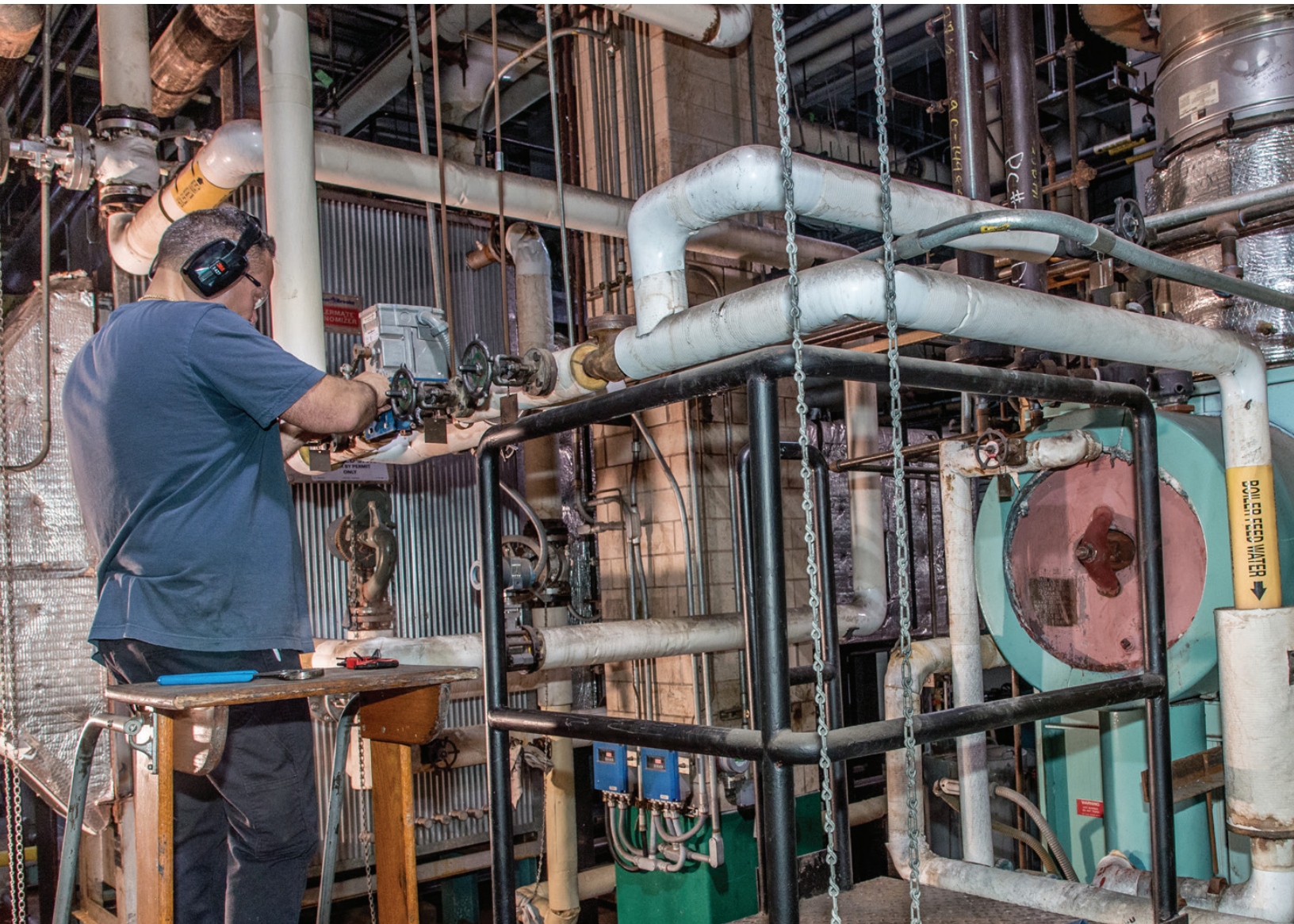
DCAS staff performing preventative maintenance on a boiler | Source: DCAS
