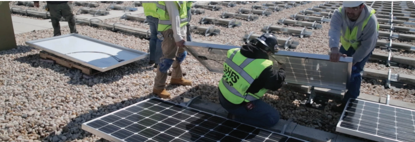
Solar panel installation at Queens Rachel Carson Intermediate School | Source: DCAS
