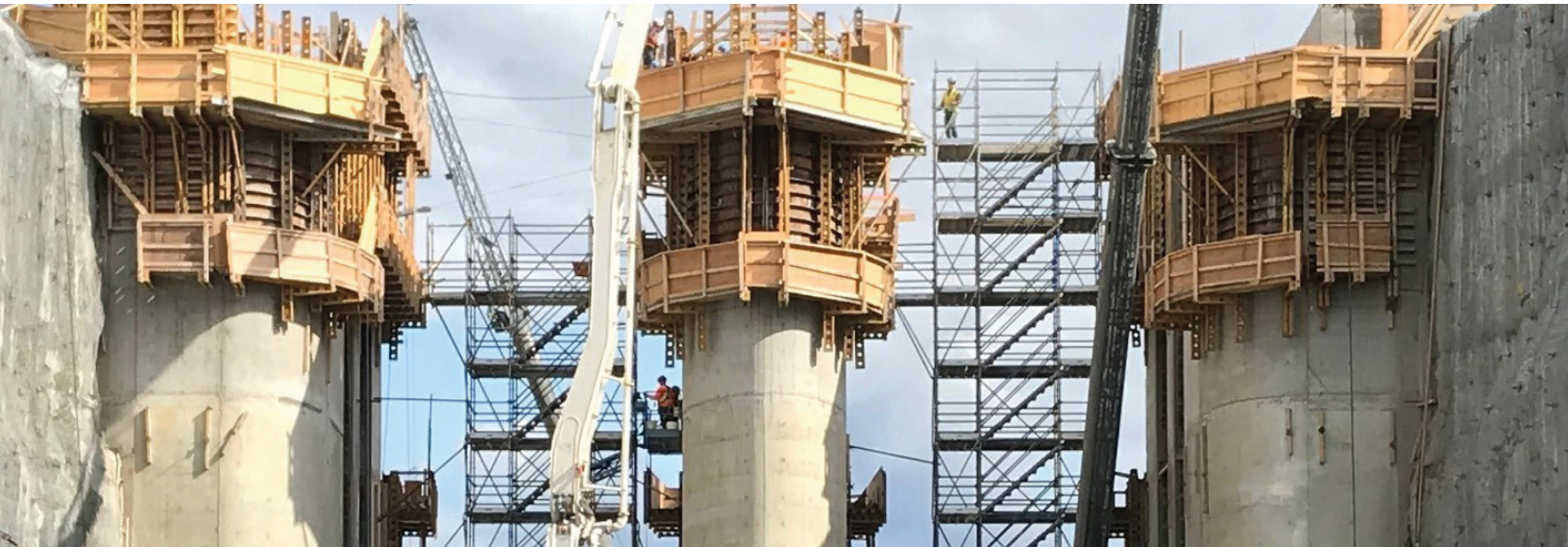
Hydropower dam construction | Source: DCAS
