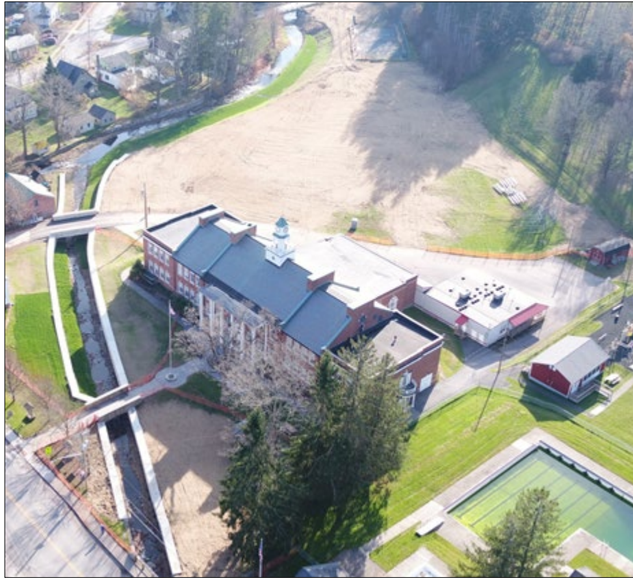
Figure 4.10 Aerial view of the completed Liddle Brook project.
