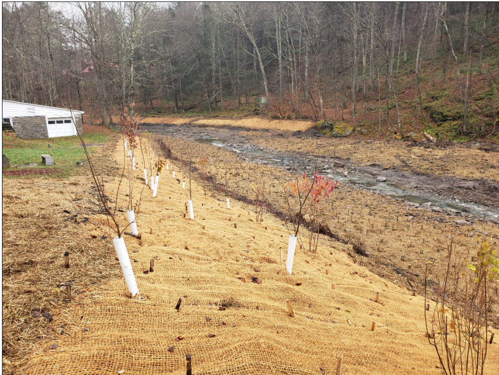
Figure 4.6 Elk Bushkill project before and after restoration.
