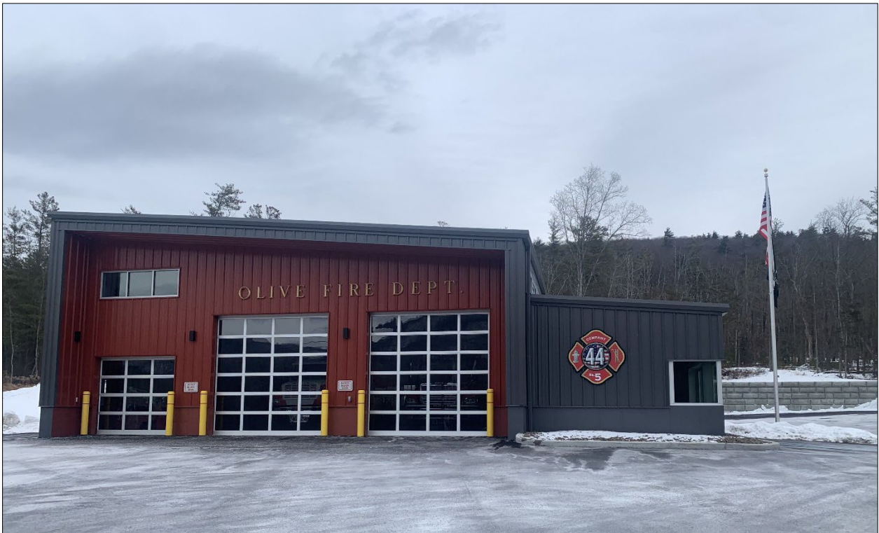
Figure 4.11 Eastern side entrance of the completed Boiceville firehouse in November 2023.
