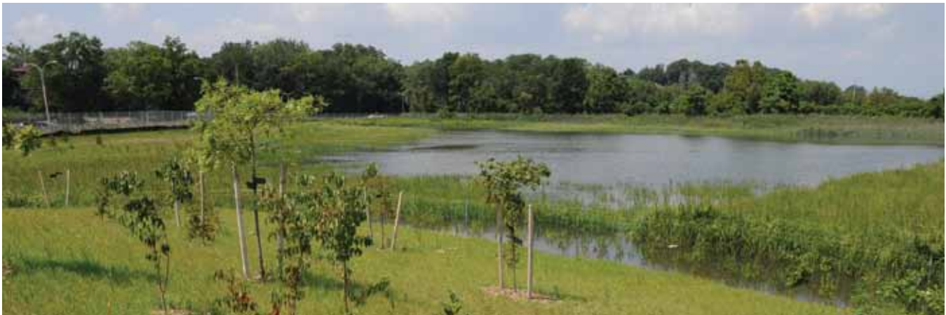
DEP restored wetlands and reintroduced local plant life to a 16-acre section of Alley Pond Park in Bayside, Queens to reduce combined sewer overflows into Alley Creek and Little Neck Bay.
