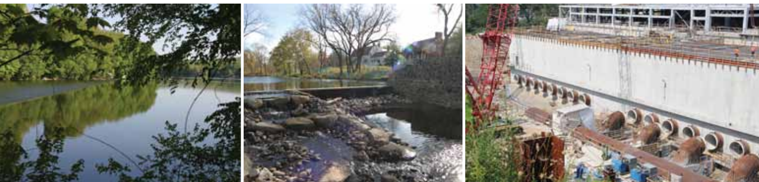
New York City's water is delivered from watersheds that extend more than 125 miles from the city and comprise 19 reservoirs and three controlled lakes. Our new water filtration and ultraviolet disinfection plants will ensure that NYC's supply of water meets stringent federal guidelines. Opposite: the Ashokan Reservoir.
