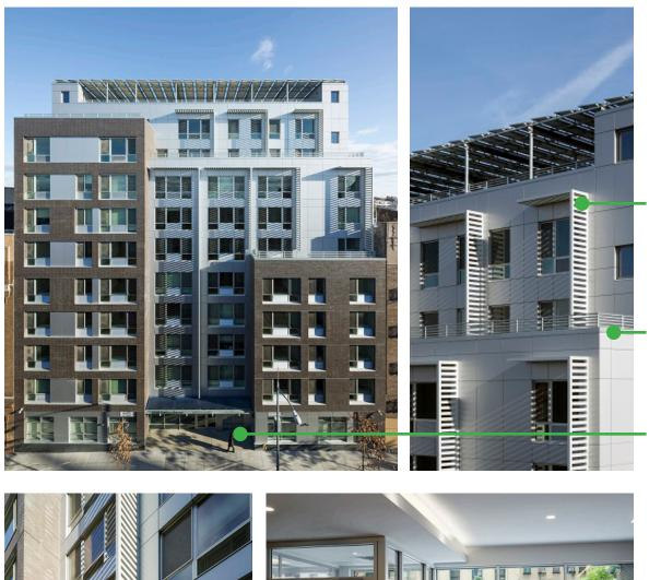
solar screens to mitigate heat gain within units
