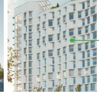
facade design helps minimize heat gain within units and could be used as inspiration for nonstandard balcony projections.
