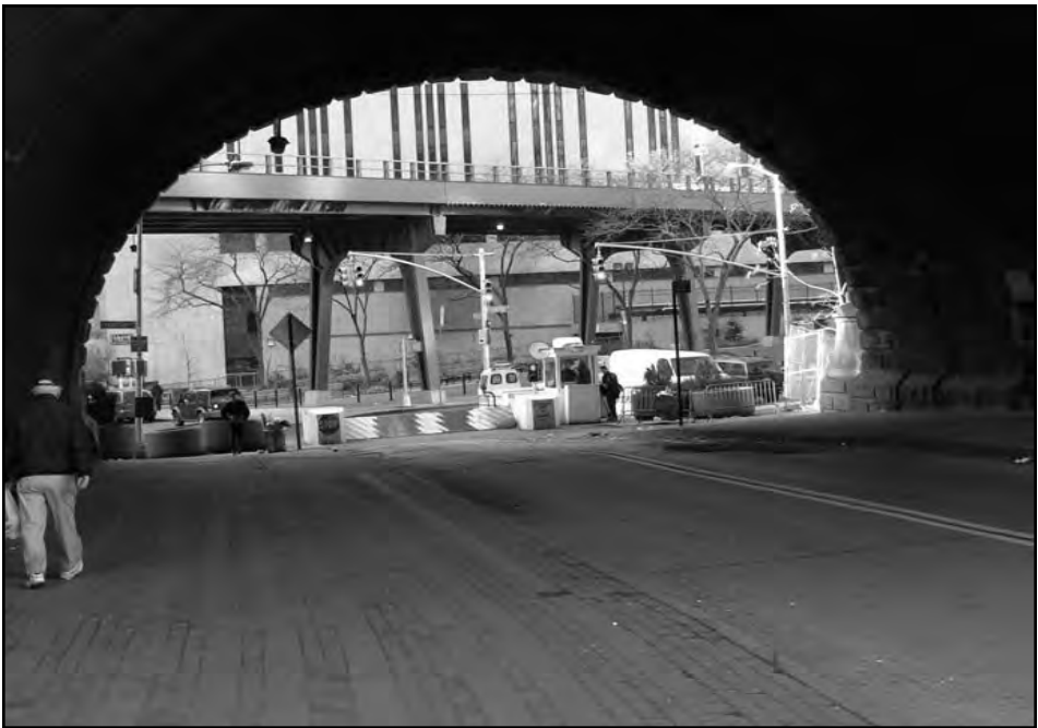
11. View south on Rose Street at Avenue of the Finest
