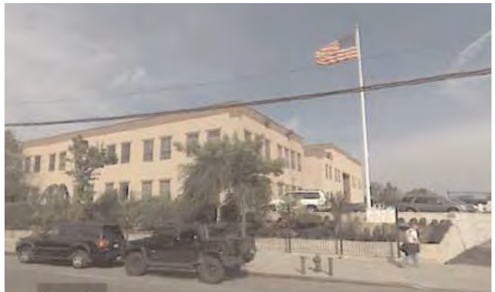
2. Street view of the office building located on the east side of Ulmer Street between 28th Avenue and 25th Avenue.
