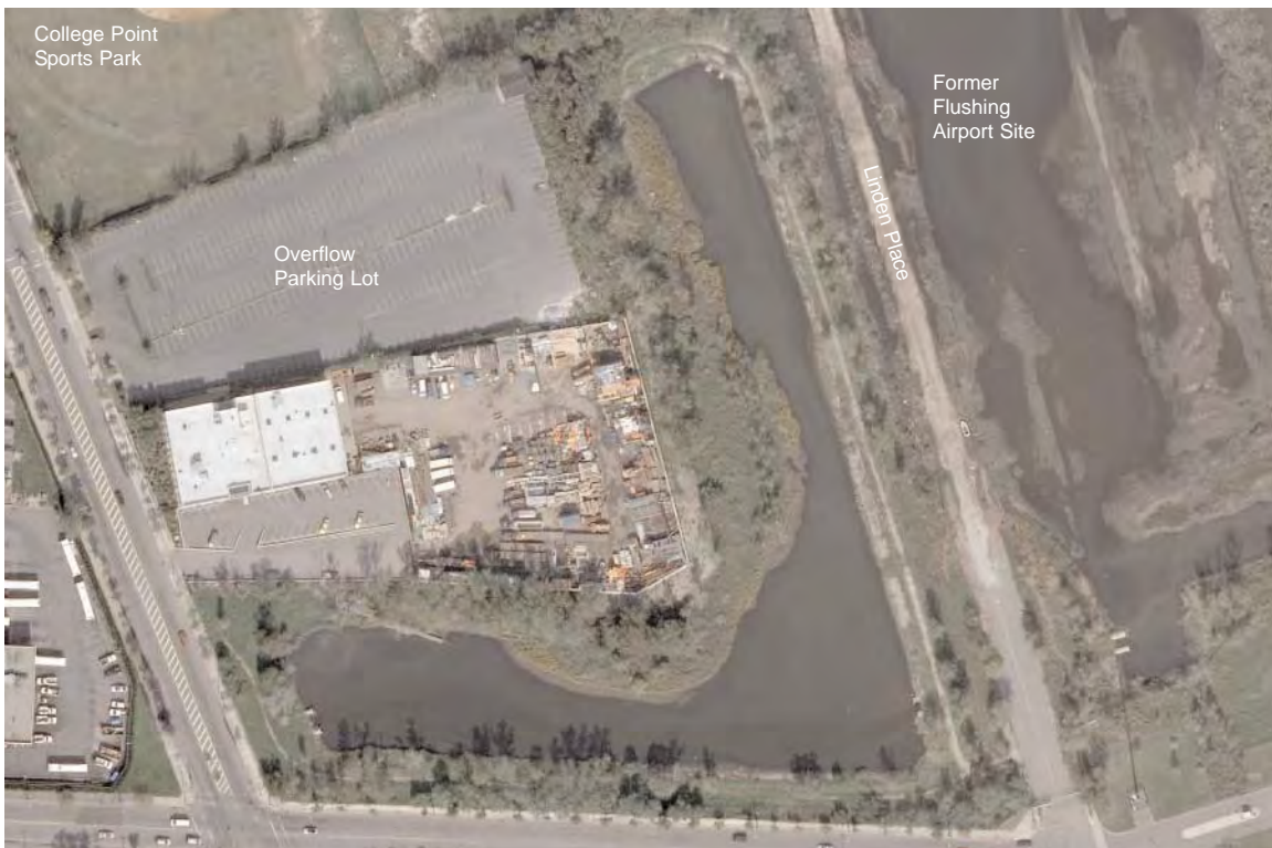
2. An aerial view of the off-site waterway that is located to the northeast of the proposed Academy site. Linden Place will be reconstructed to the east of the waterway. A portion of the flooded former Flushing Airport site is visible along the right side of the photo.
