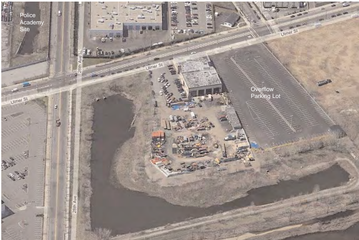
1. A birdseye view from the east of the off-site waterway that is located to the northeast of the proposed Academy site. The waterway is connected to the on-site drainage ditch via culverts that flow diagonally beneath Ulmer Street and 28th Avenue to the proposed Academy site.
