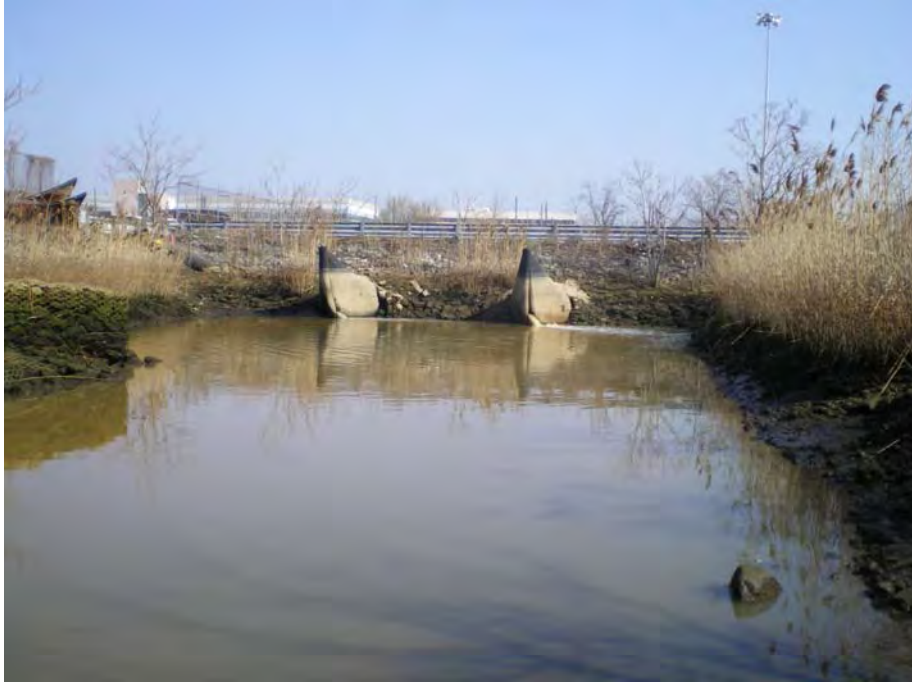
Site Photograph 5-4: Looking north at the northern crossing of drainage ditch. Note attached tide gates.
