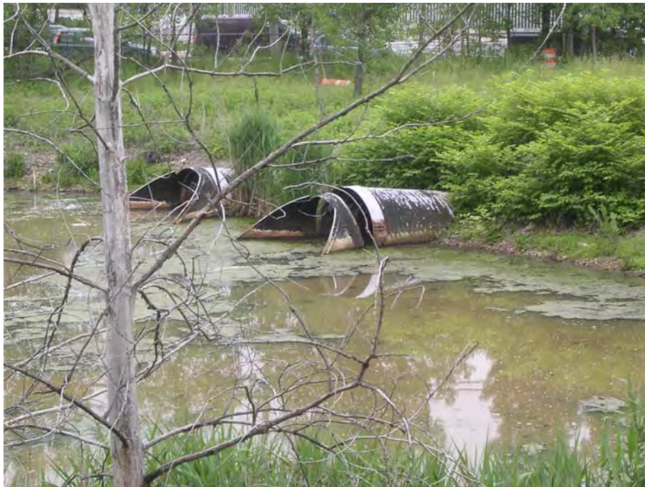
Photo 5-9: Culverts in "V-Shaped" detention pond northeast of Project Site.
