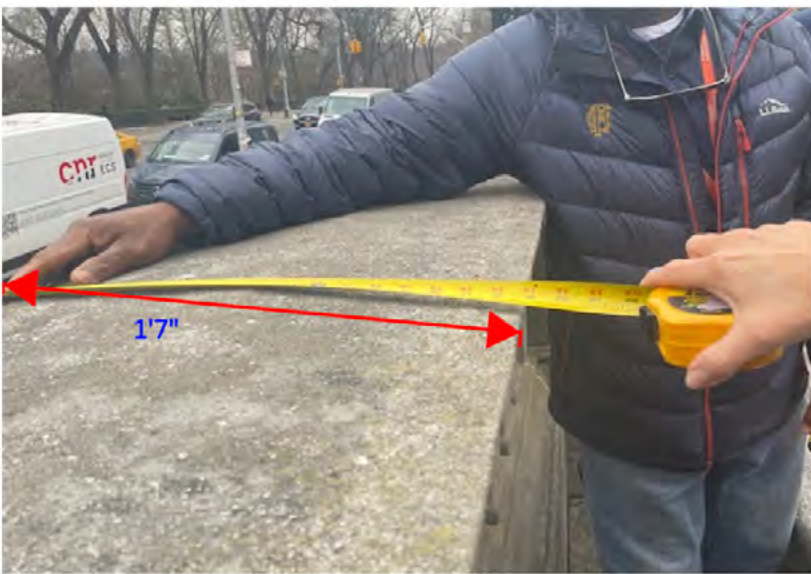
ONSITE FIELD MEASUREMENT OF BALUSTRADE
