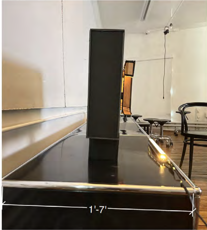
LOI FULL SCALE MOCKUP SIDE ELEVATION - LIGHTING NEEDS TO BE PLACED CLOSE TO THE EDGE OF THE LEDGE IF THE SIGNAGE IS CENTERED ON THE LEDGE
