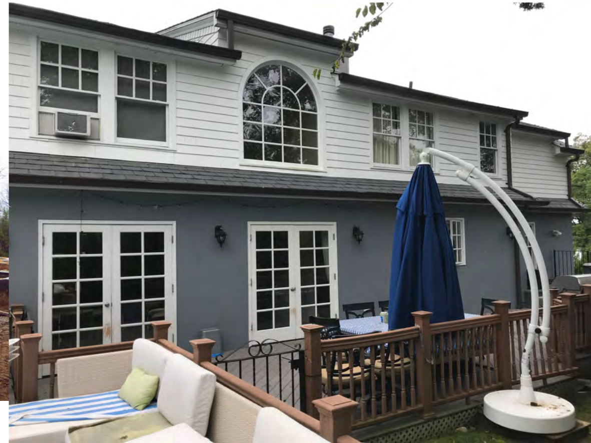
AS BUILT FROM WOOD DECK AT REAR
