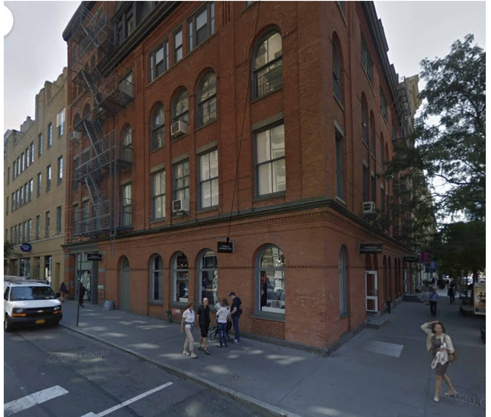
EXISTING CONDITIONS- PRINCE STREET SEPTEMBER 2014
