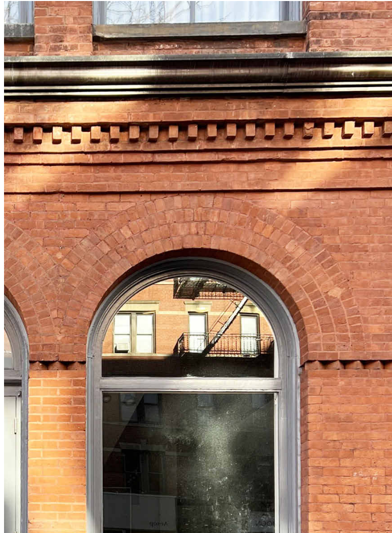
EXISTING CONDITIONS- TYPICAL BRICKWORK
