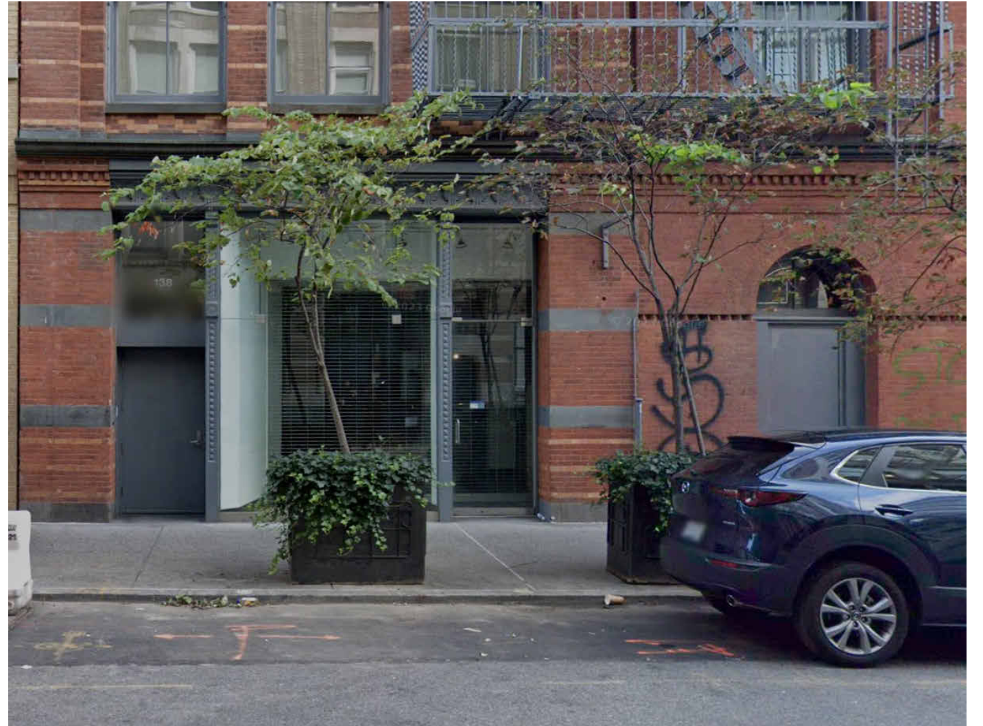
EXISTING CONDITIONS- PRINCE STREET STOREFRONT
