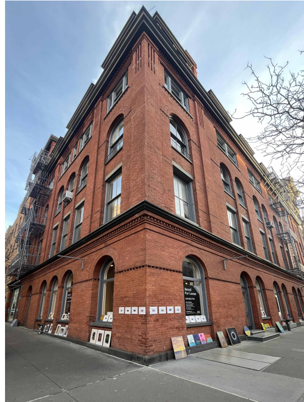
EXISTING CONDITIONS- PRINCE STREET & WEST BROADWAY
