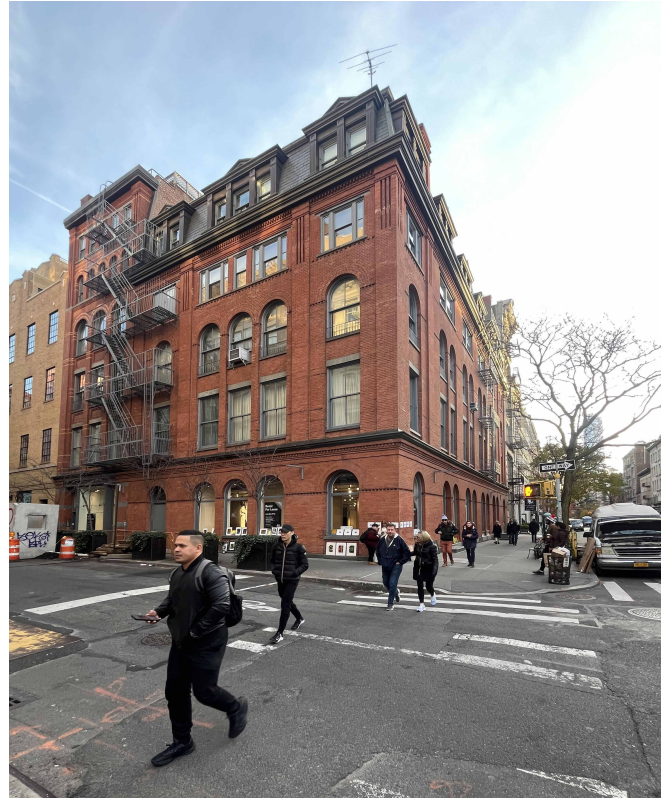
EXISTING CONDITIONS- PRINCE STREET & WEST BROADWAY
