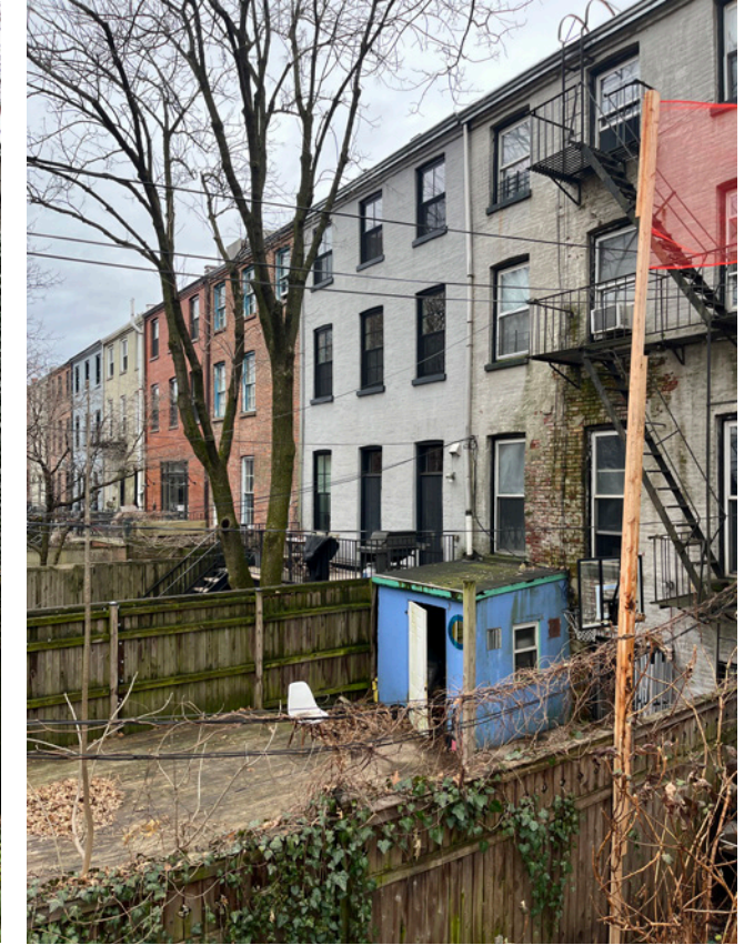
4. EXISTING REAR YARD: VIEW TOWARD
