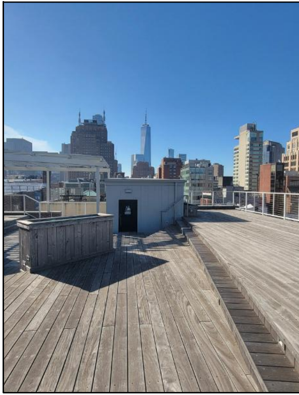
1 VIEW OF PASSENGER ELEVATOR FROM NORTH SIDE
