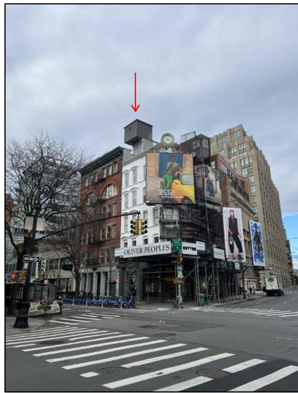
18 VIEW FROM CORNER OF W BROADWAY & WATTS ST LPC-19-20218
