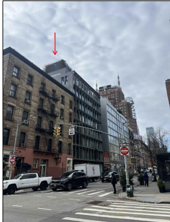
22 VIEW FROM CORNER OF W BROADWAY & GRAND ST NEW CONSTRUCTION
