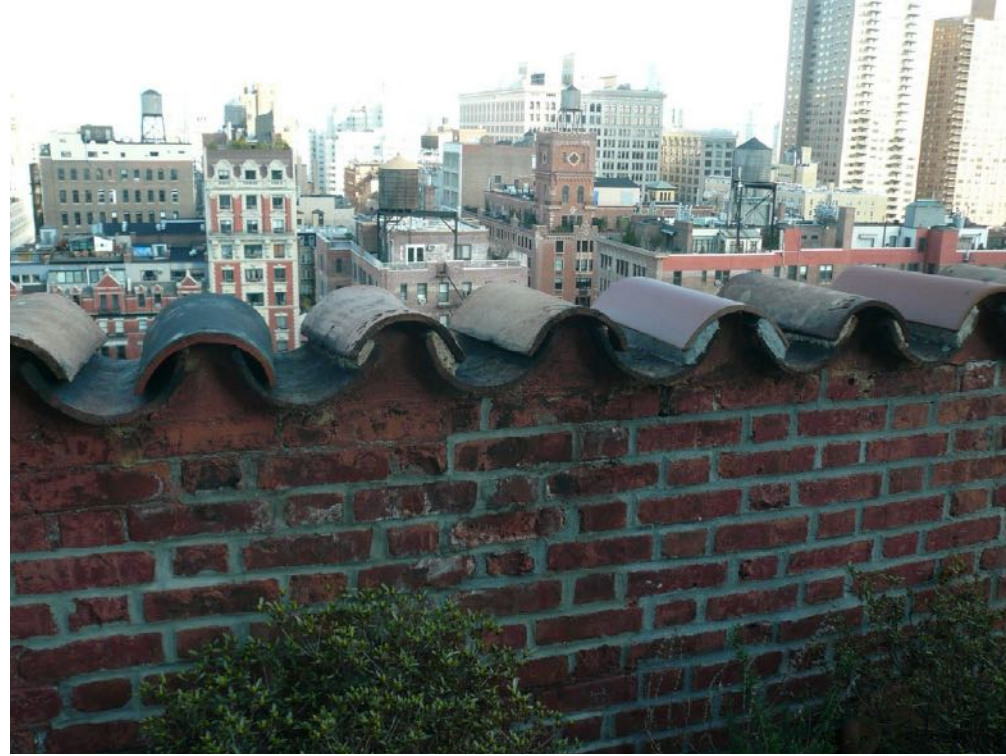
DETAIL VIEW OF EXISTING PARAPET WALL
