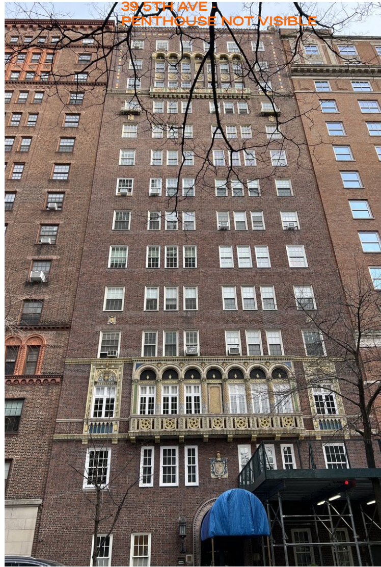
2: VIEW FROM 5TH AVENUE AND 11TH ST LOOKING EAST
