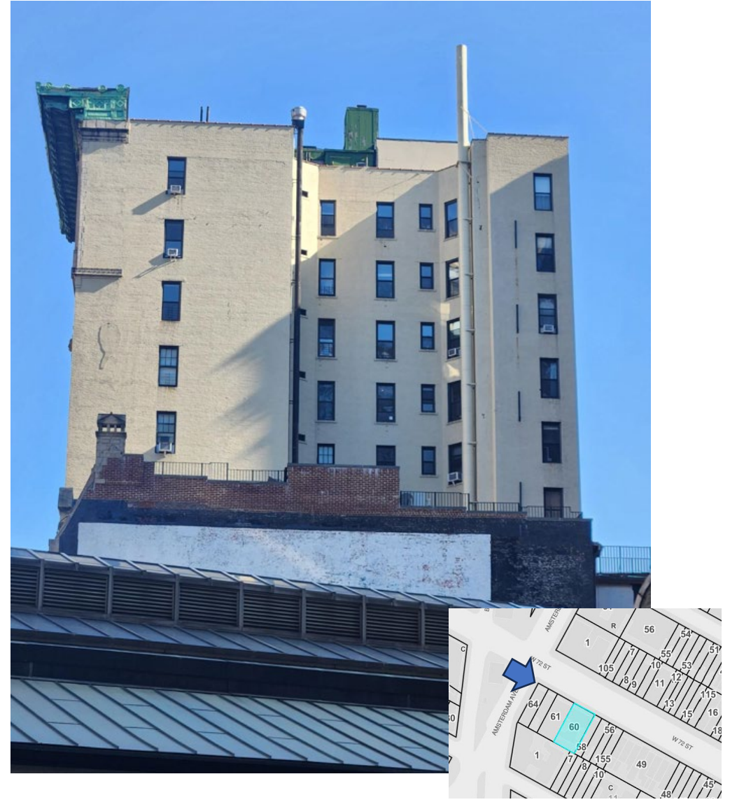
Proposed View of West Facade via Broadway - 2024
