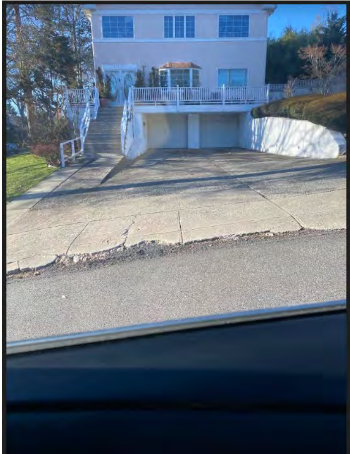
231-05 Hillside Avenue / Center Drive
