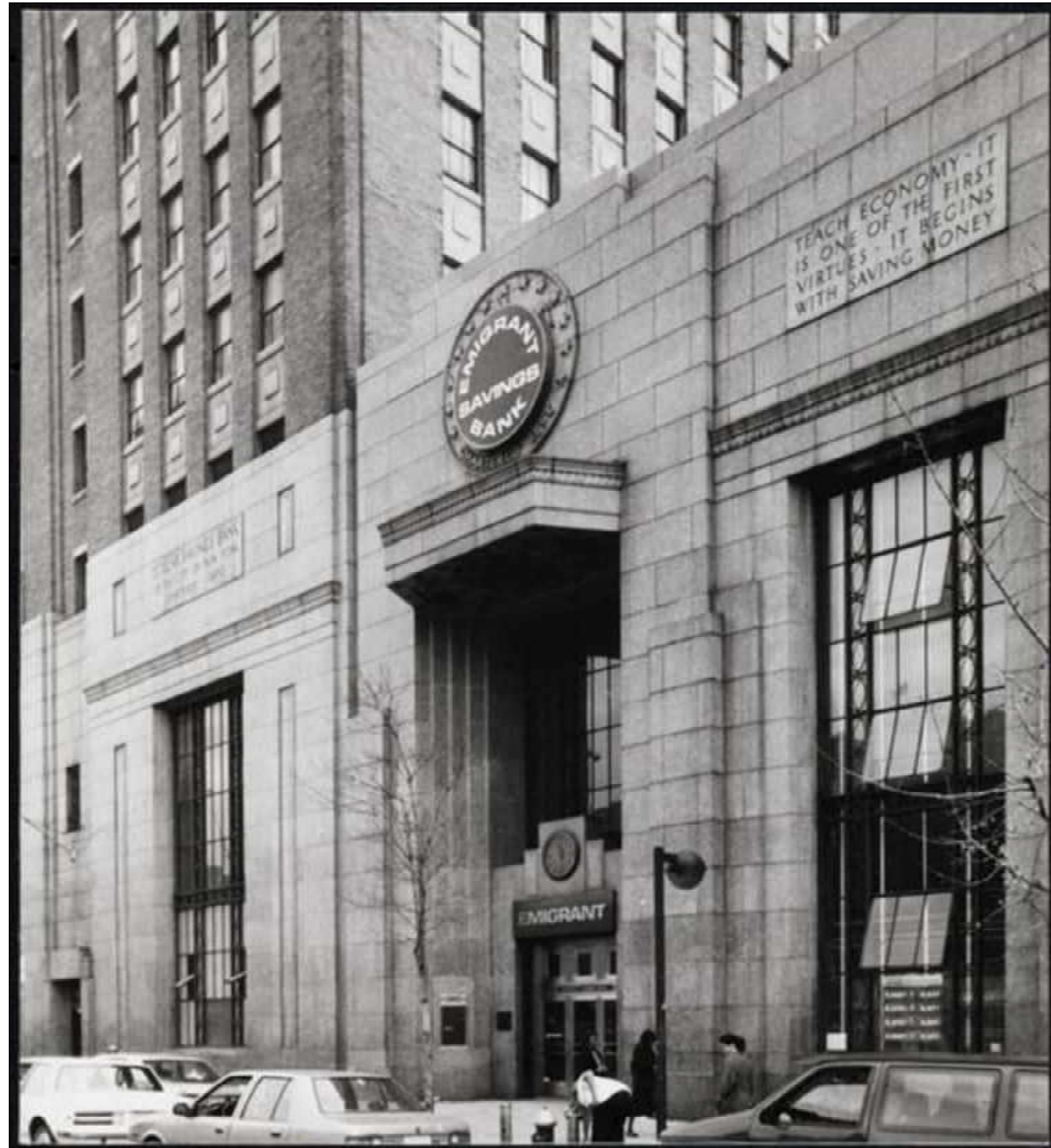
HISTORIC PHOTO WEST VIEW LATE 1984's
