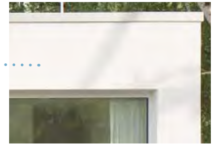
LIGHT STUCCO SIDING WITH PAINTED METAL FASCIA.
