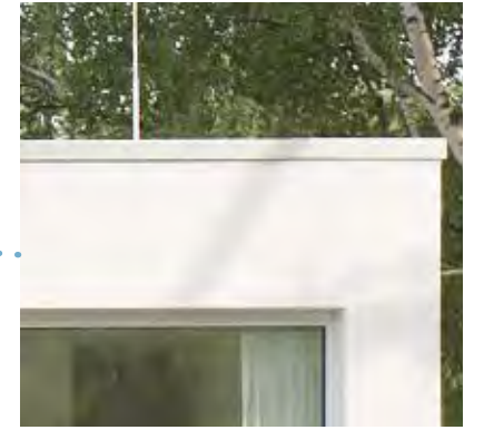
LIGHT STUCCO SIDING WITH PAINTED METAL FASCIA.
