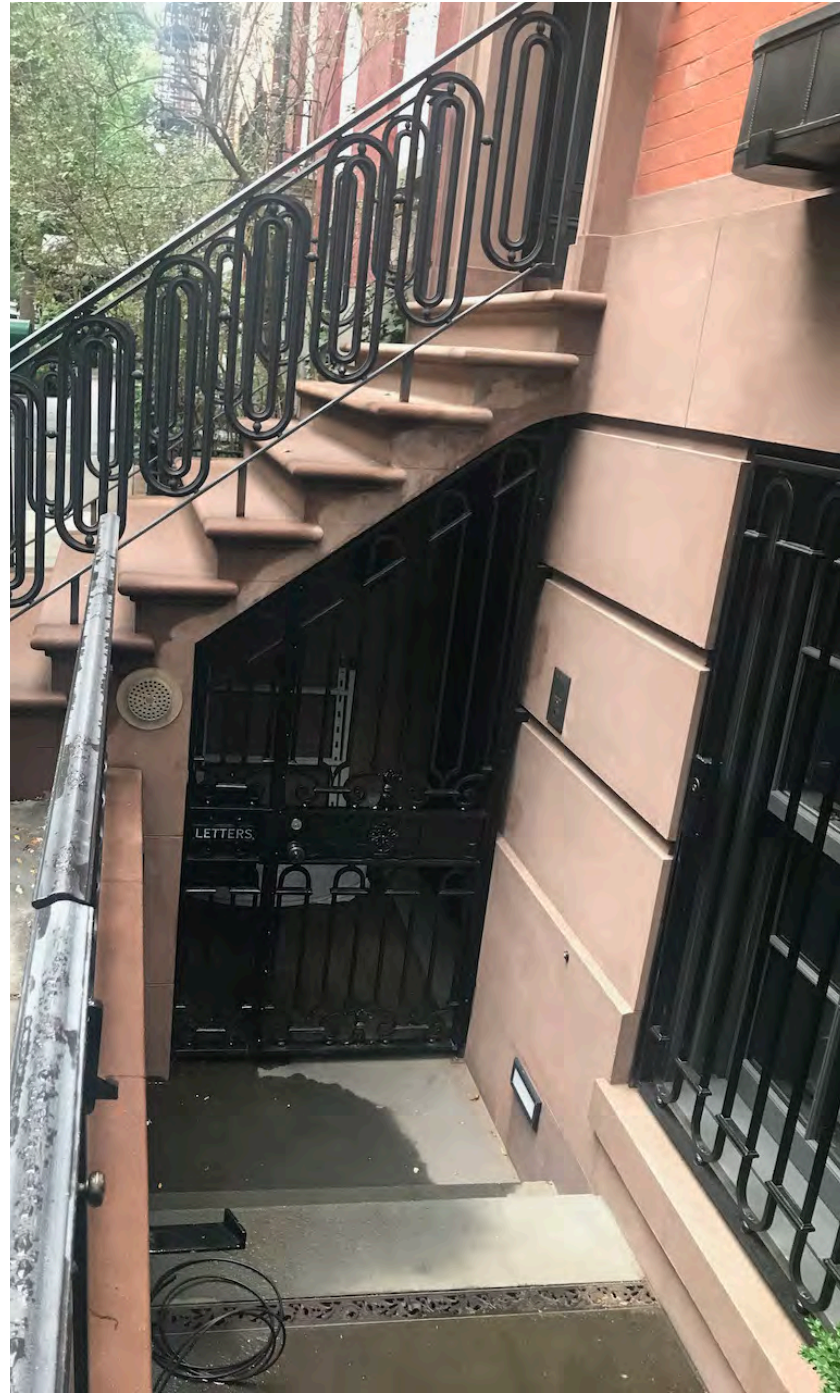
EXISTING BASEMENT GATE
