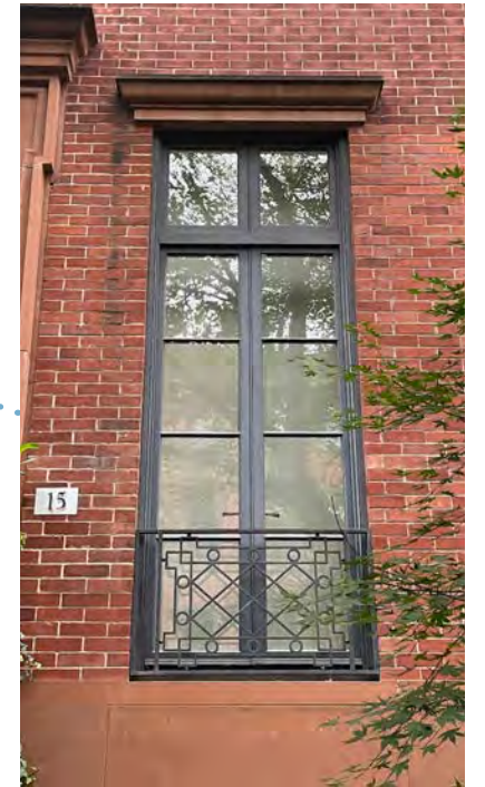
BROWNSTONE LINTELS AND SILLS TO MATCH EXISTING. DARK PAINTED IN-SWING FRENCH CASEMENT WINDOWS.
