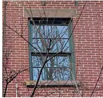
CAST STONE LINTELS AND SILLS TO MATCH EXISTING. DARK PAINTED DOUBLE HUNG WINDOWS.
