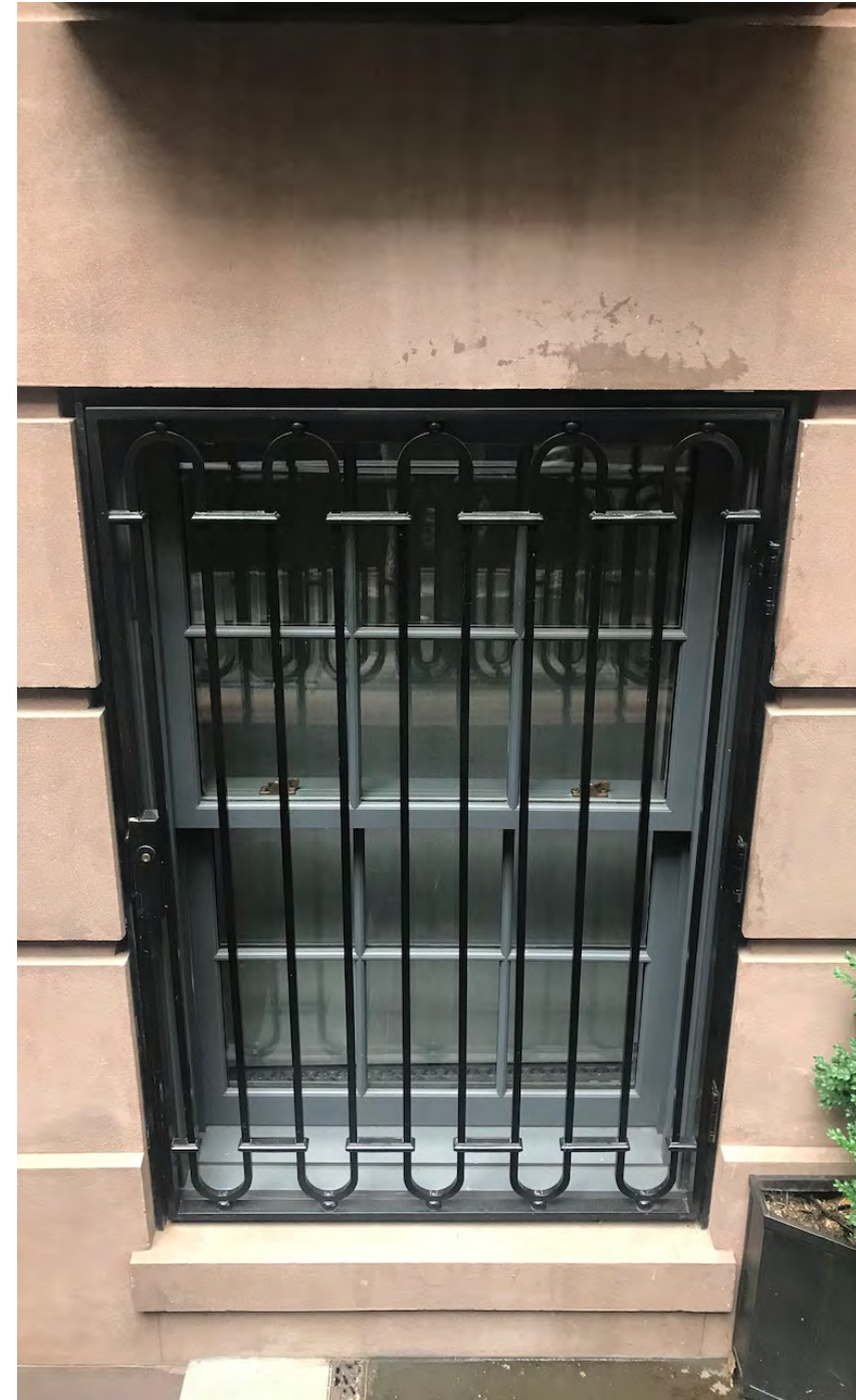
EXISTING WINDOW BARS
