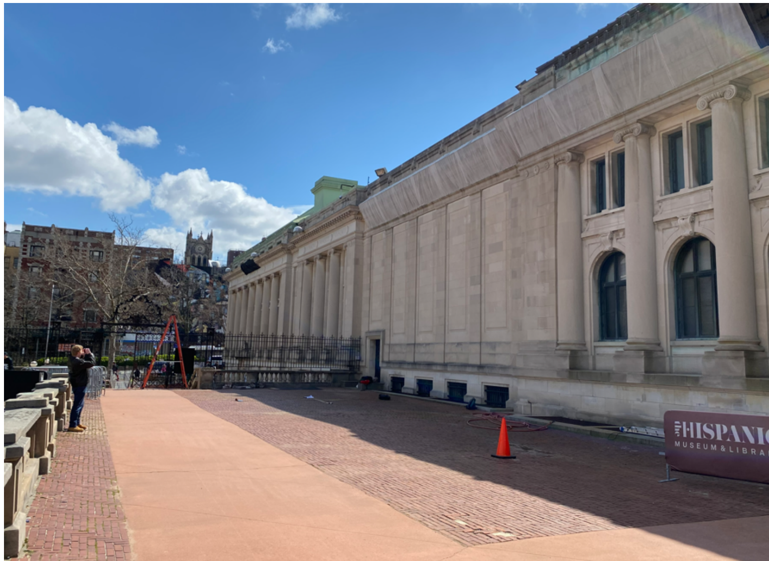
1 - View of Upper Terrace looking southeast
