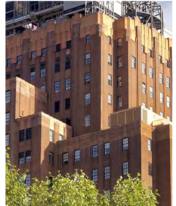
CROWN OF EXISTING BUILDING
