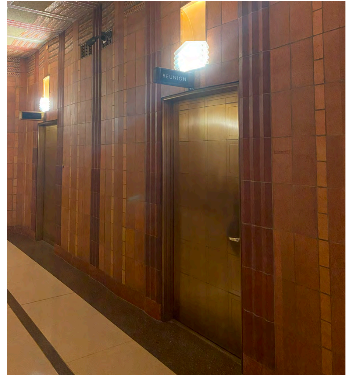
DETAIL VIEW OF DOORS AT SOUTH LOBBY WALL
