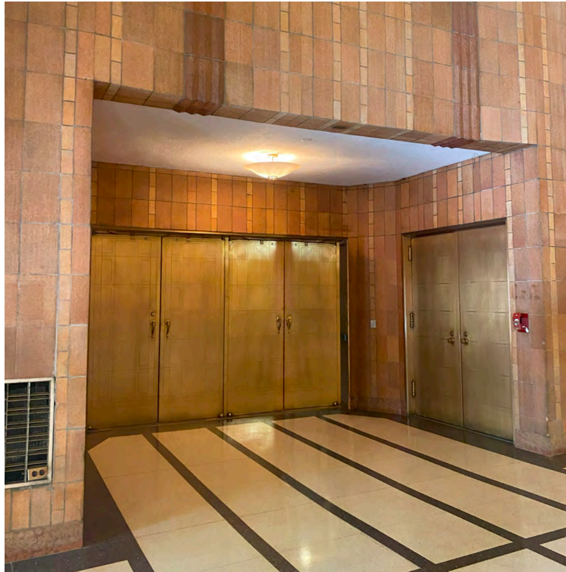
EXISTING DOUBLE DOORS AT FORMER AUDITORIUM
