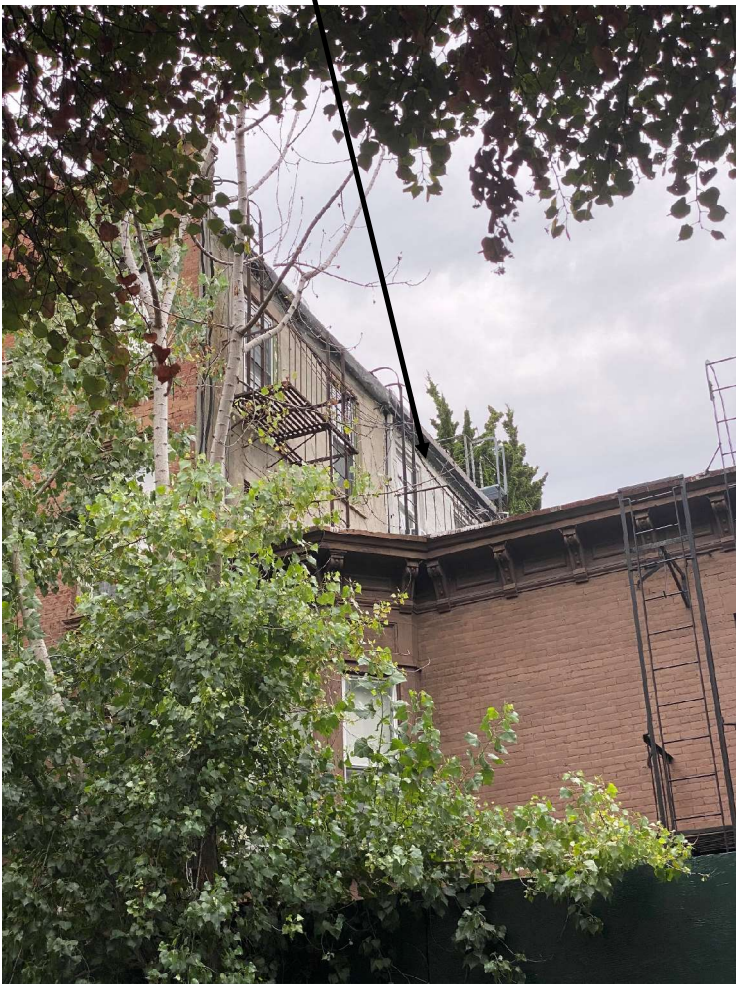
Existing Conditions from Cross Street Baltic Street
