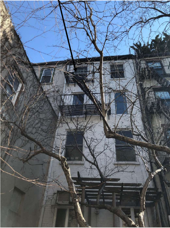
4th Floor Fire escape
