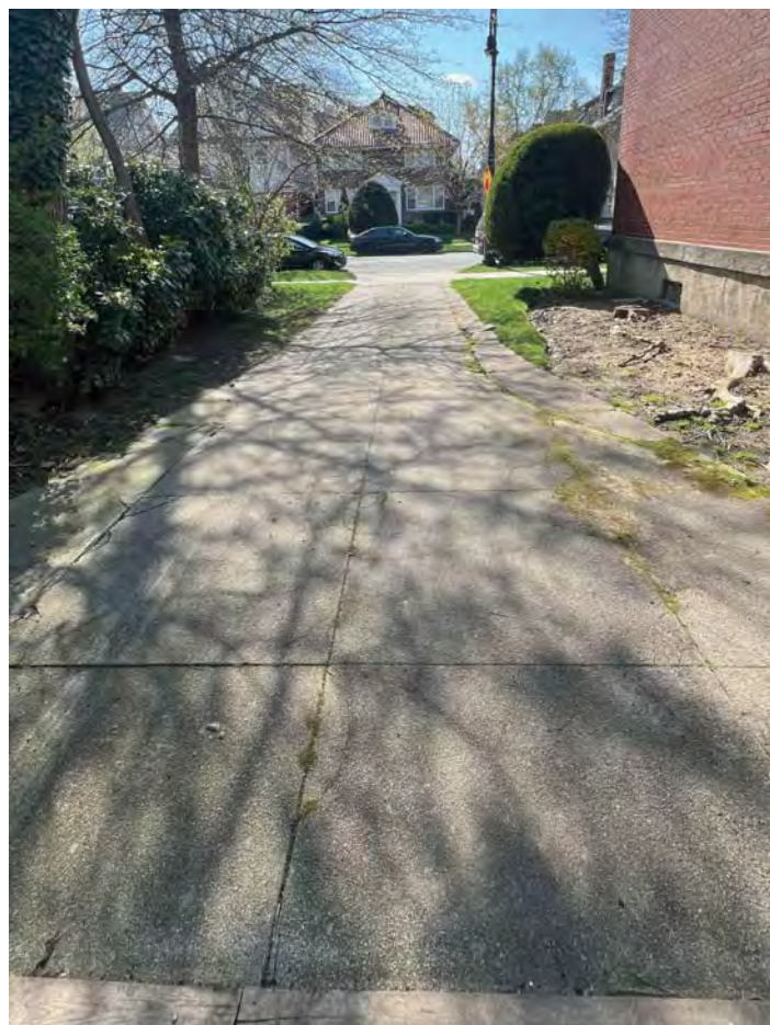
DRIVEWAY VIEW FROM GARAGE
