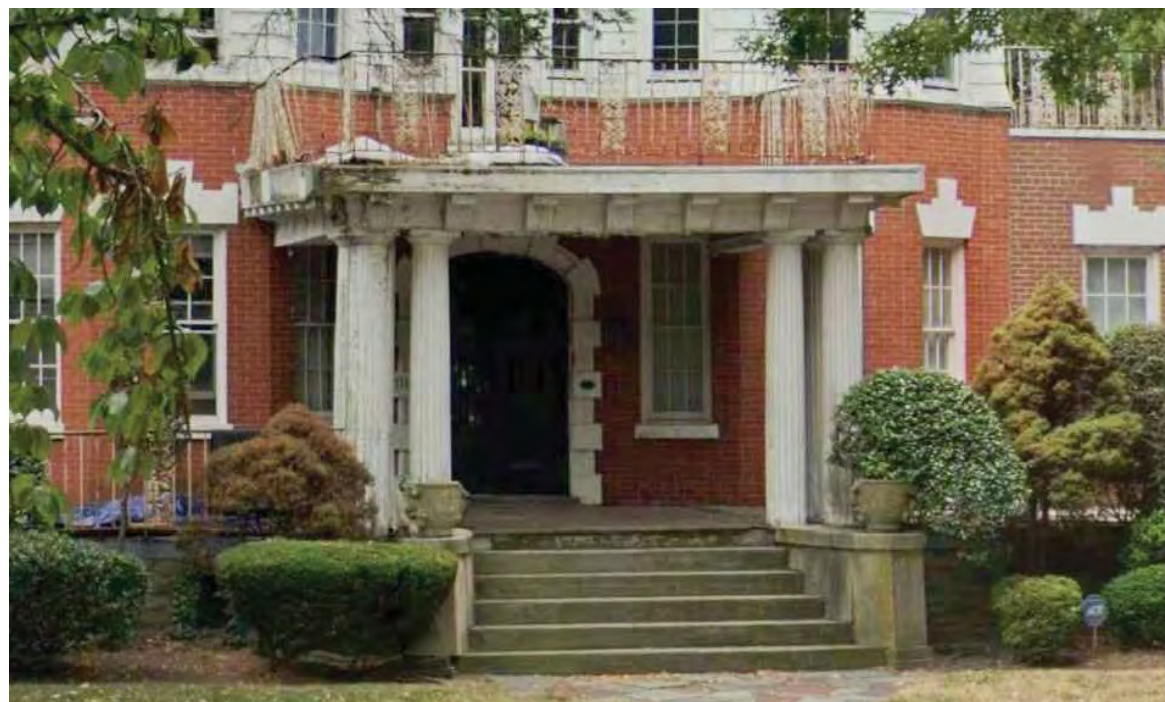
EXISTING PORCH, FRONT VIEW
