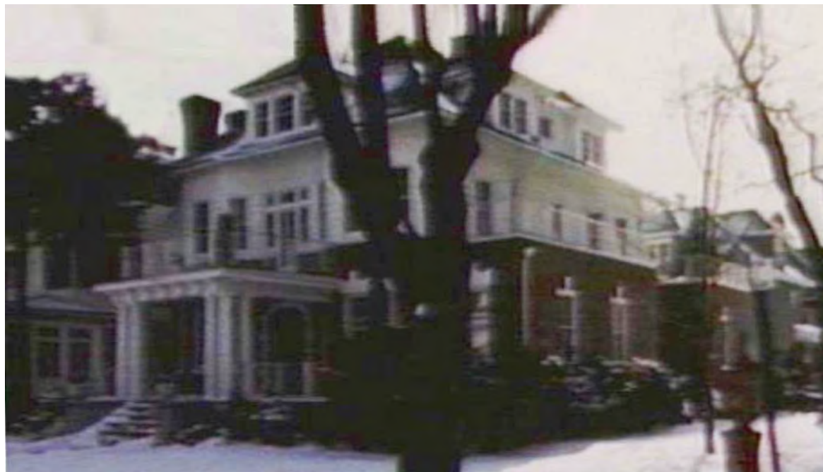
HOUSE ADDITION SHOWN IN TAX PHOTO, 1980S
