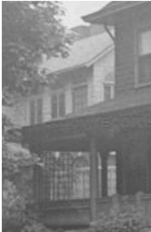
ORIGINAL HOUSE SOUTH WEST CORNER
