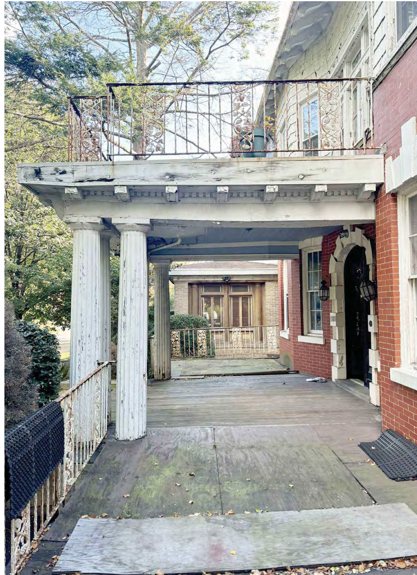
EXISTING PORCH, SIDE VIEW
