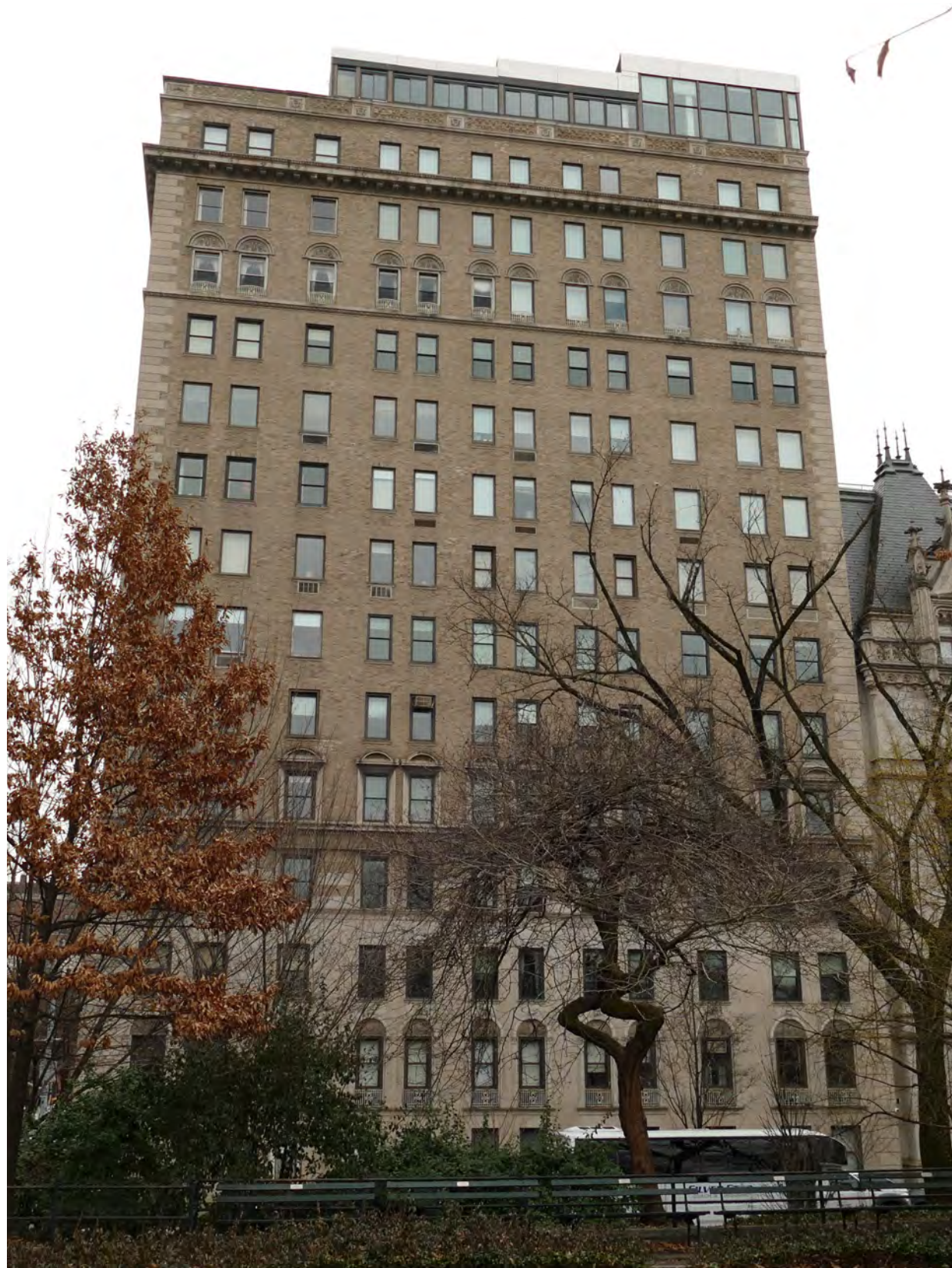
1115 Fifth Ave - primary facade.
