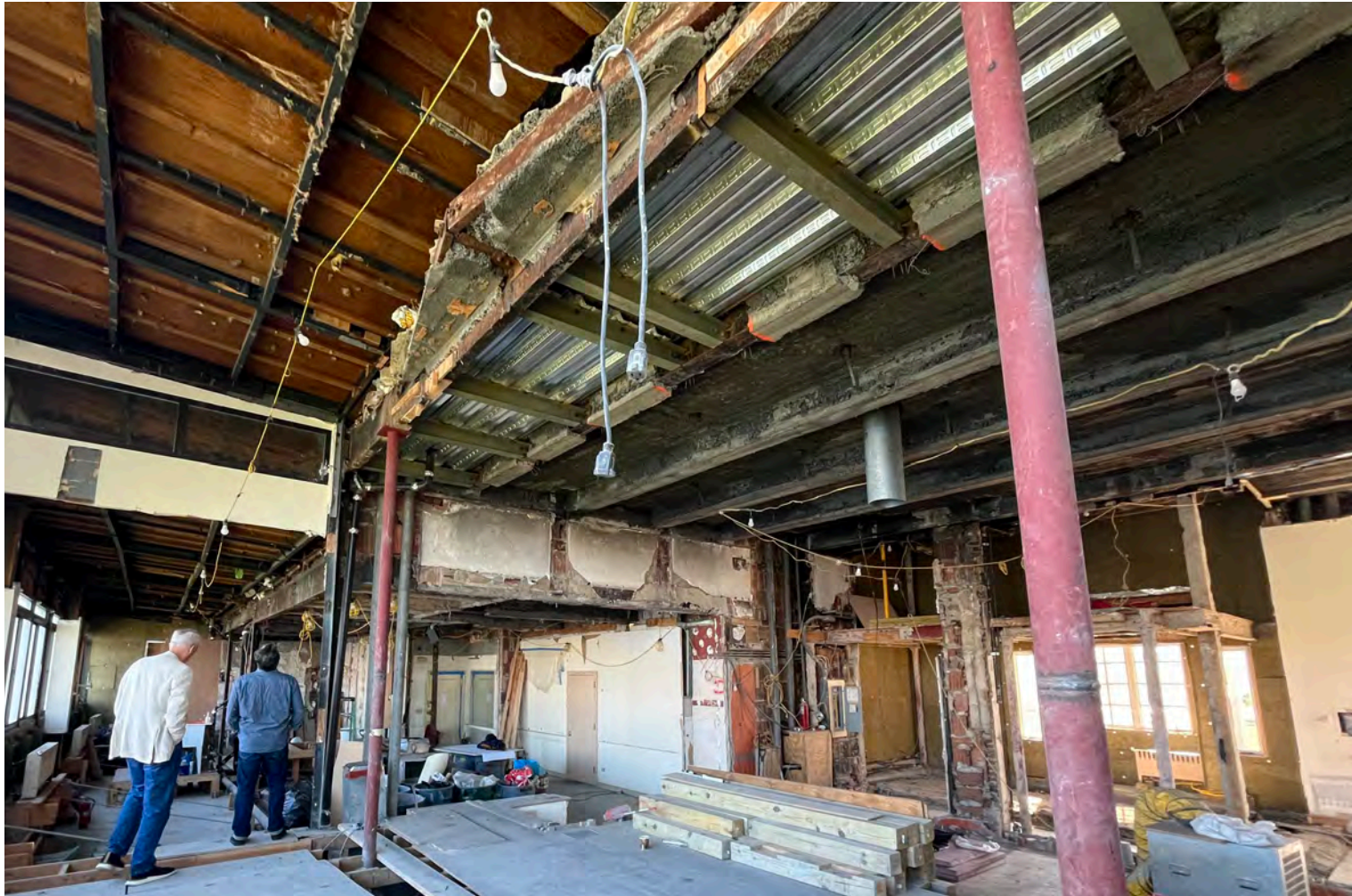
INTERIOR ROOF STRUCTURE SHOWING HISTORIC MULTI-LEVEL CONDITIONS.
