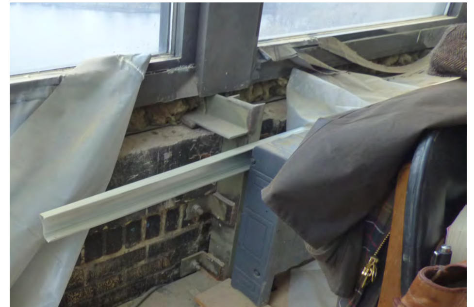
Detail of parapet.
