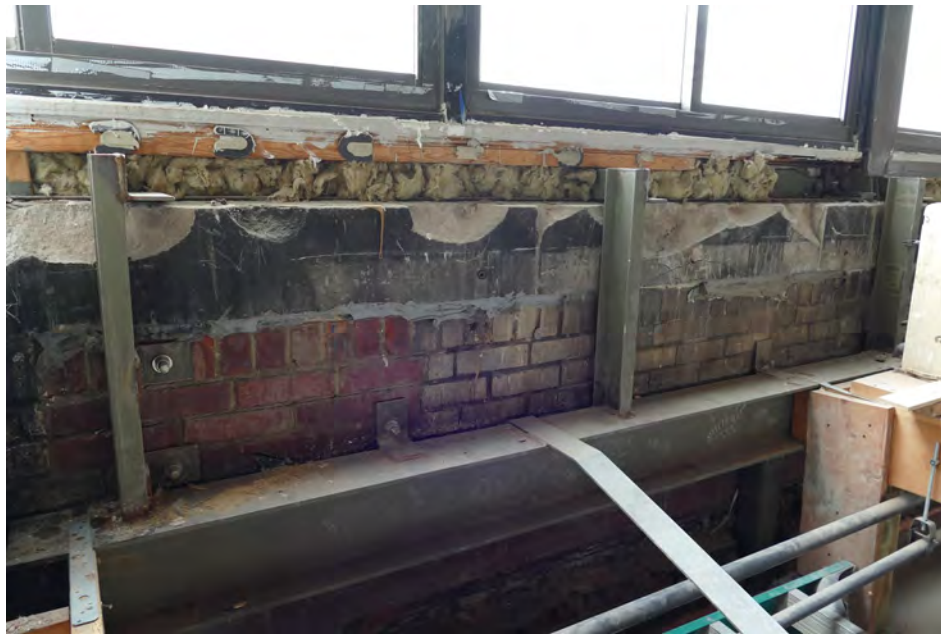
Detail of structure of unknown vintage mounted to parapet.
