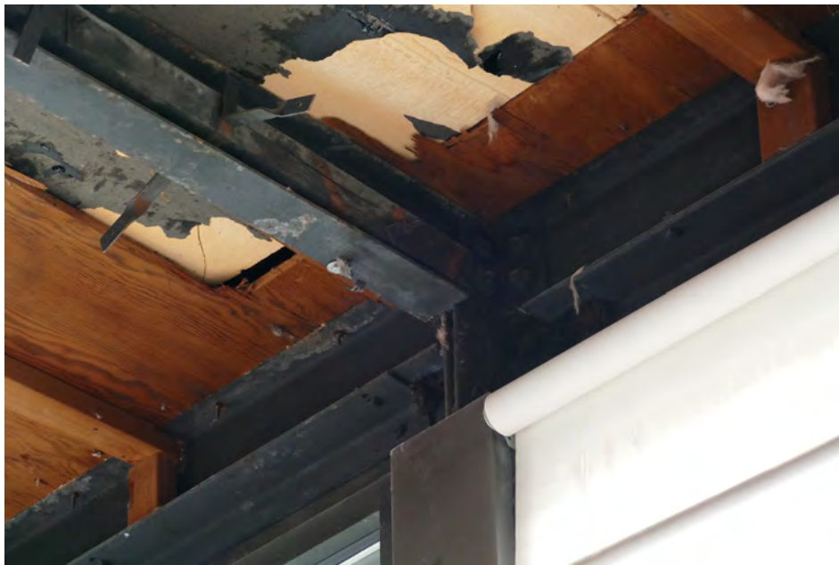
Detail of structure above tall windows.
