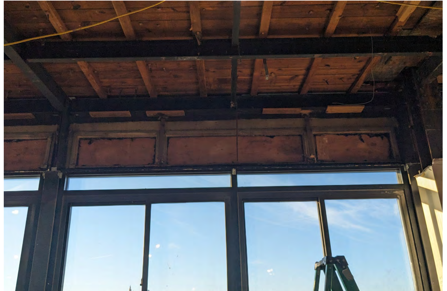
HISTORIC WINDOWS VISIBLE FOLLOWING INTERIOR DEMOLITION.
