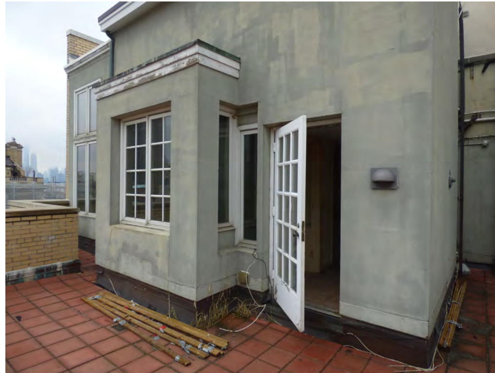
2. East elevation, looking southwest
