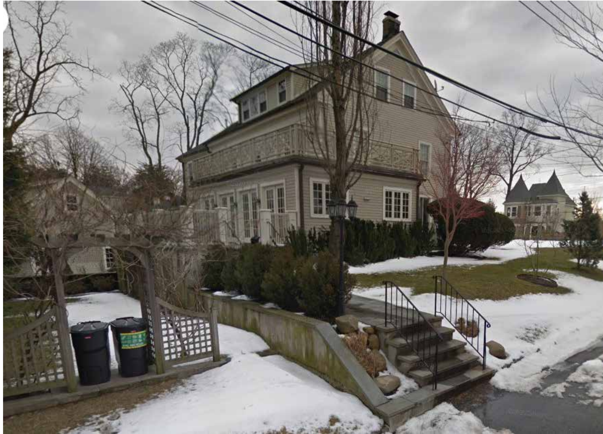
REAR FACADE - PRIOR TO INSTALLATION OF SHED AND FENCE
