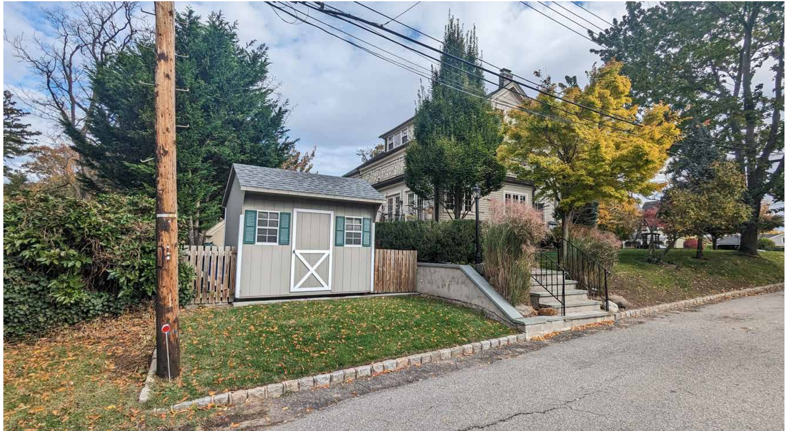
REAR FACADE - SOUTH ELEVATION
