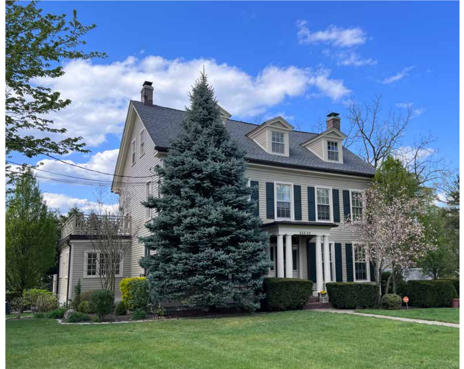
EXISTING SOUTH-WEST VIEW
