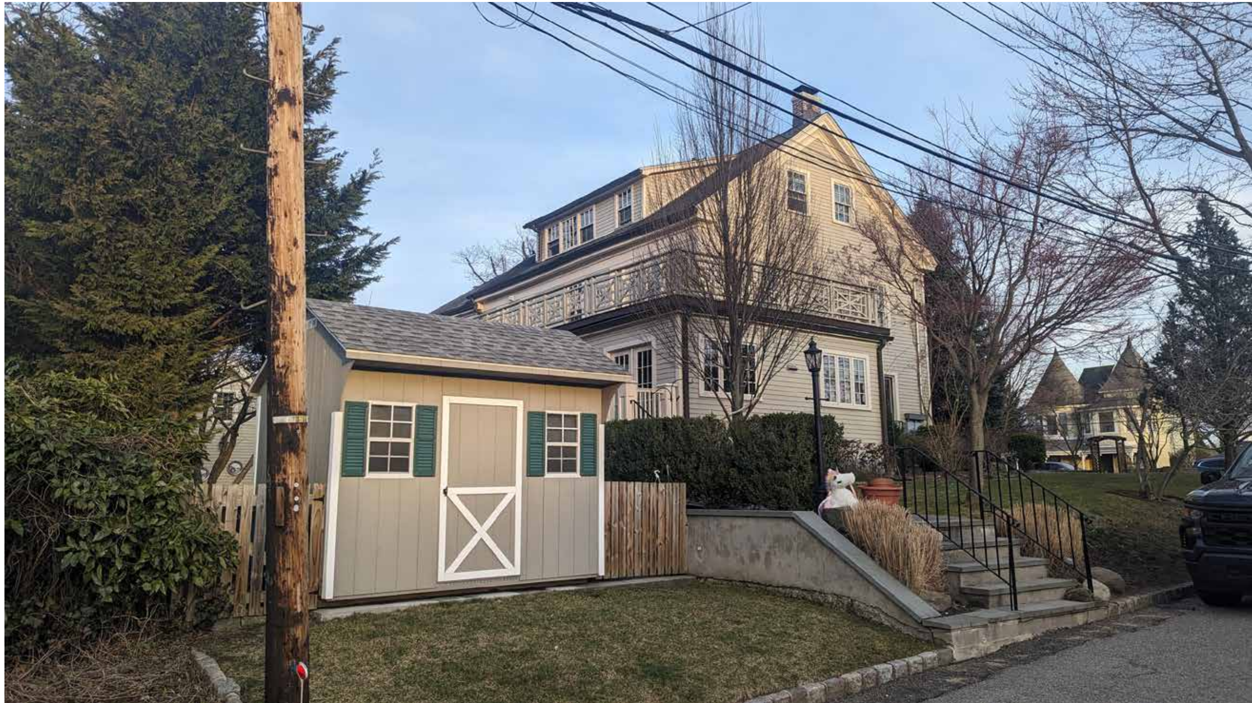
REAR FACADE - SOUTH
