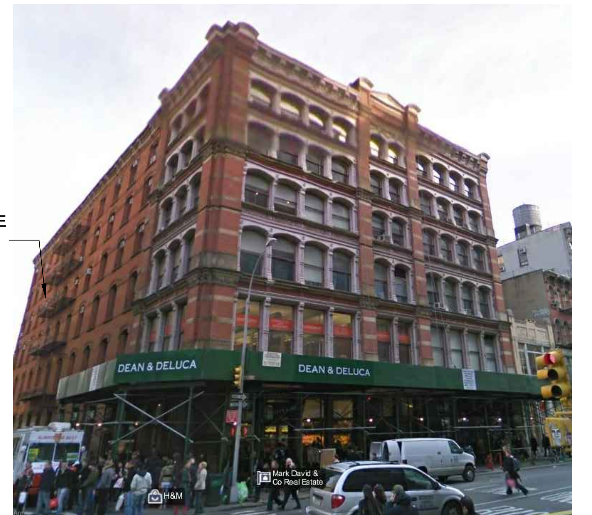
C 560 BROADWAY BEFORE REMOVAL
