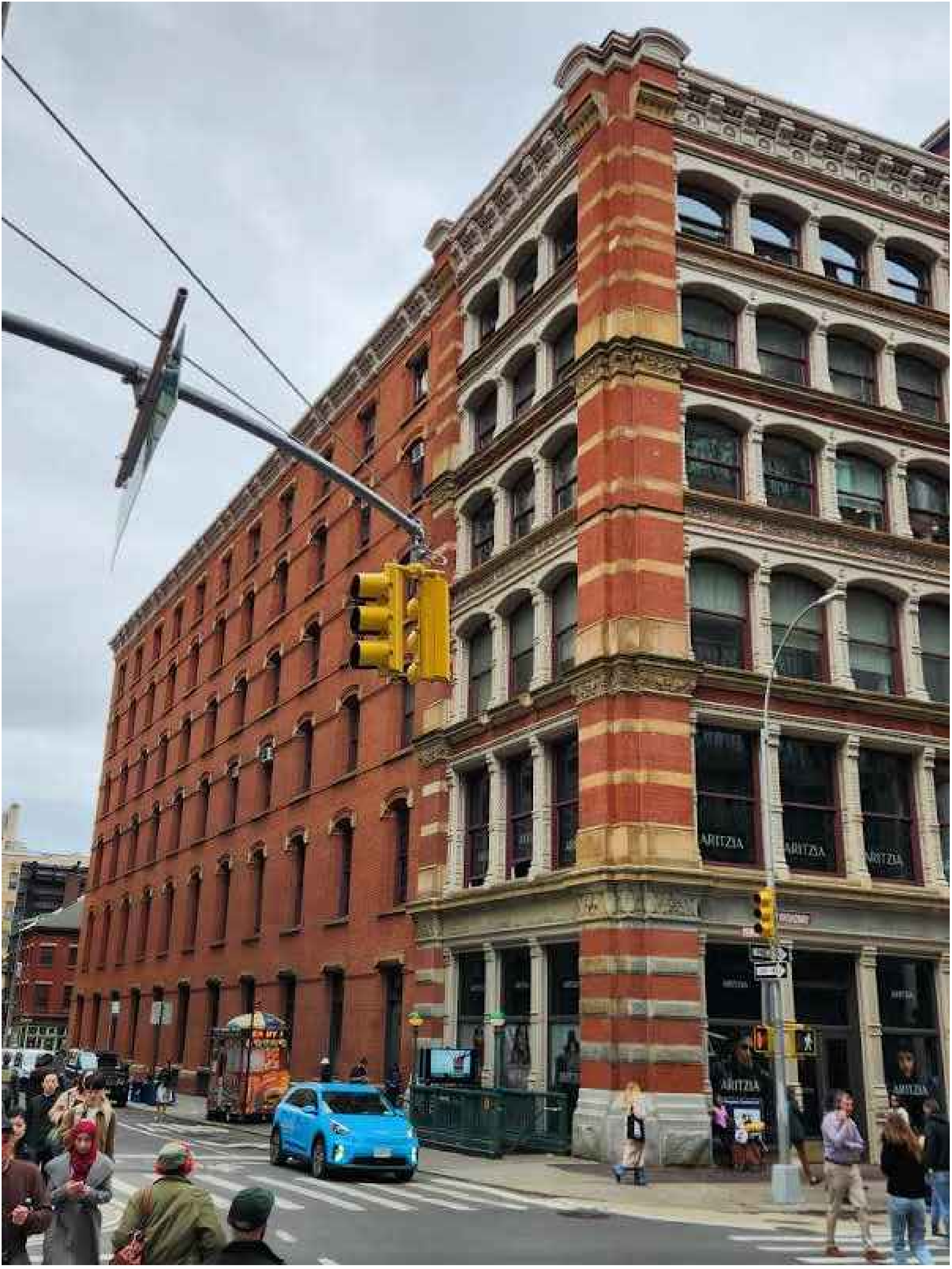
© 560 BROADWAY AFTER REMOVAL
