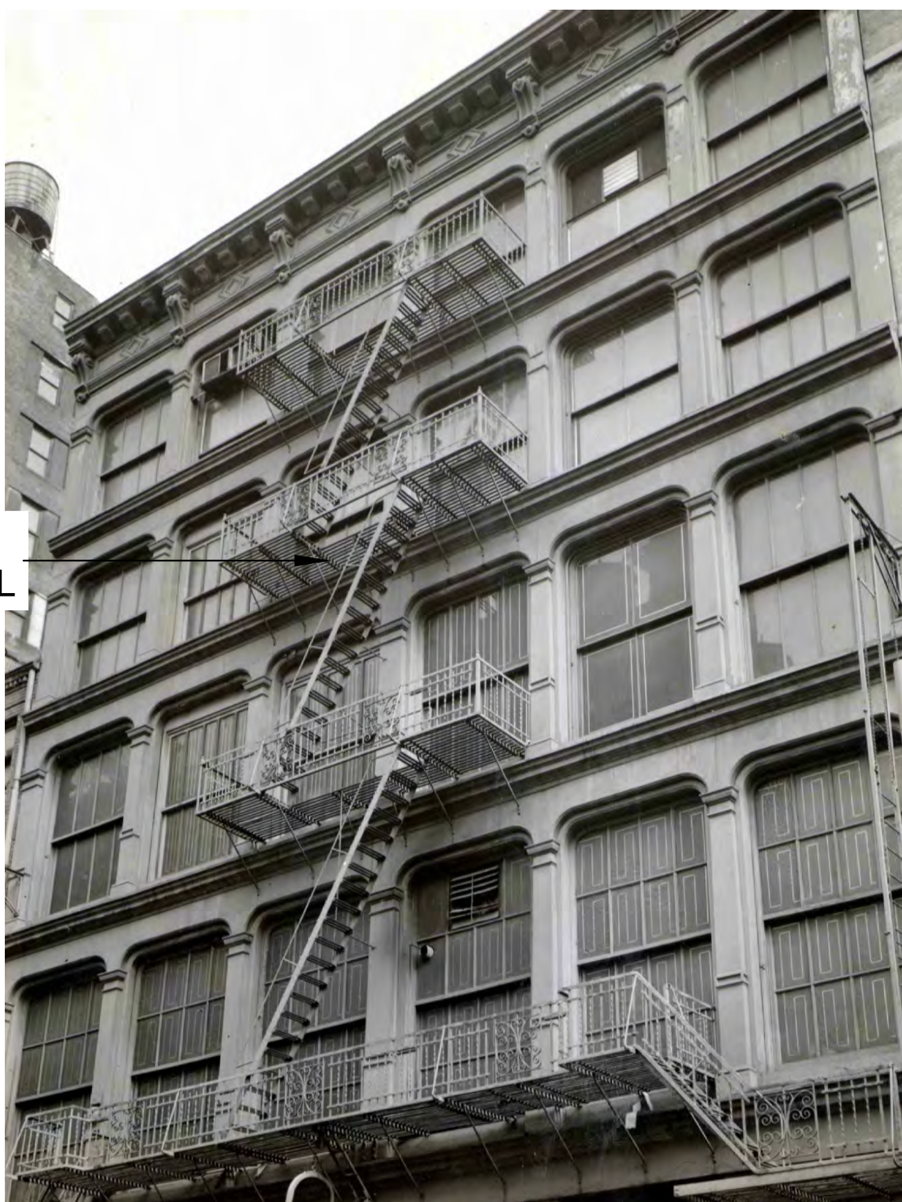
A 50-52 MERCER STREET BEFORE REMOVAL
