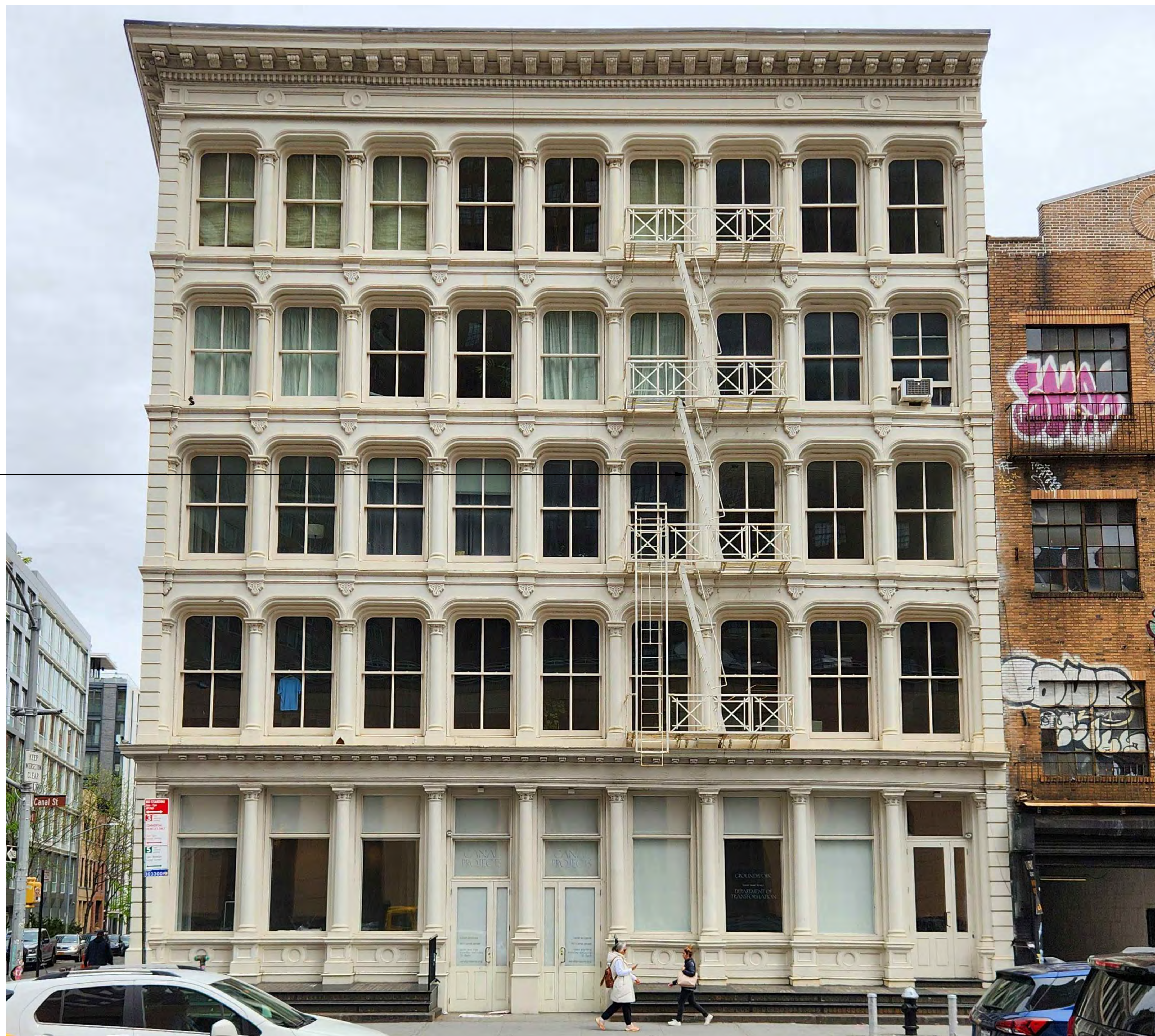
B 351 CANAL STREET BEFORE REMOVAL
