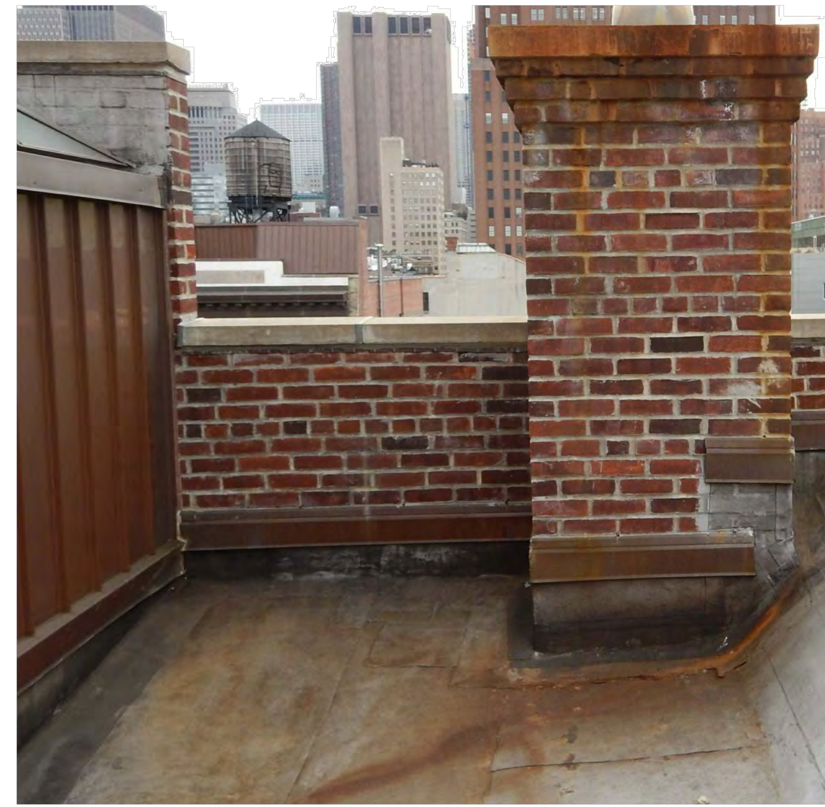
7 ROOF LEVEL PARAPET, LOOKING WEST
