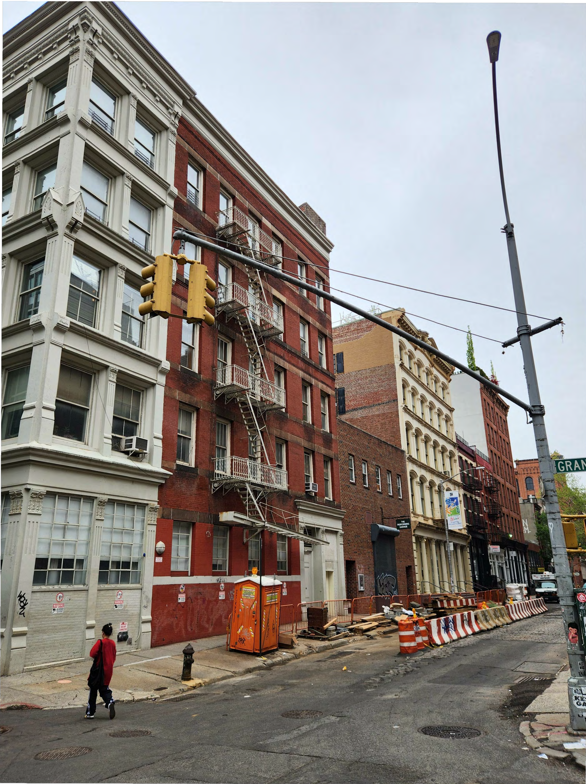
VIEW A: ALONG WOOSTER STREET WEST SIDE FACING NORTH
