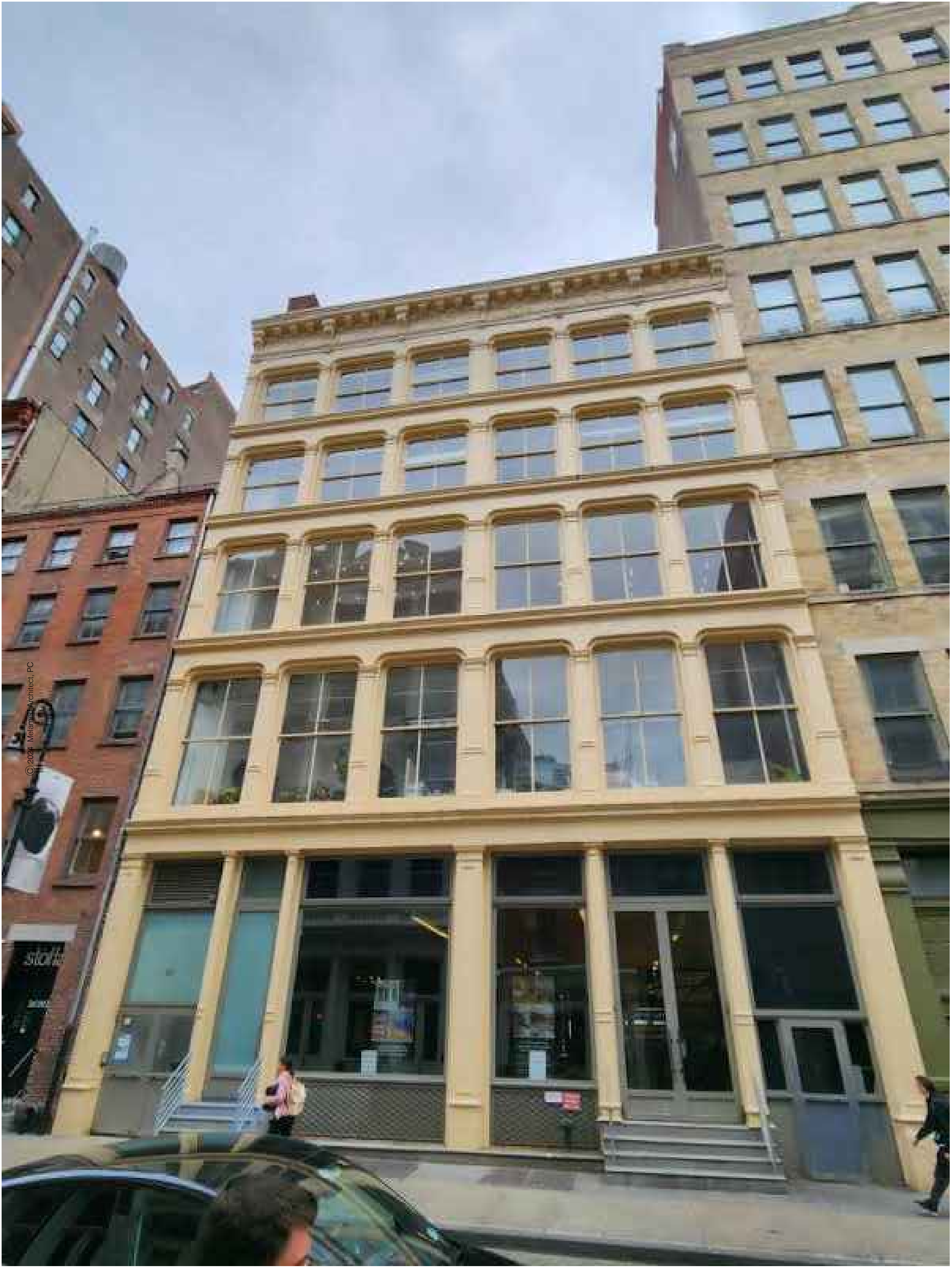
A 50-52 MERCER STREET AFTER REMOVAL
