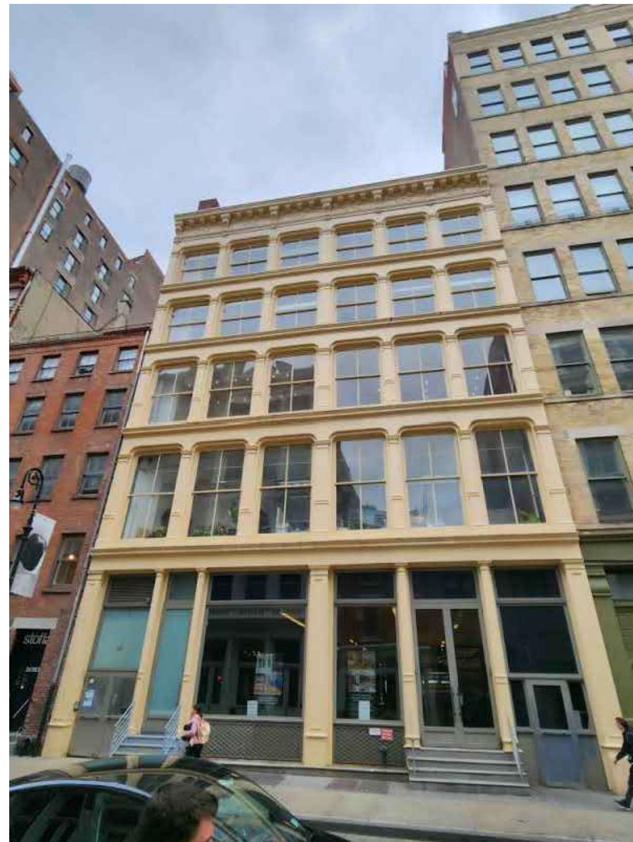
A 50-52 MERCER STREET AFTER REMOVAL
