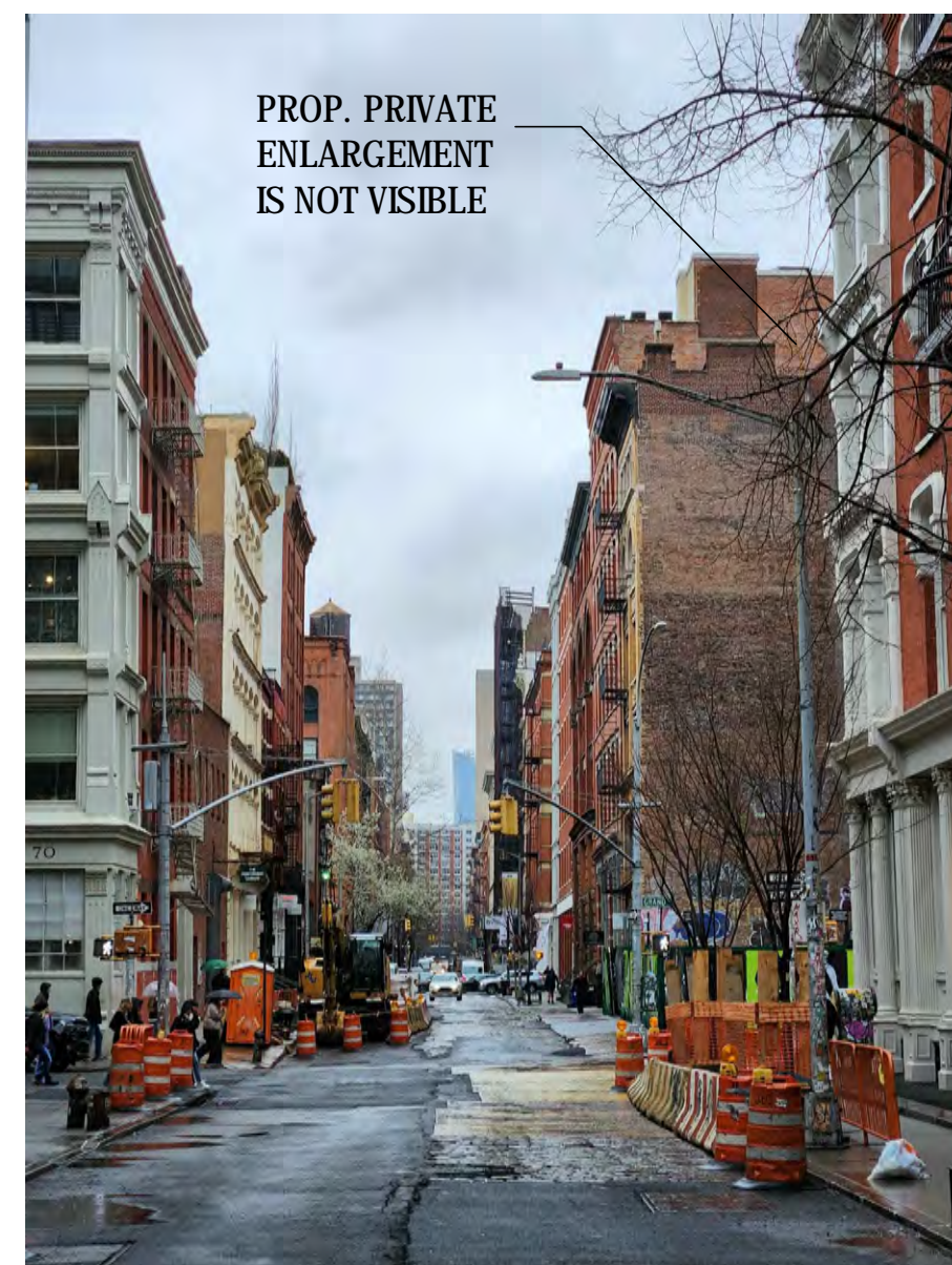
VIEW 4: ALONG WOOSTER STREET PROPOSED ADDITION IS NOT VISIBLE
