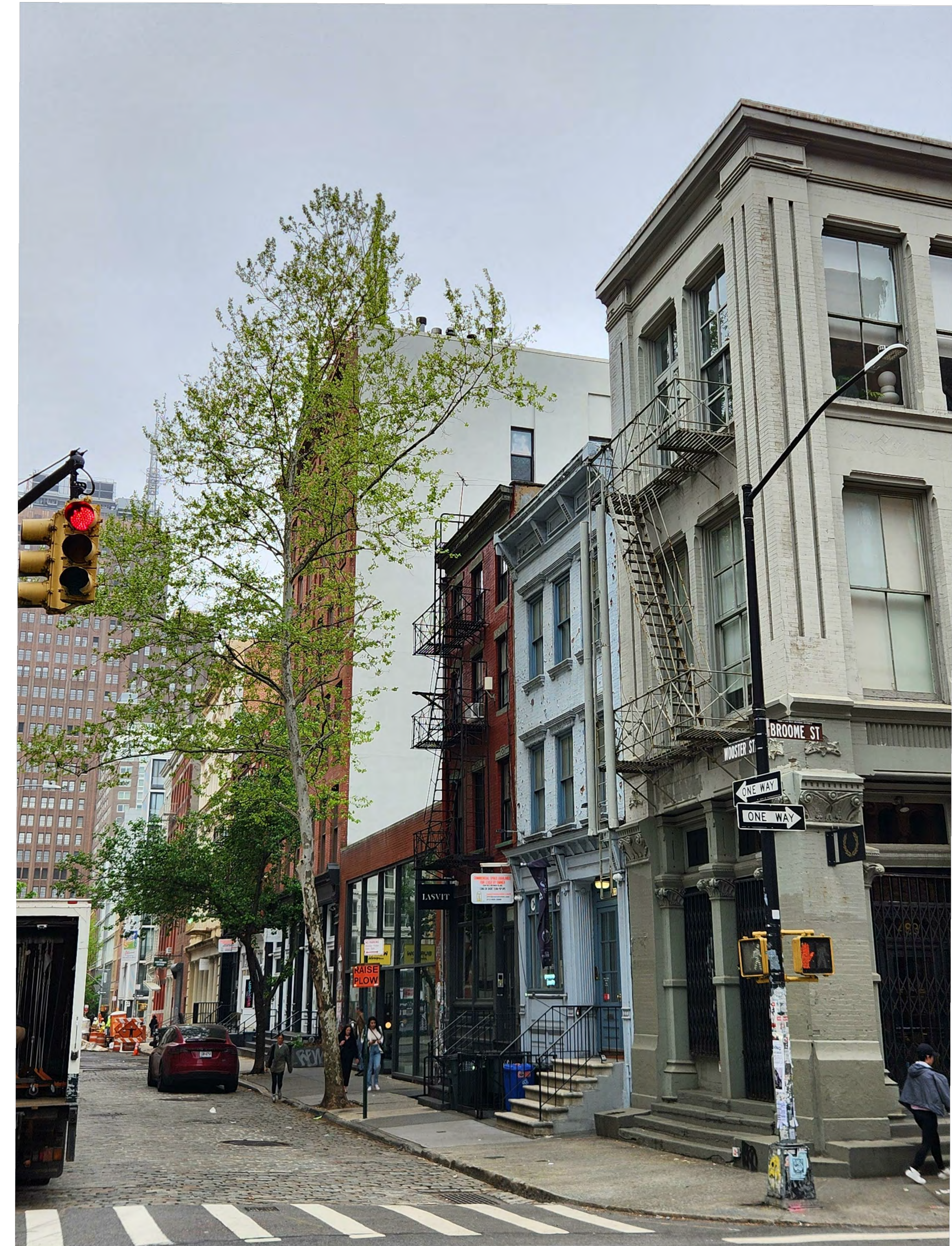
VIEW B: ALONG WOOSTER STREET WEST SIDE FACING SOUTH
