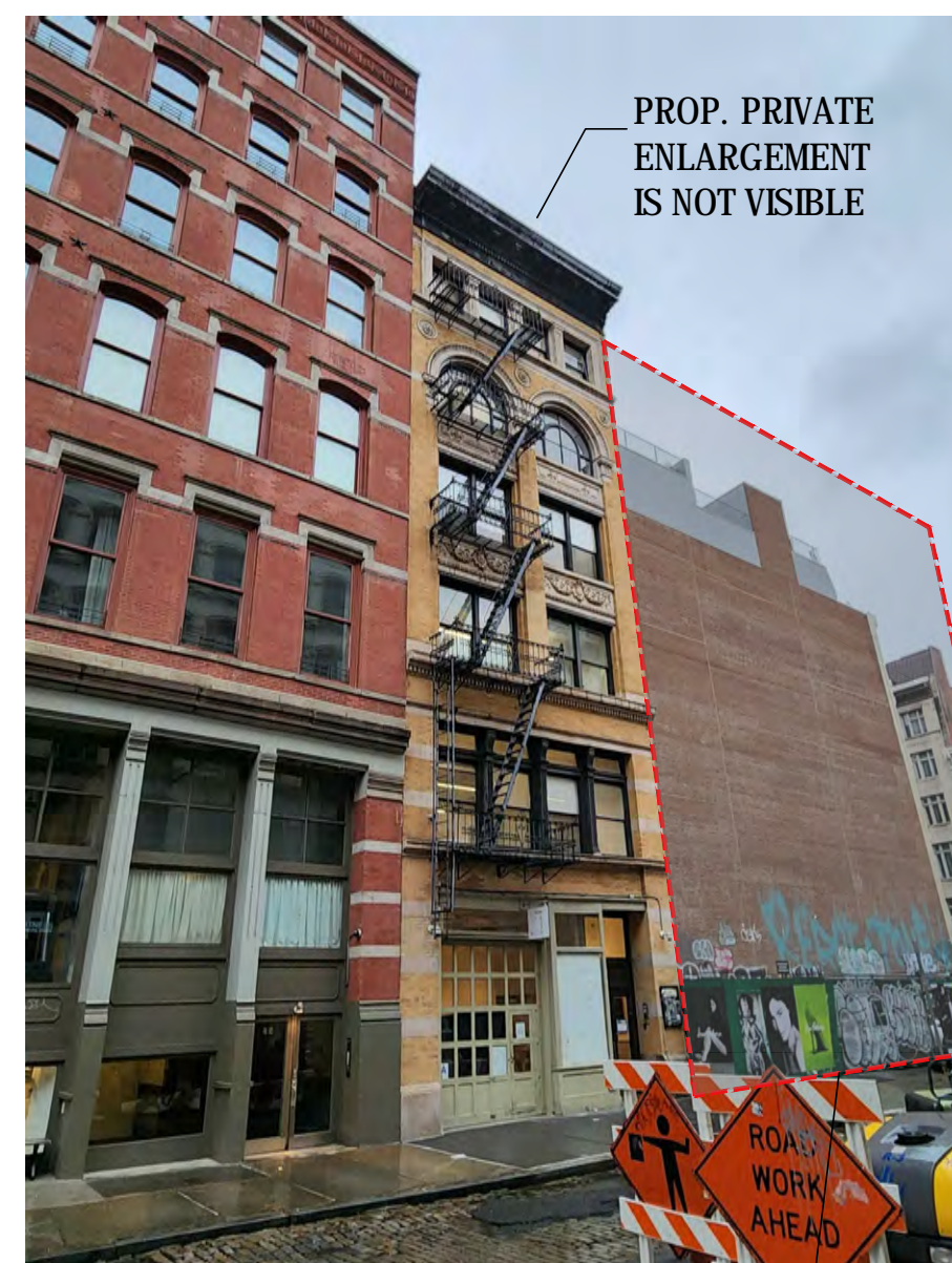
VIEW 8: ALONG WOOSTER STREET PROPOSED ADDITION IS NOT VISIBLE
