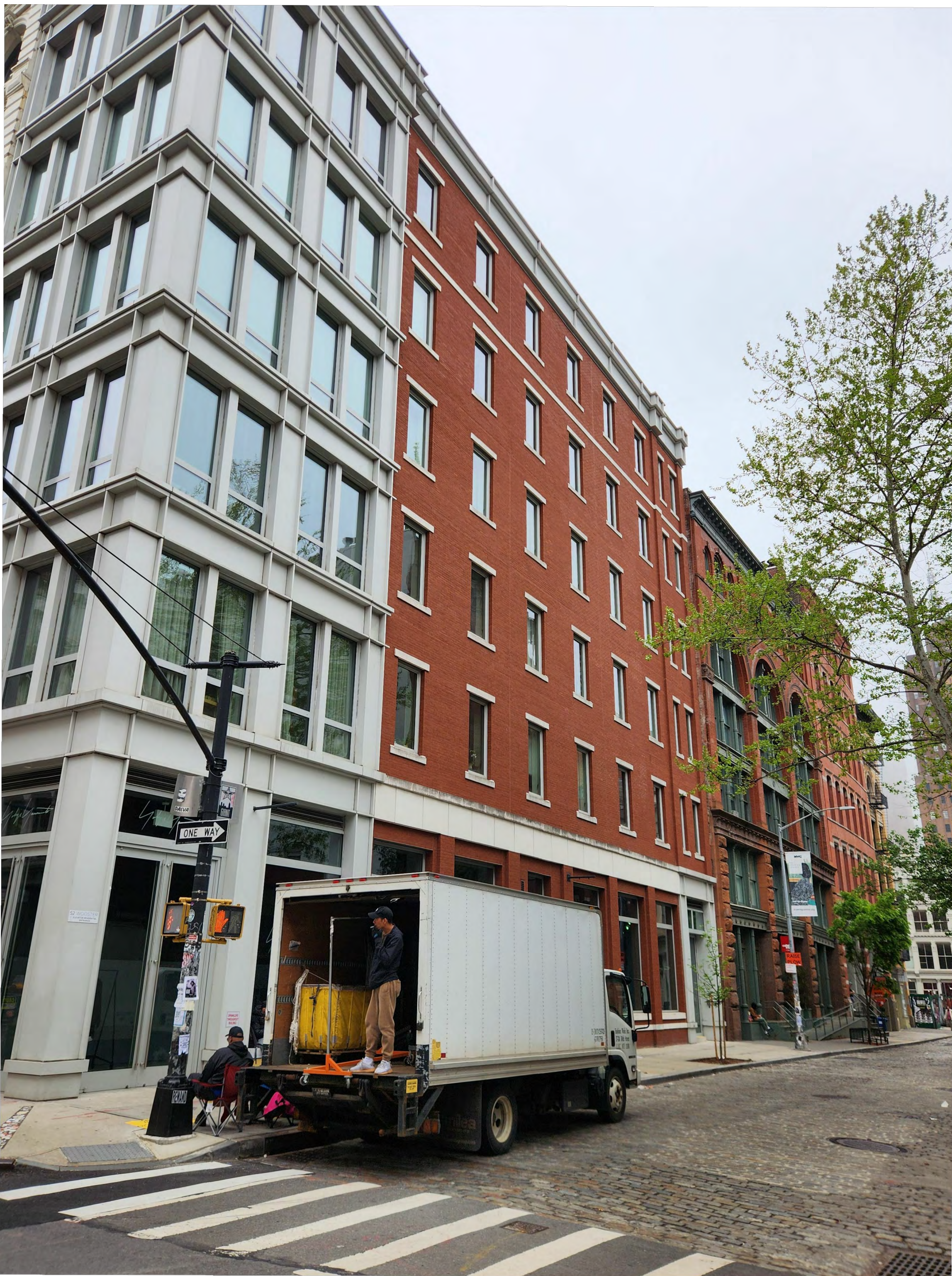
VIEW C: ALONG WOOSTER STREET EAST SIDE FACING SOUTH
