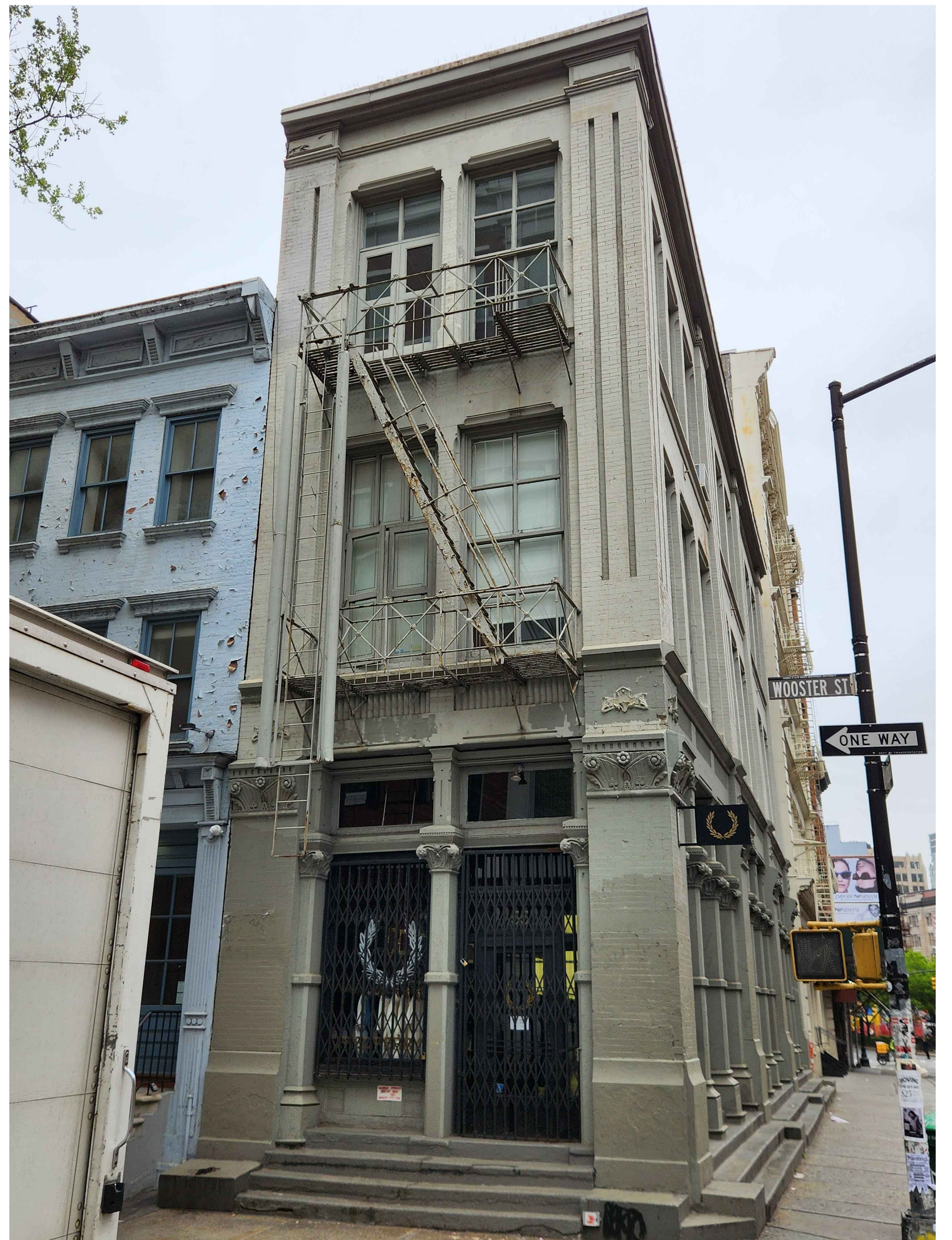
VIEW 2: 483 BROOME ST (SOUTHWEST CORNER - WOOSTER & BROOME)
