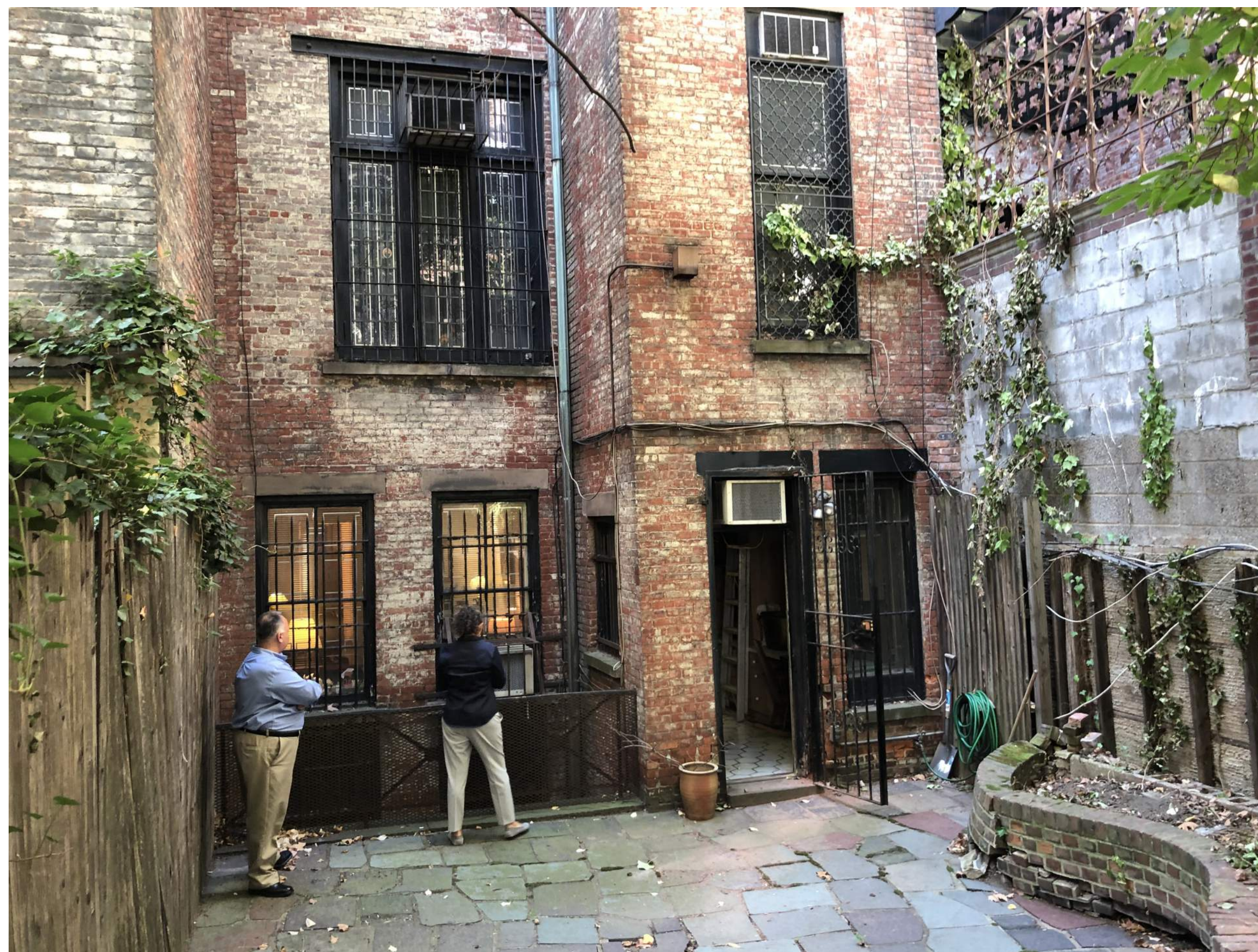
04 PHOTO FROM REAR YARD LOOKING SOUTH N.T.S.
