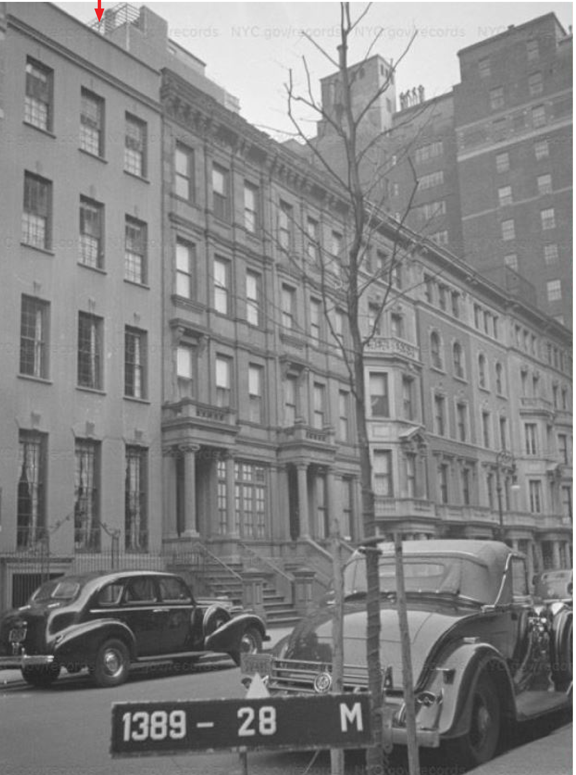
03 HISTORIC 1940 TAX PHOTO LOOKING NORTH N.T.S.
