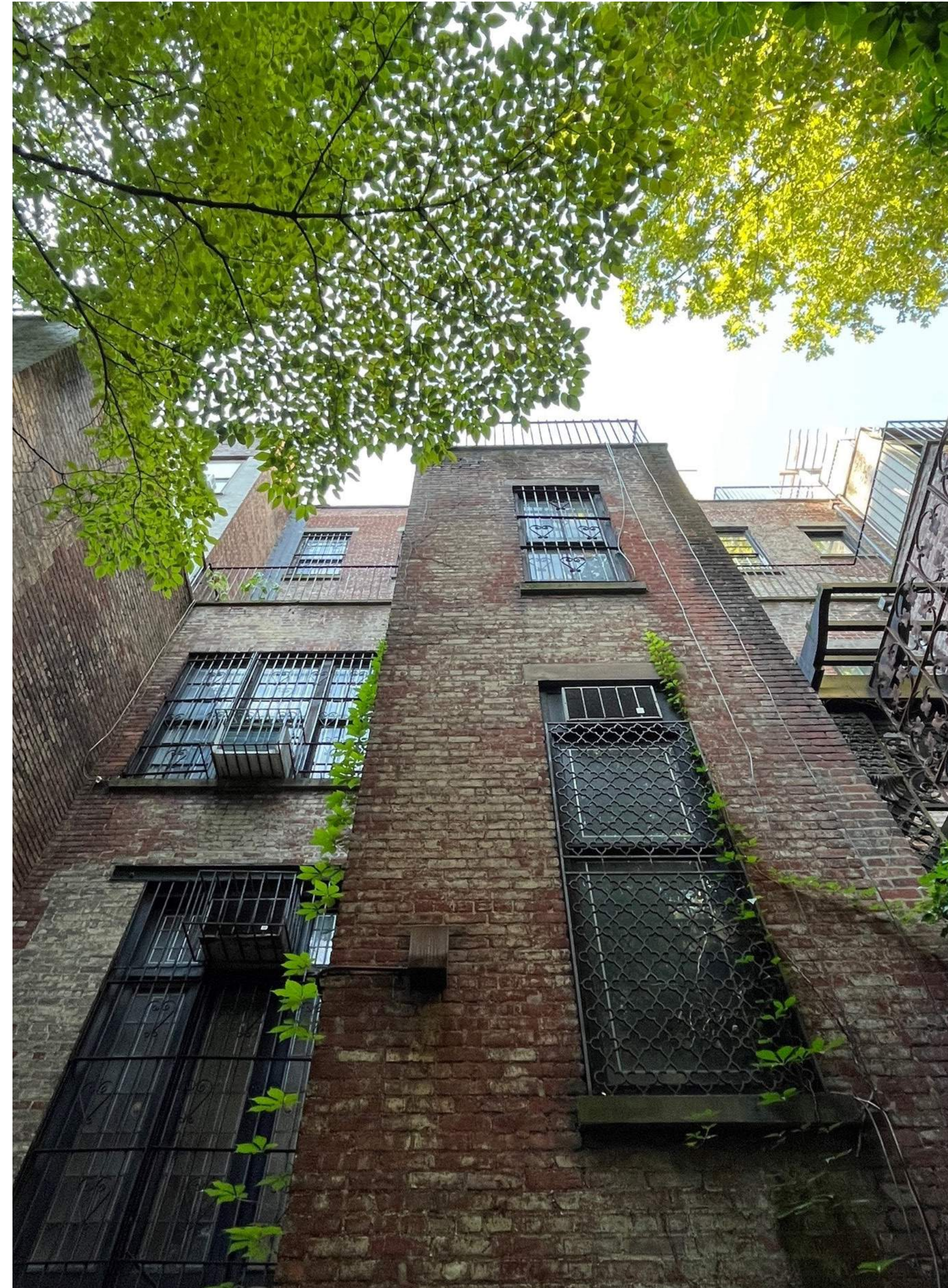
02 PHOTO FROM REAR YARD LOOKING SOUTH N.T.S.
