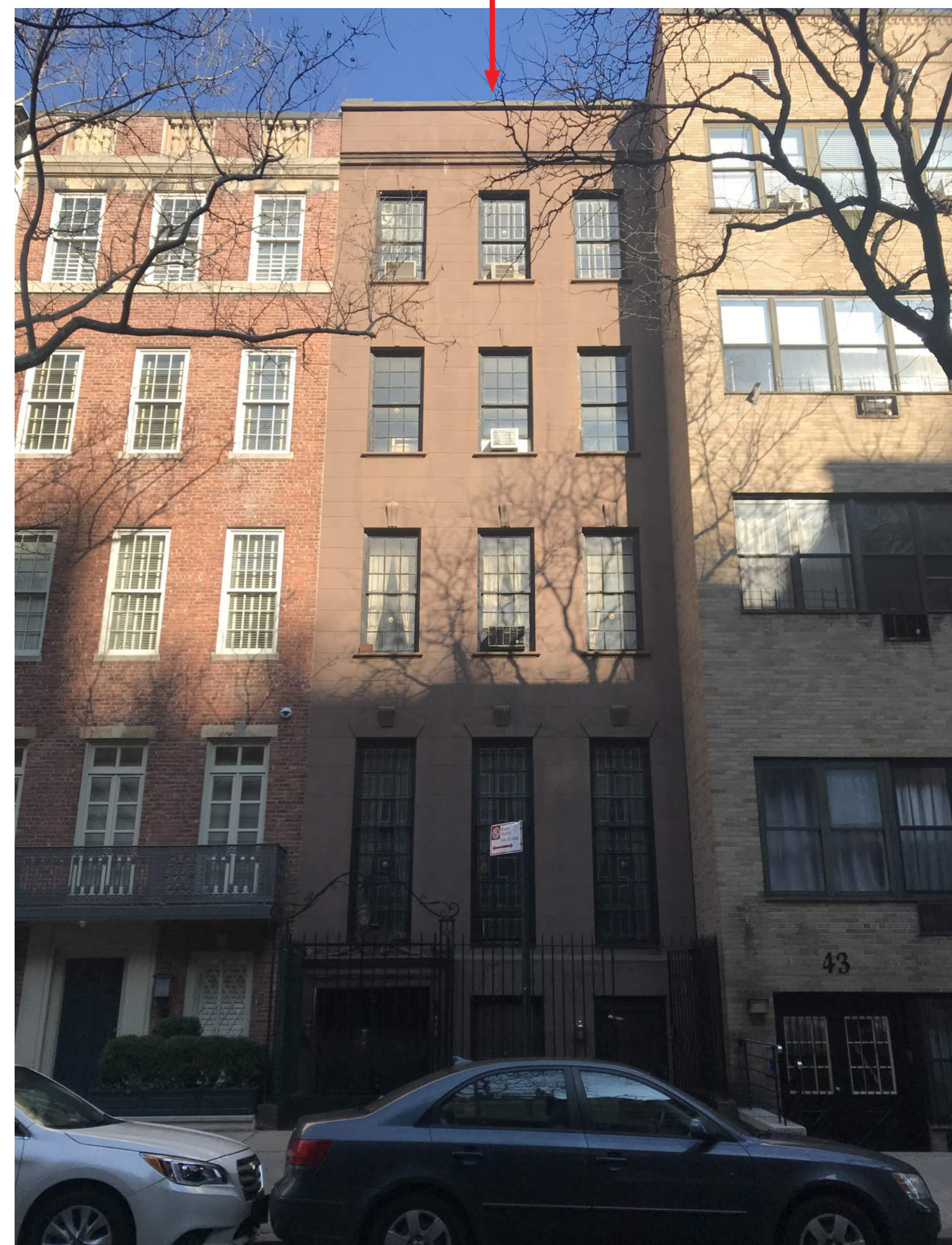
02 OVERALL VIEW OF BUILDING FRONT FACADE N.T.S.
