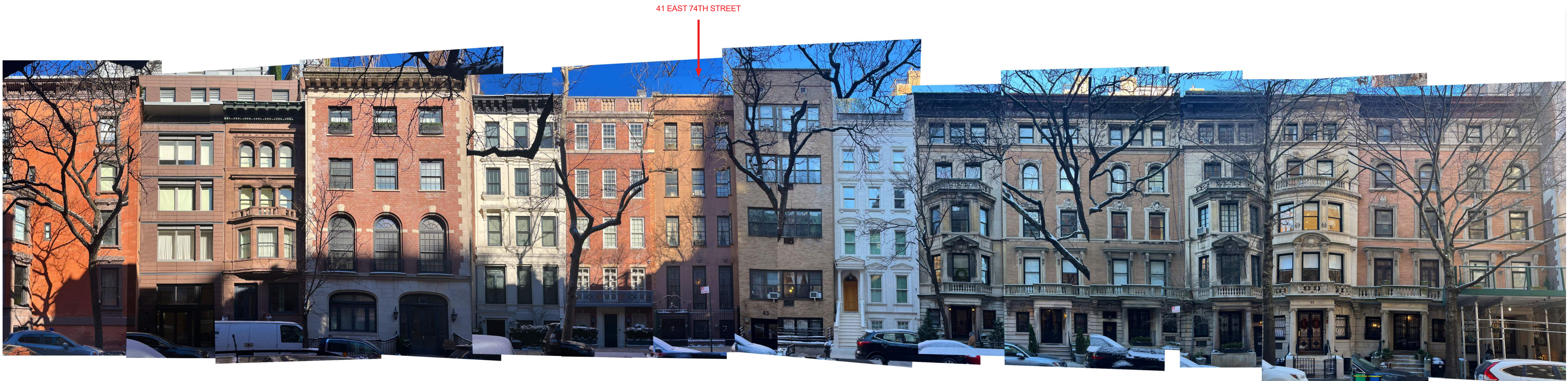
01 EXISTING PANORAMIC VIEW - NORTH SIDE OF BLOCK N.T.S.
