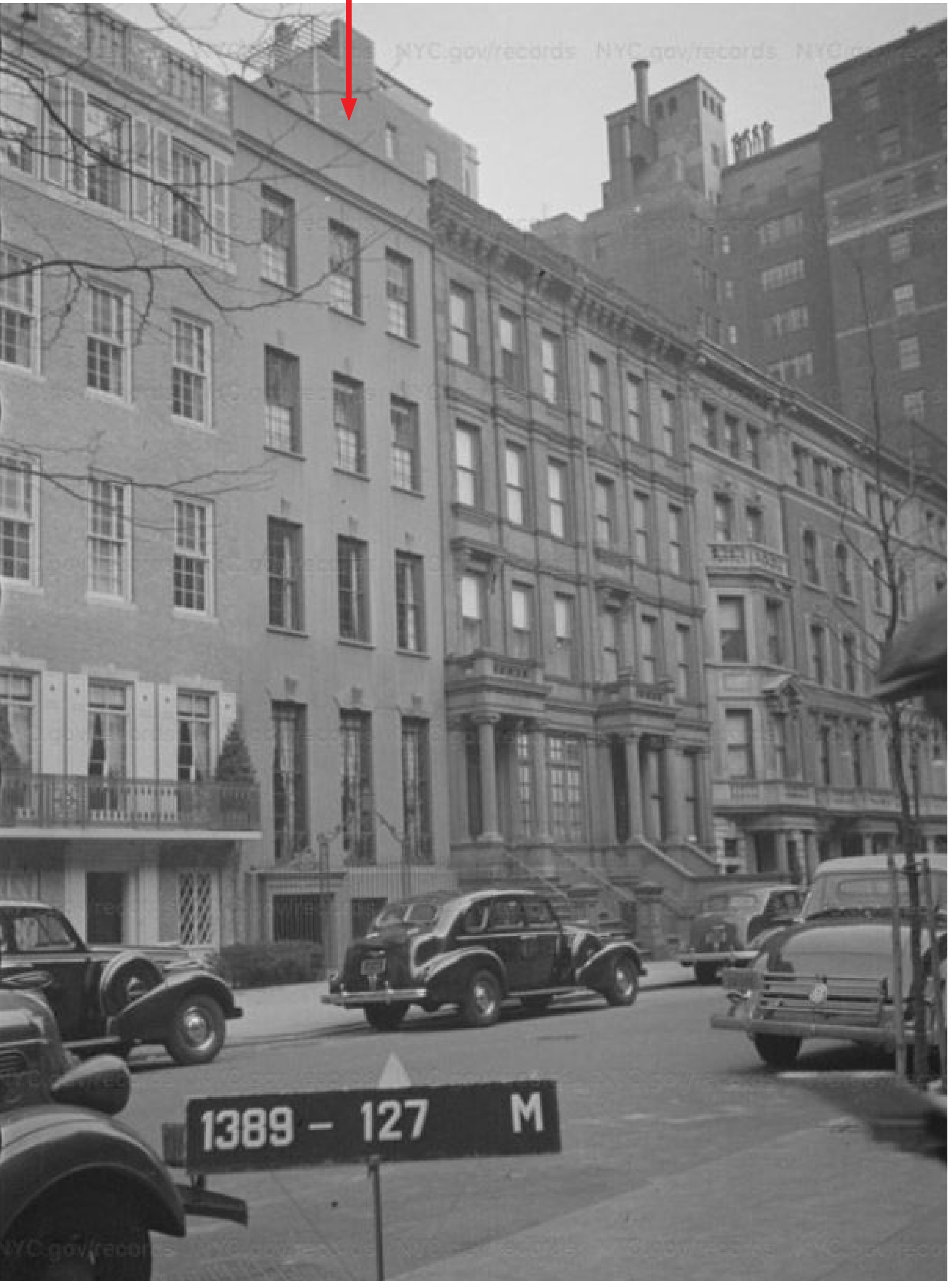
02 HISTORIC 1940 TAX PHOTO LOOKING NORTH N.T.S.
