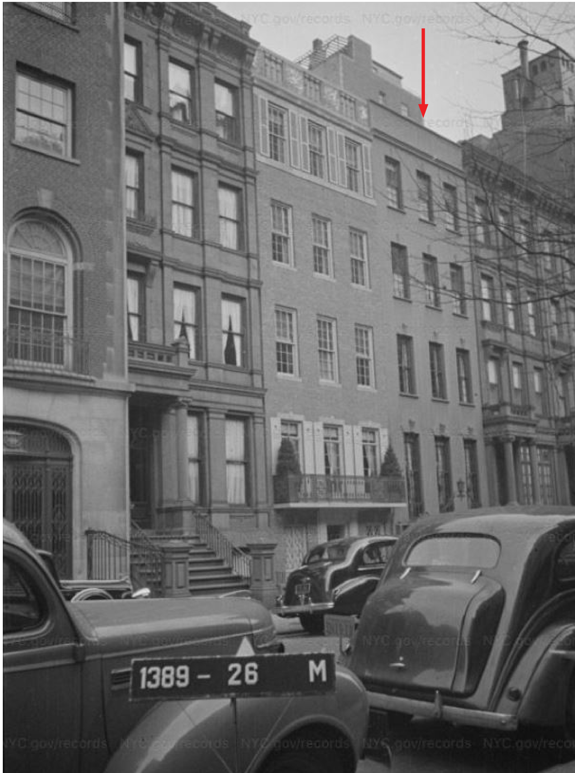
01 HISTORIC 1940 TAX PHOTO LOOKING NORTH N.T.S.
