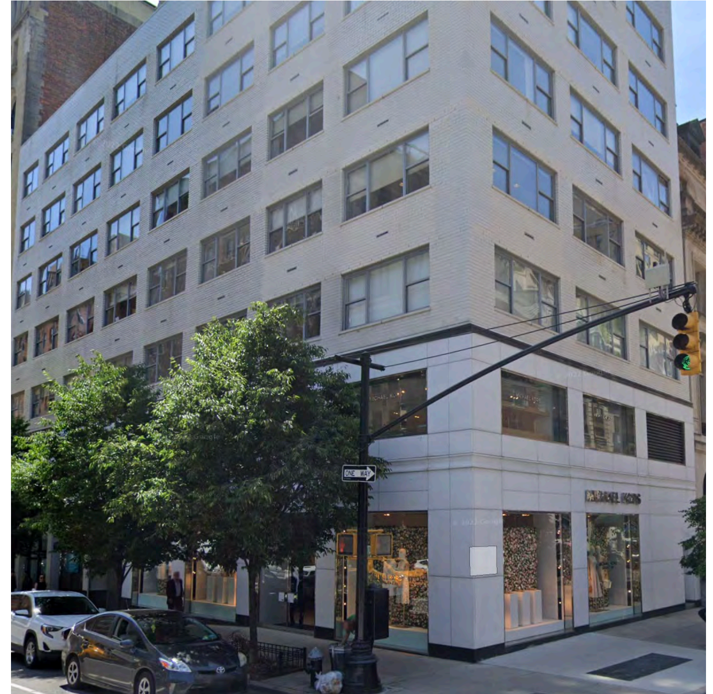
790 Madison Avenue, 2023. 2010 COFA for removal of granite veneer at ground floor and brick from second floor; installation of new masonry cladding at bottom two floors. No style building in UES.
