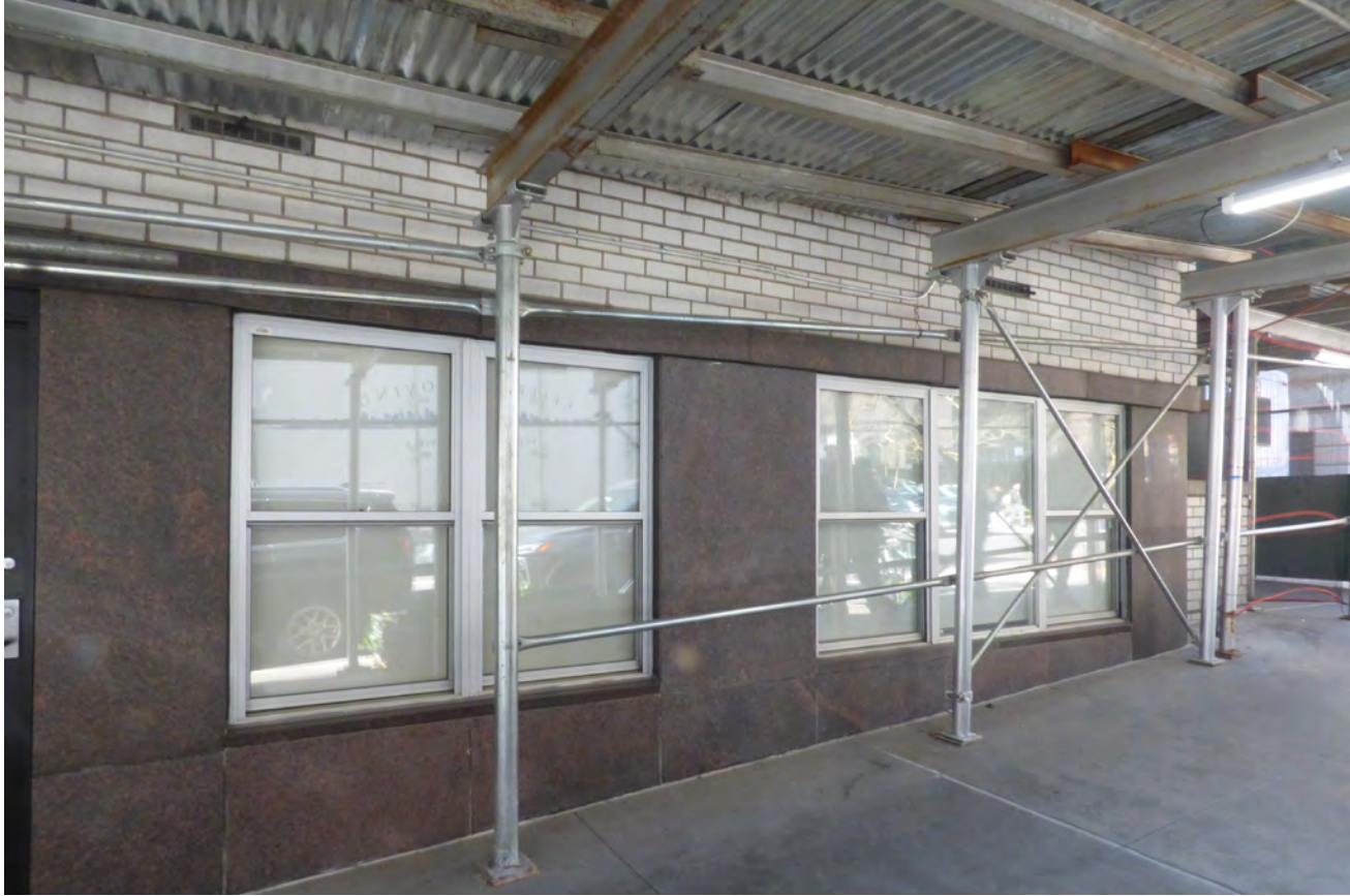
Northern end of Park Avenue base
