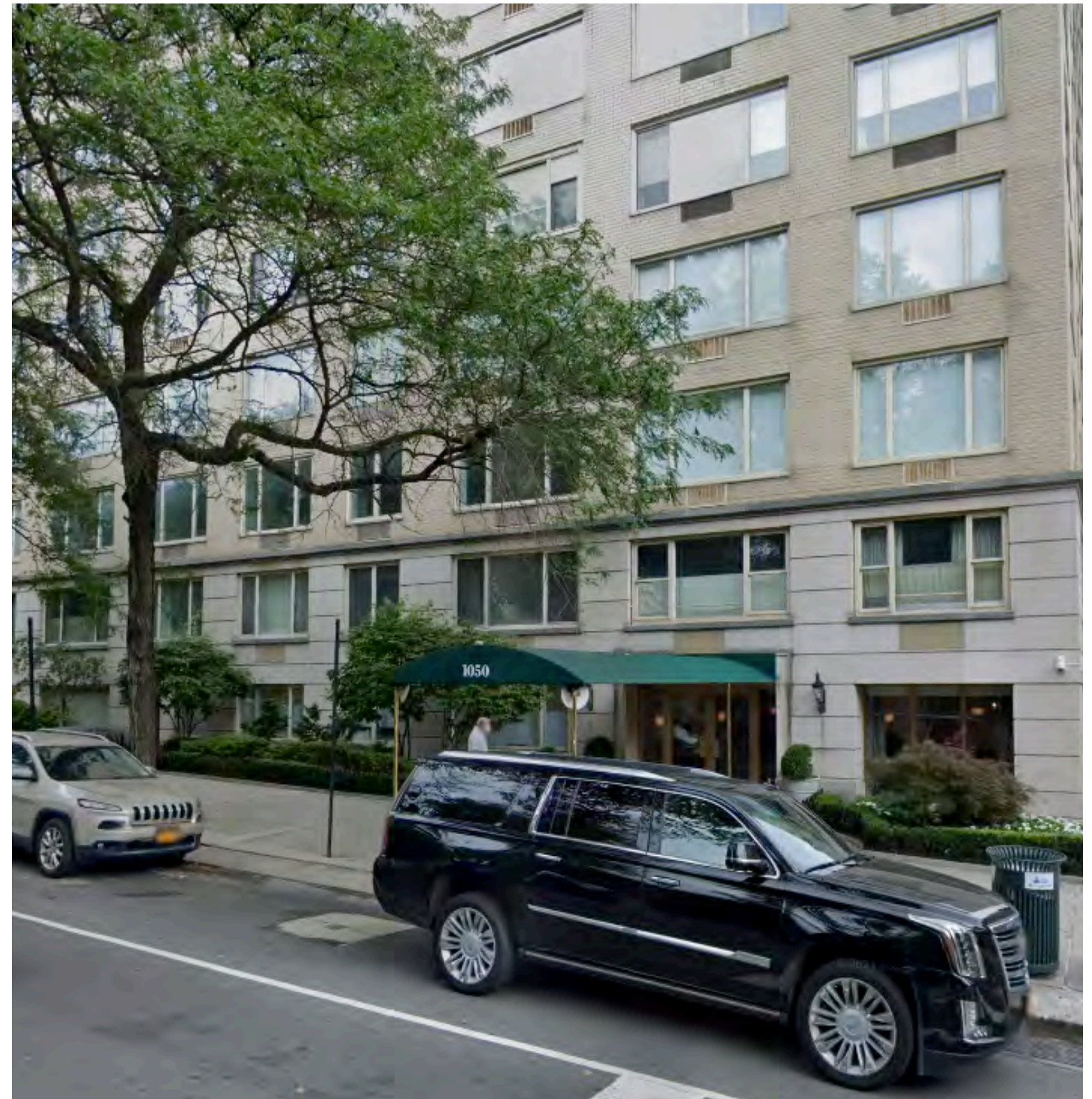
1050 Fifth Avenue, 2004 COFA to remove existing marble cladding at ground floor and brick cladding at the second floor and install new limestone cladding. Contributing building in Carnegie Hill Historic District.
