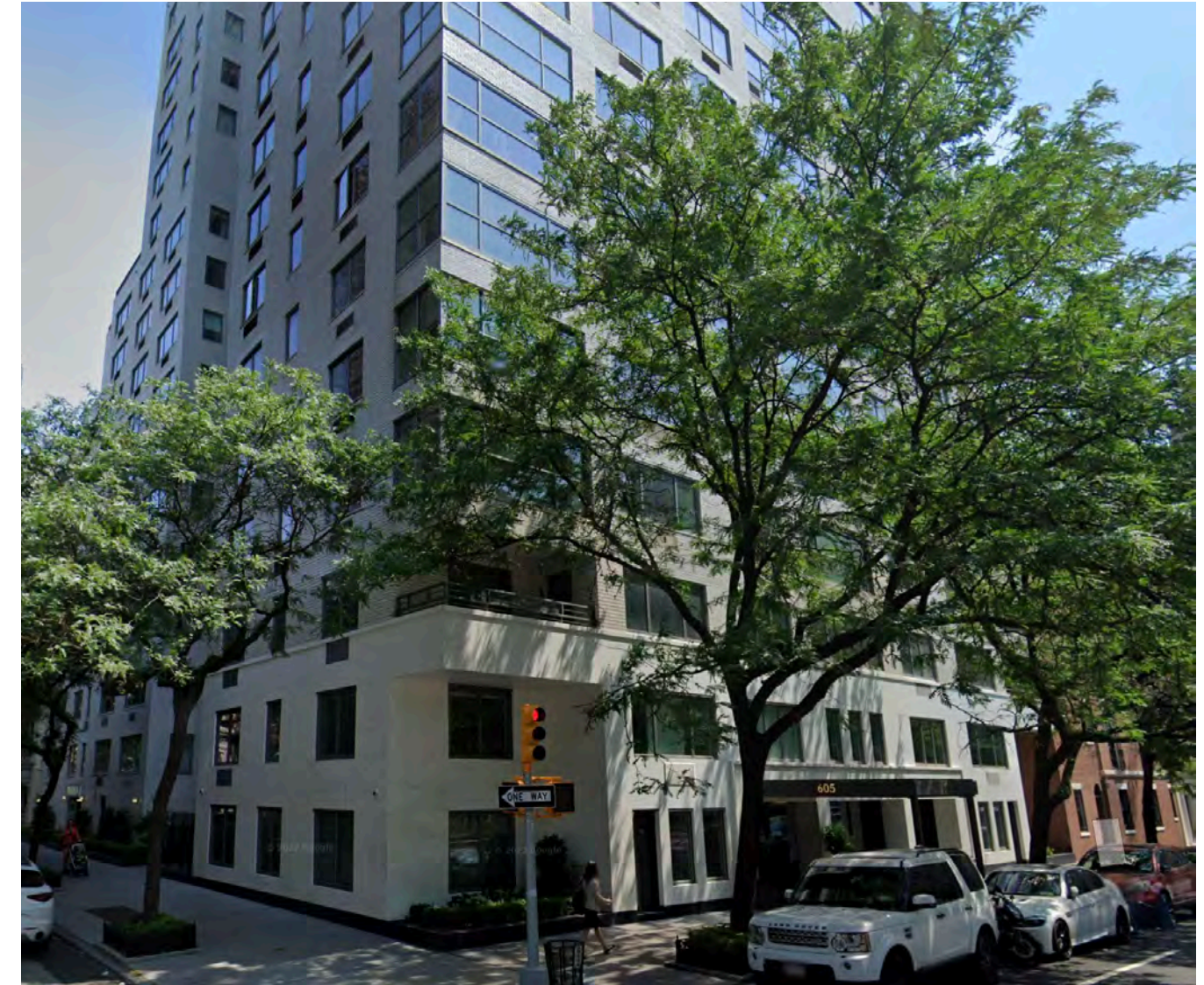
605 Park Avenue. 2016 COFA to remove the first and second floor cladding, and install white marble cladding with a black granite water table.
