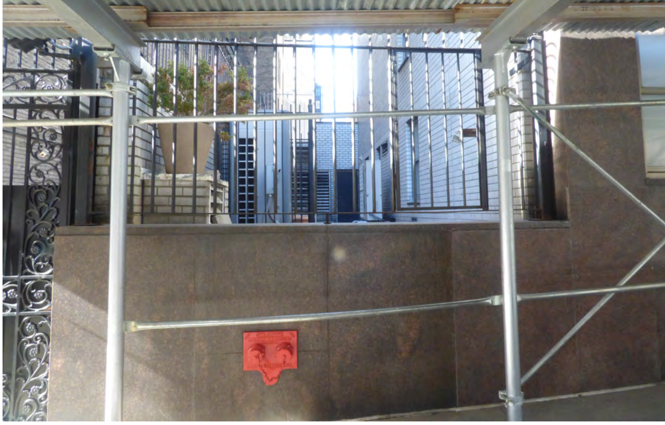
Southern end of Park Avenue base
