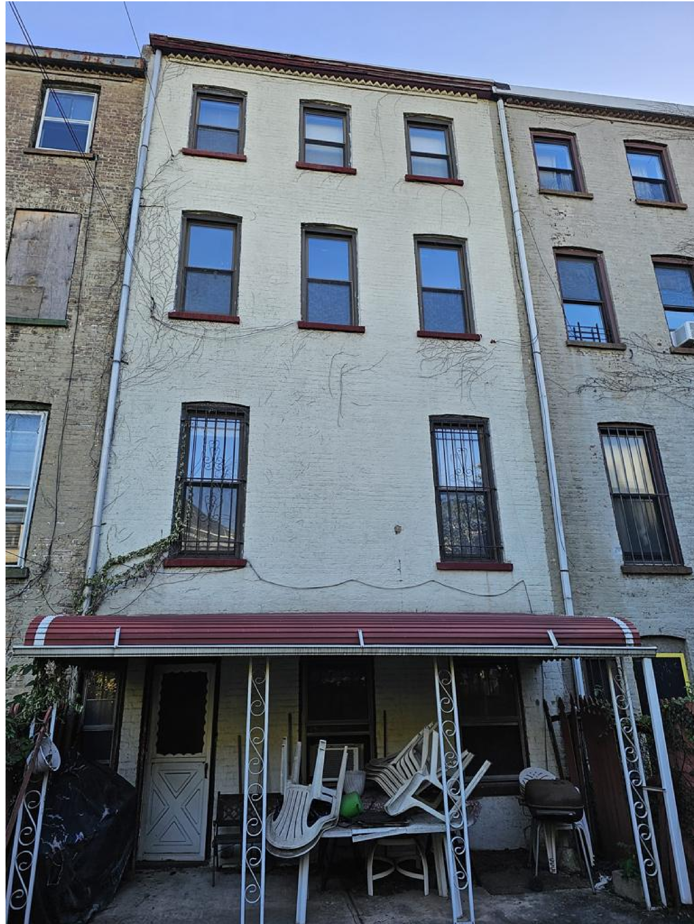
EXISTING CONDITION - GARDEN FACADE
