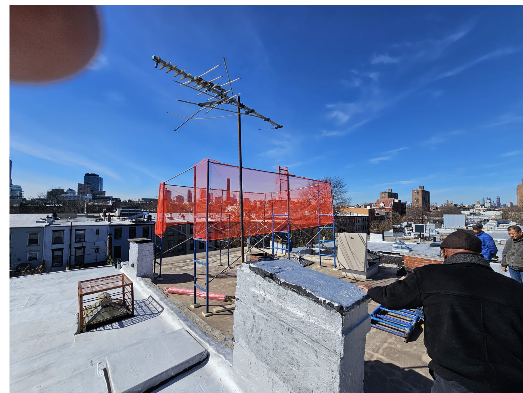
MOCK-UP IN PLACE ON 66 DOWNING STREET
