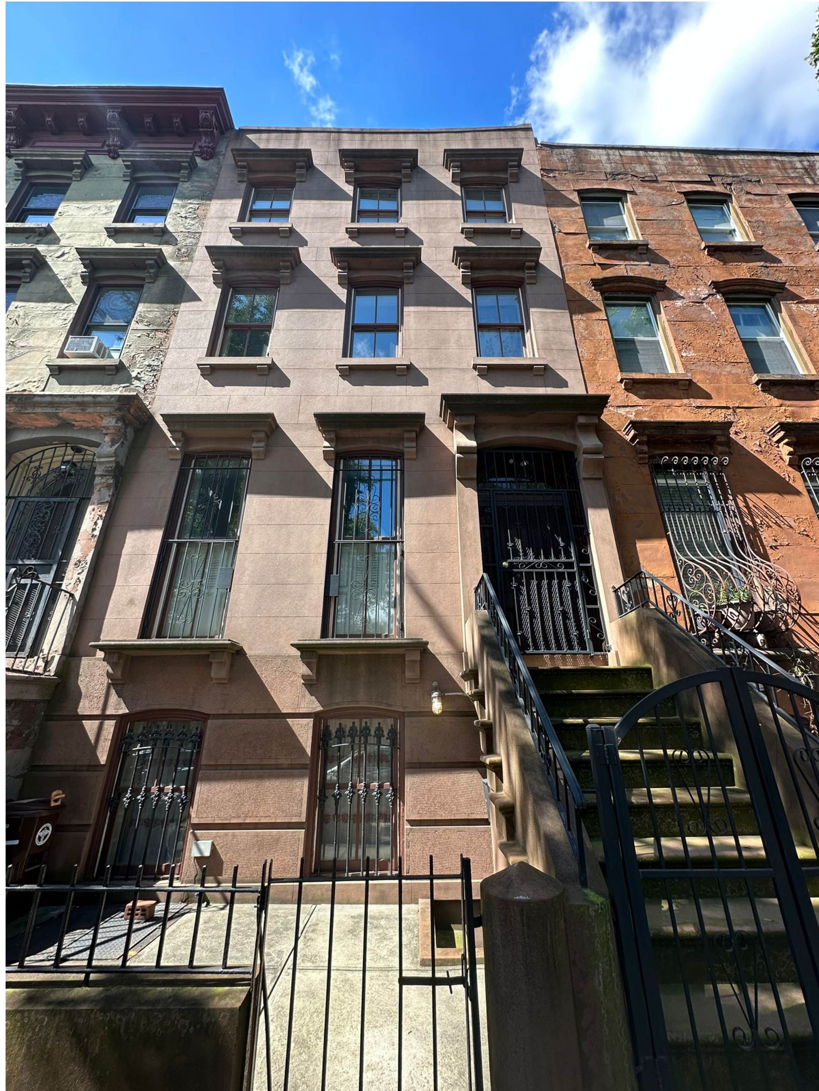
EXISTING CONDITION - STREET FACADE
