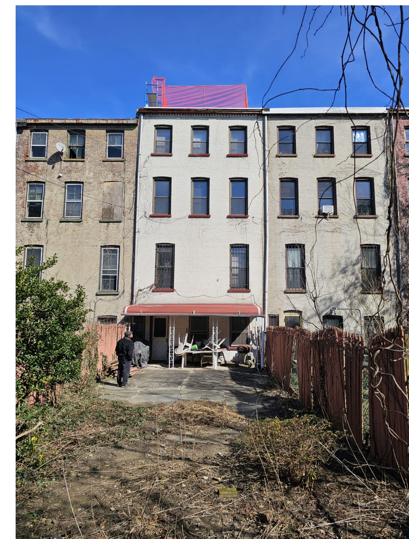
VIEW FROM REAR YARD OF 66 DOWNING ST
