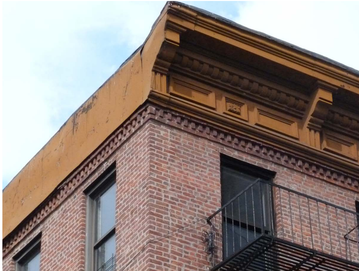
Cornice/parapet Detail
