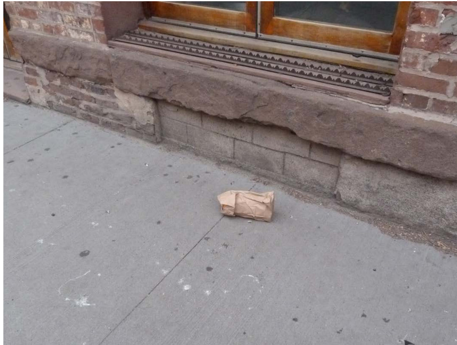
Along Hudson Street- repair work over the years
