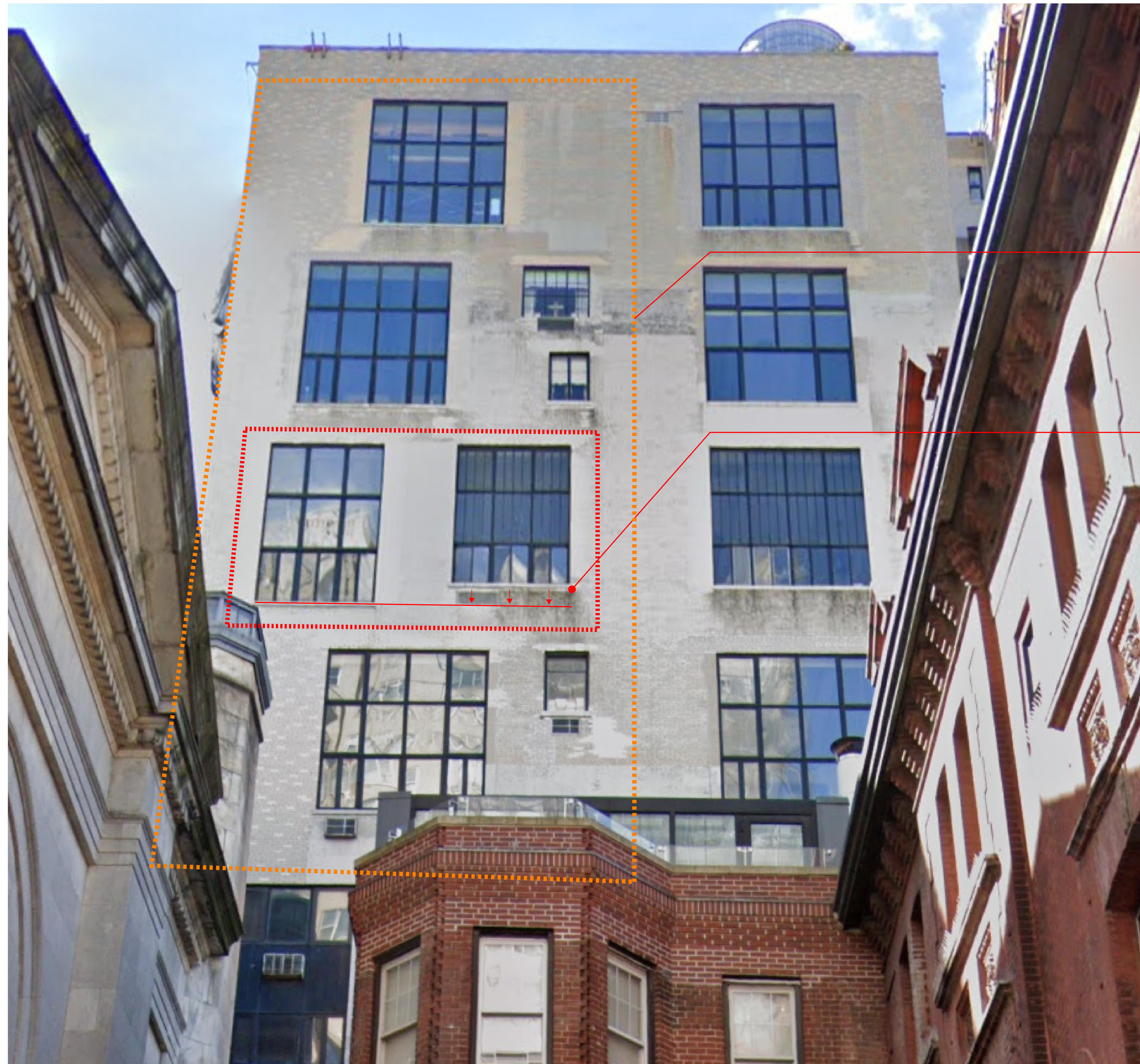
Existing North Facade
