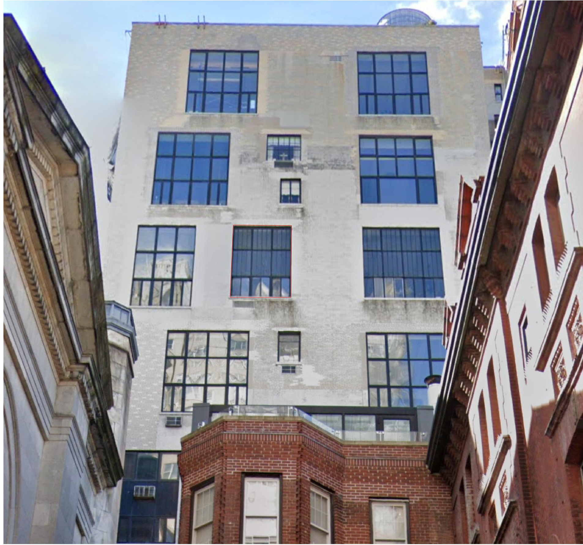
Existing North Facade
