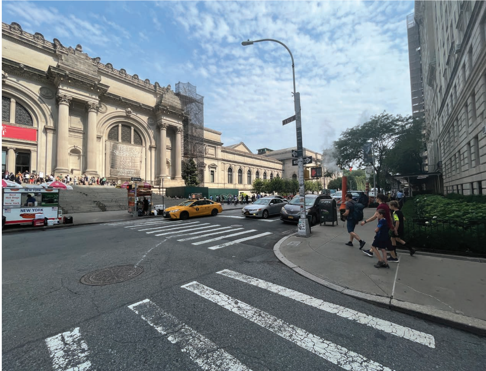
EXISTING CONDITION PHOTO - WING E EXTERIOR
