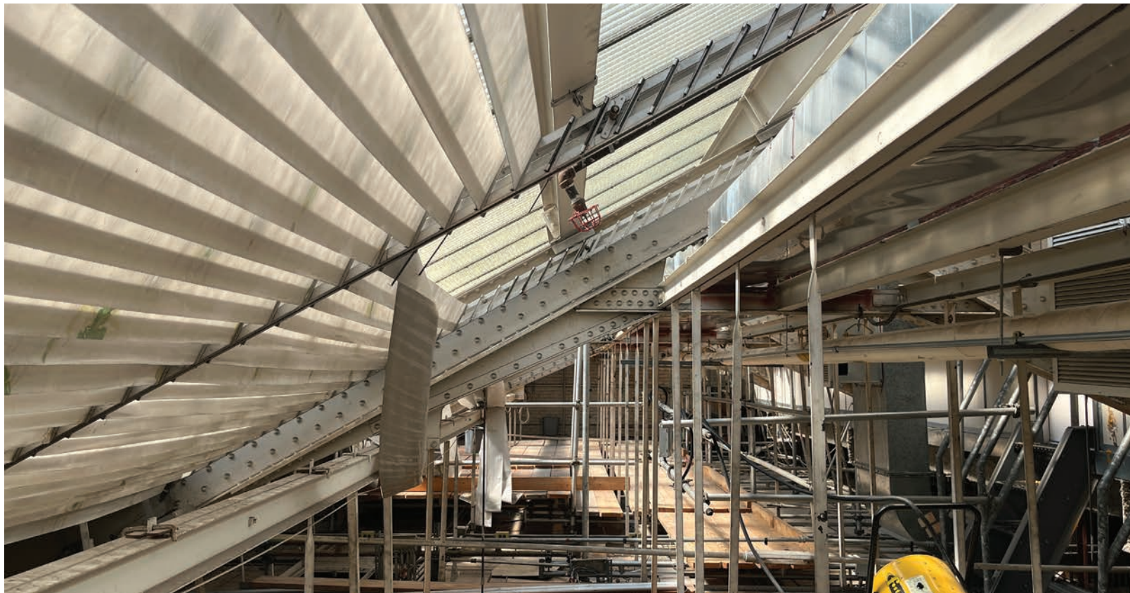
2 EXISTING WING J ATTIC LOOKING SOUTH
