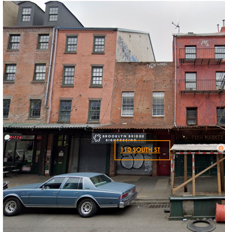
EXISTING CONDITIONS SHOWING SUBSTANTIAL REMOVAL/ LOSS OF HISTORIC BUILDING AREA AND NON-HISTORIC ALTERATIONS TO REMAINING PORTION OF THE BUILDING
