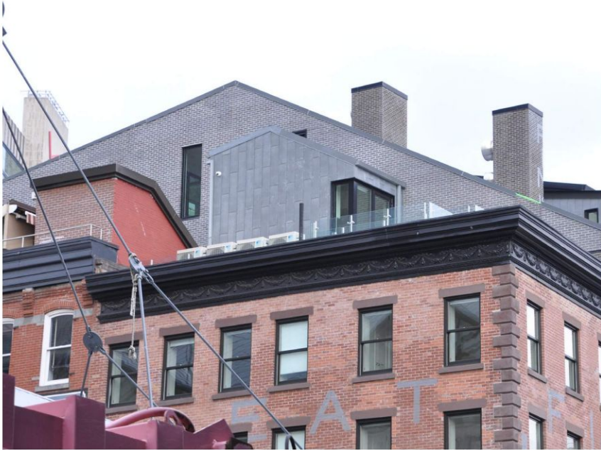
EXISTING VERTICAL EXTENSIONS AT 156 BECKMAN CLOSE UP - BRICK FAÇADE AND METAL ROOF
