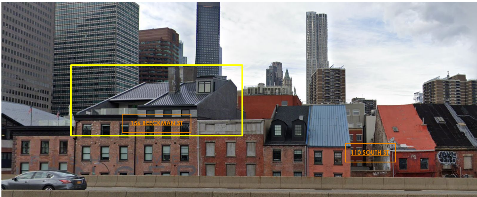
EXISTING VERTICAL ENLARGEMENTS AND ROOF DECKS AT 156 BEECKMAN STREET (added around 2017) ON THE SAME BLOCK
