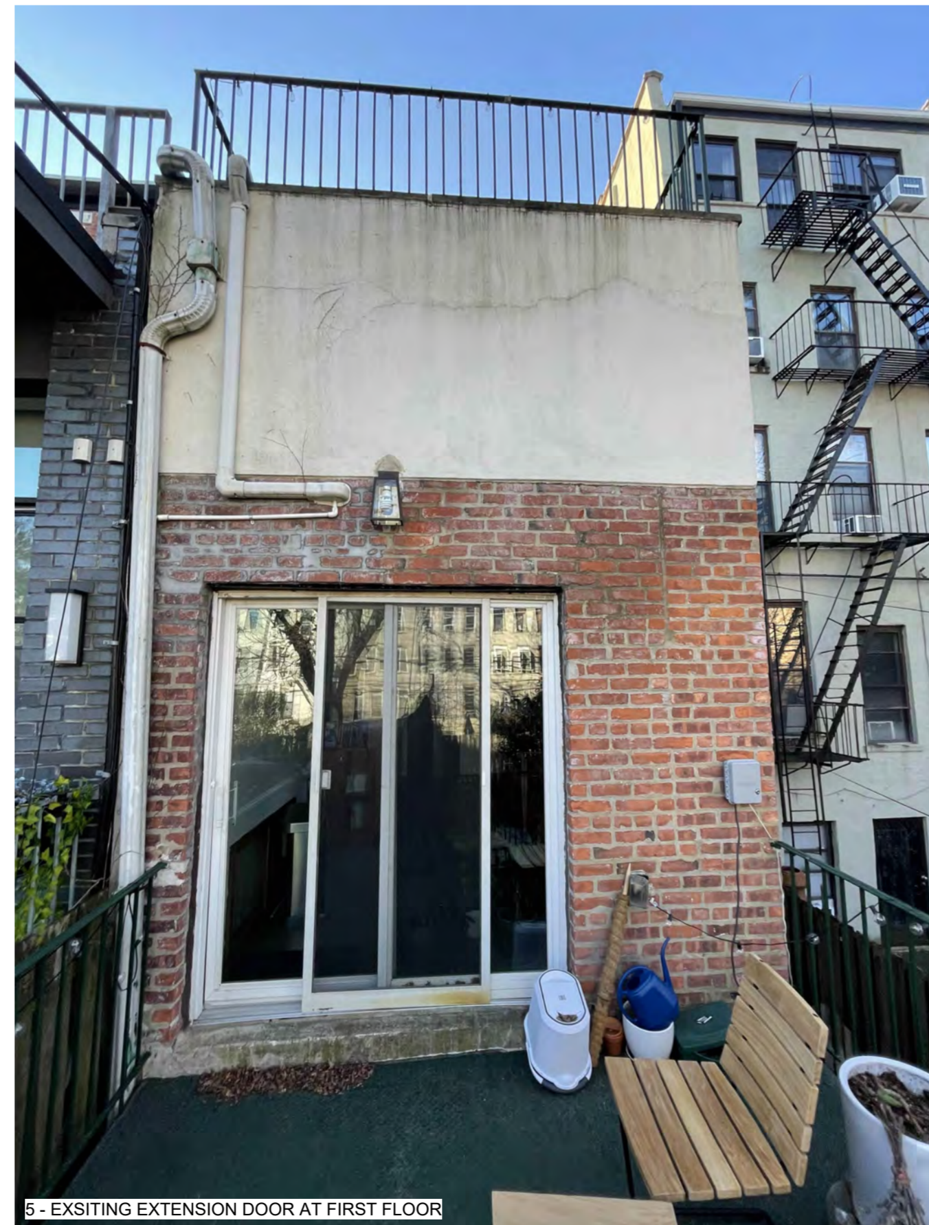
5 - EXSITING EXTENSION DOOR AT FIRST FLOOR
