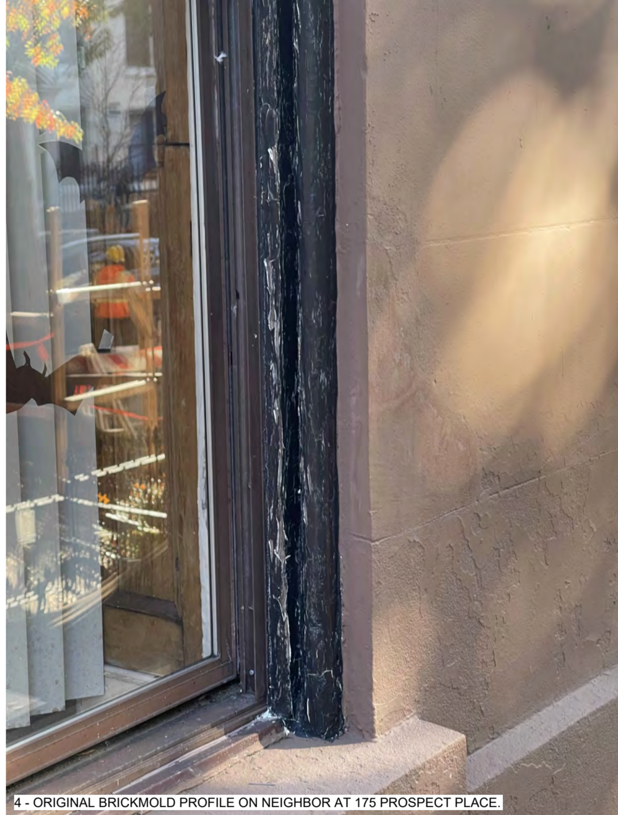
4 - ORIGINAL BRICKMOLD PROFILE ON NEIGHBOR AT 175 PROSPECT PLACE.
