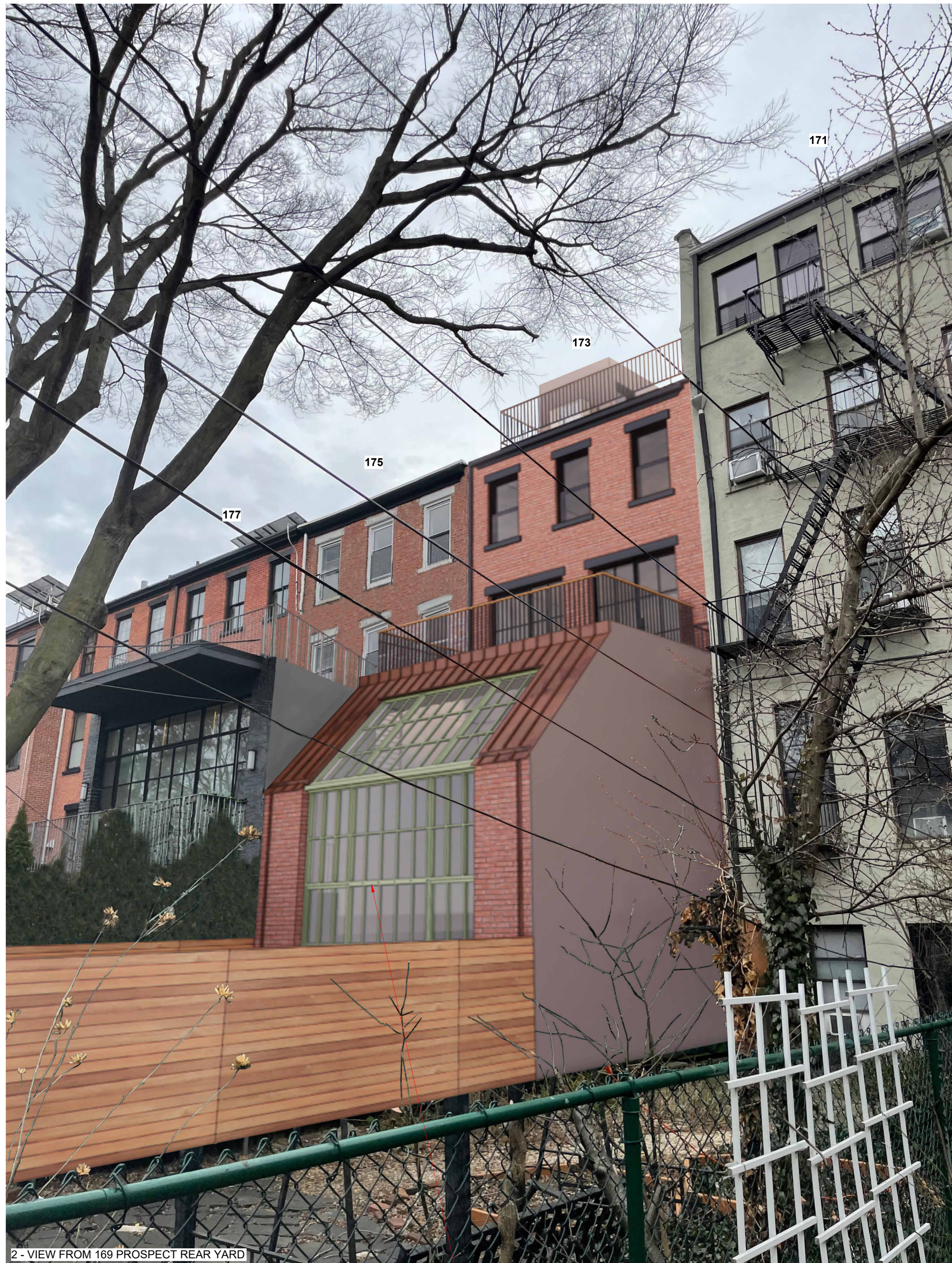
2 - VIEW FROM 169 PROSPECT REAR YARD
