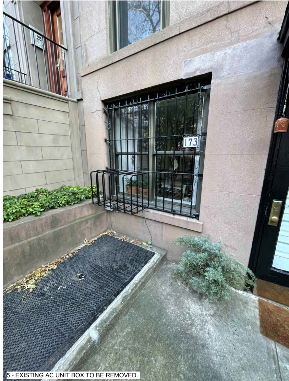
5 - EXISTING AC UNIT BOX TO BE REMOVED.
