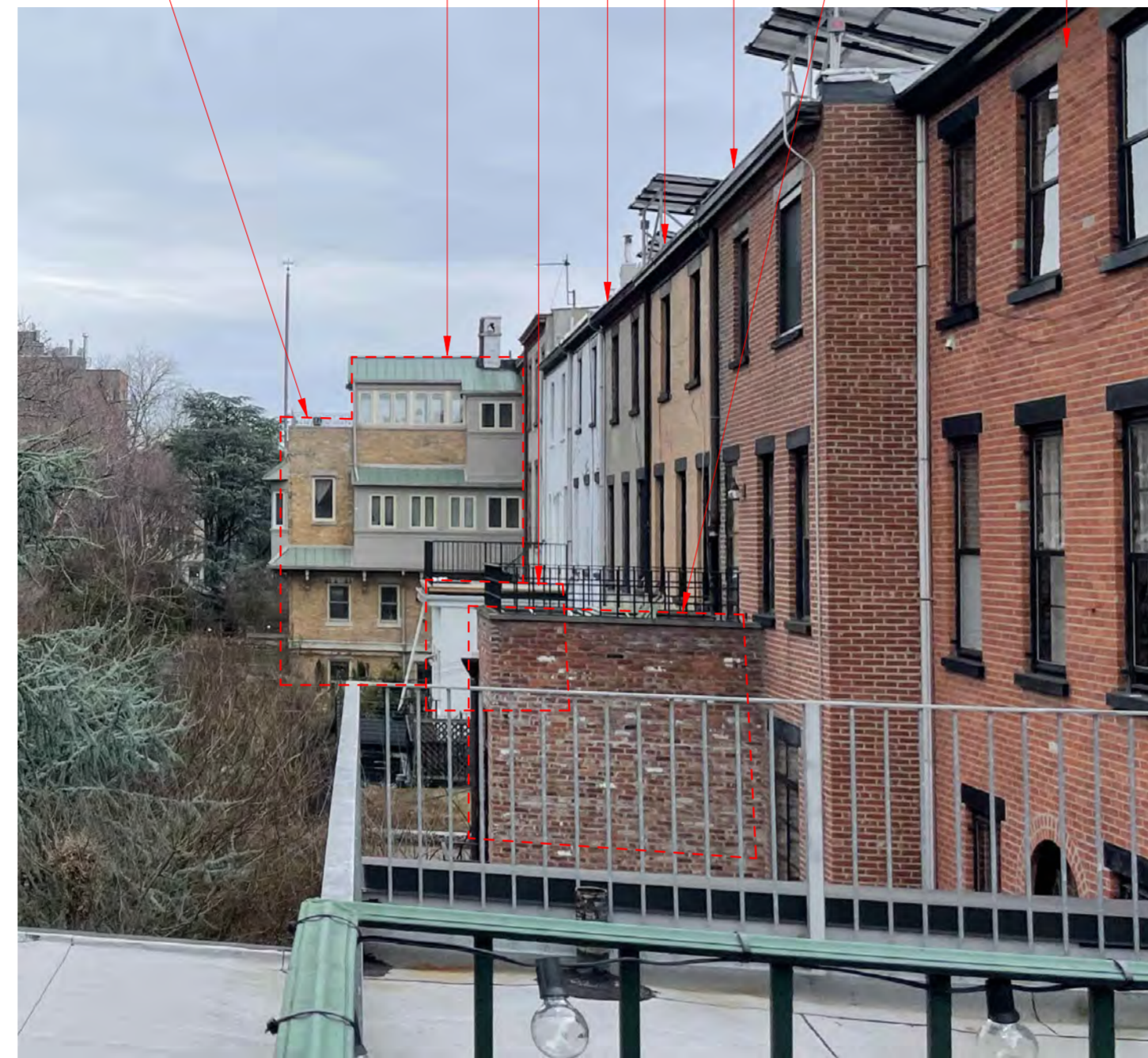
VIEW FROM 173 PROSPECT PLACE EXISTING SECOND STORY ROOF TERRACE
