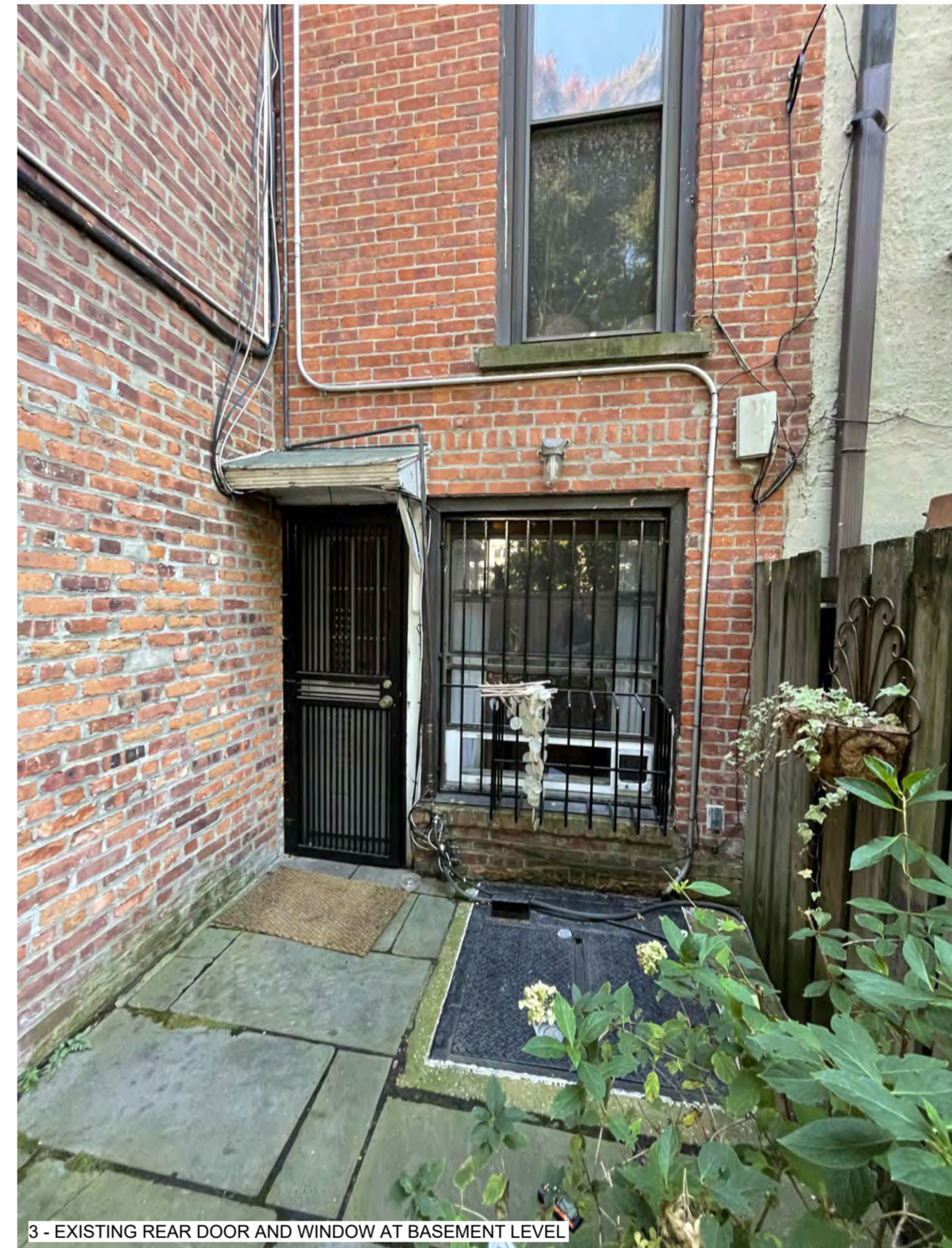
3 - EXISTING REAR DOOR AND WINDOW AT BASEMENT LEVEL
