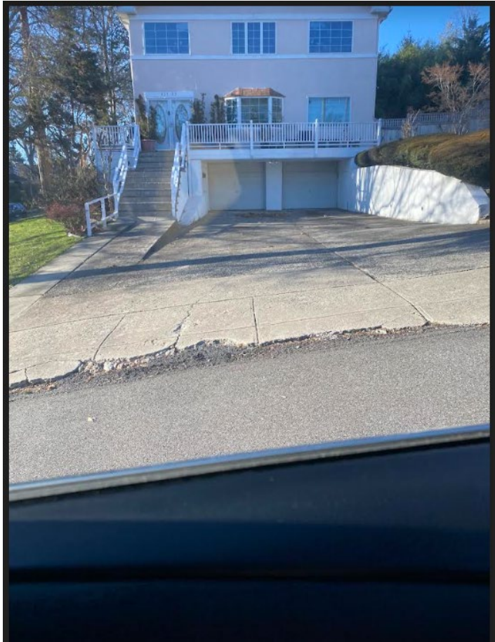
231-05 Hillside Avenue / Center Drive
