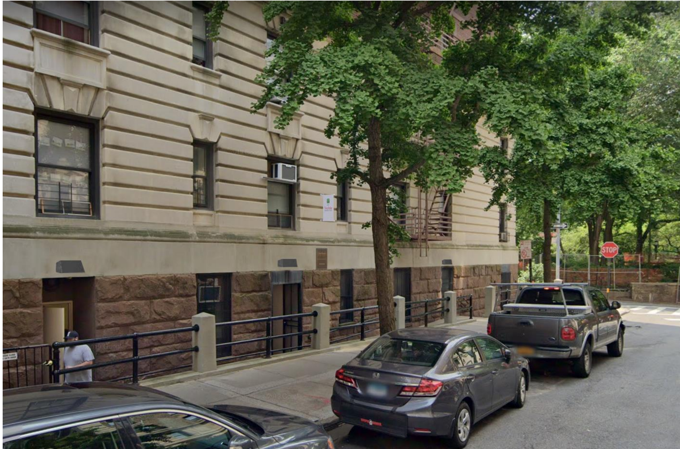
W 93 St Façade Street View Close-up with proposed banner location
