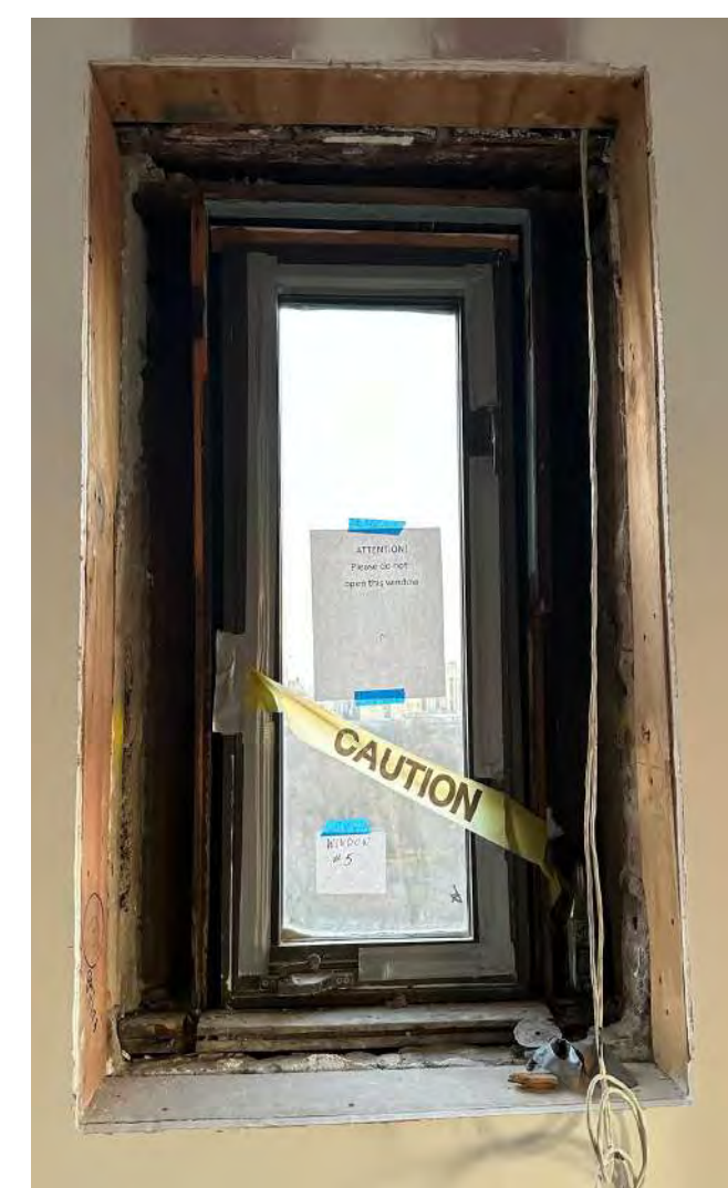
VIEW FROM INTERIOR
