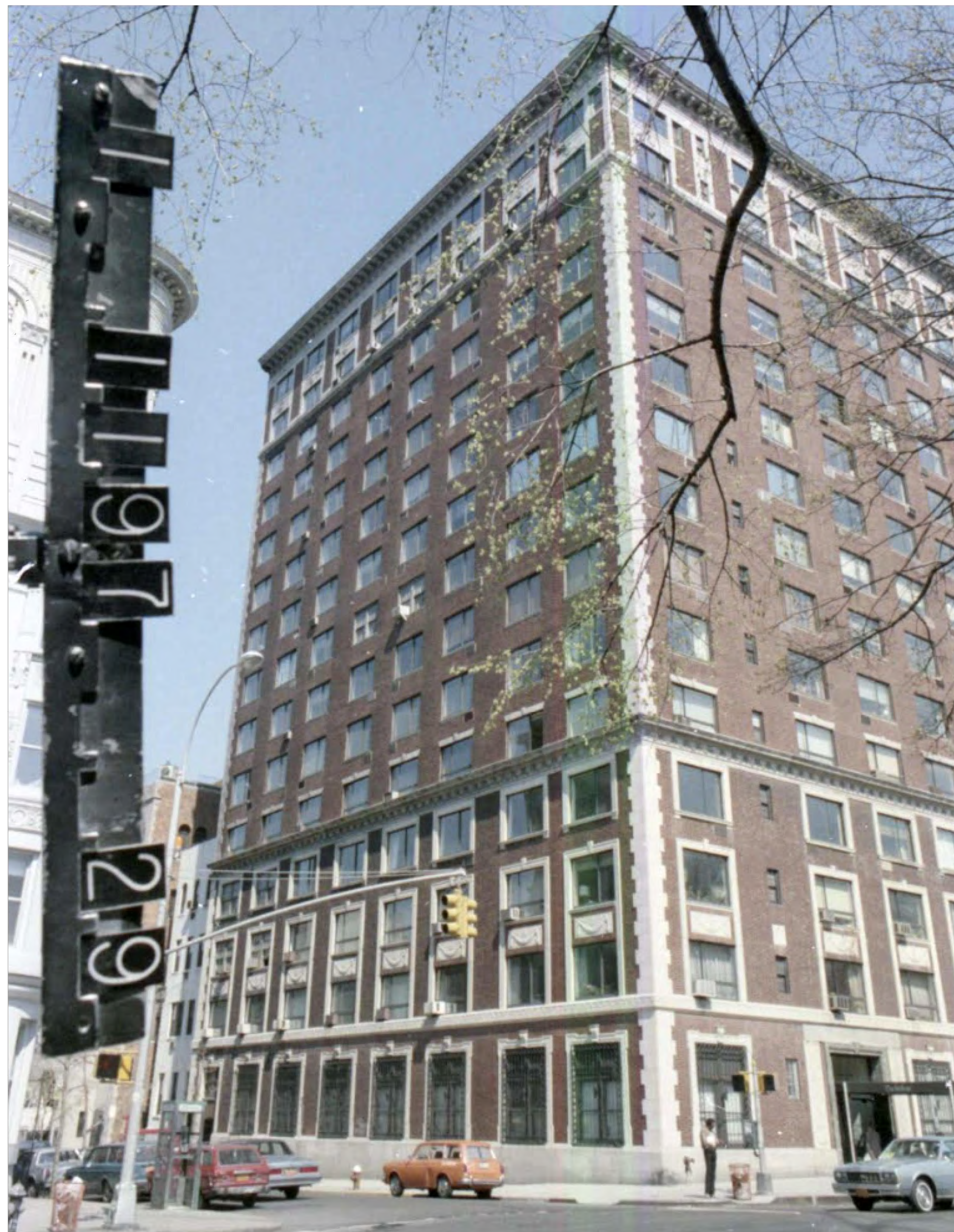
EXISTING "HISTORIC" SLIDING WINDOWS, 230 CENTRAL PARK WEST TAX PHOTO (1980s)
