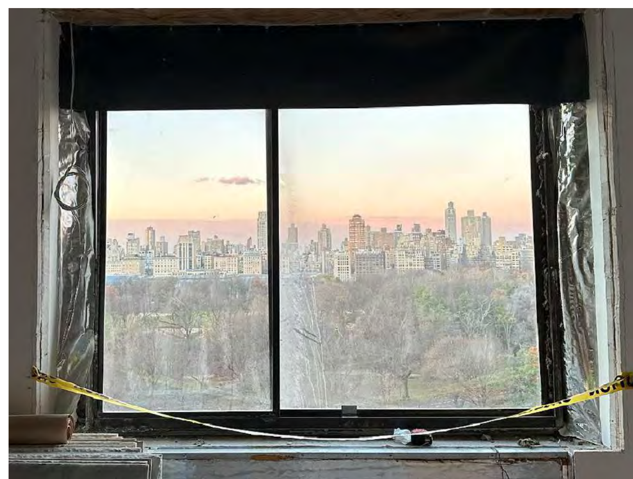
VIEW FROM INTERIOR
