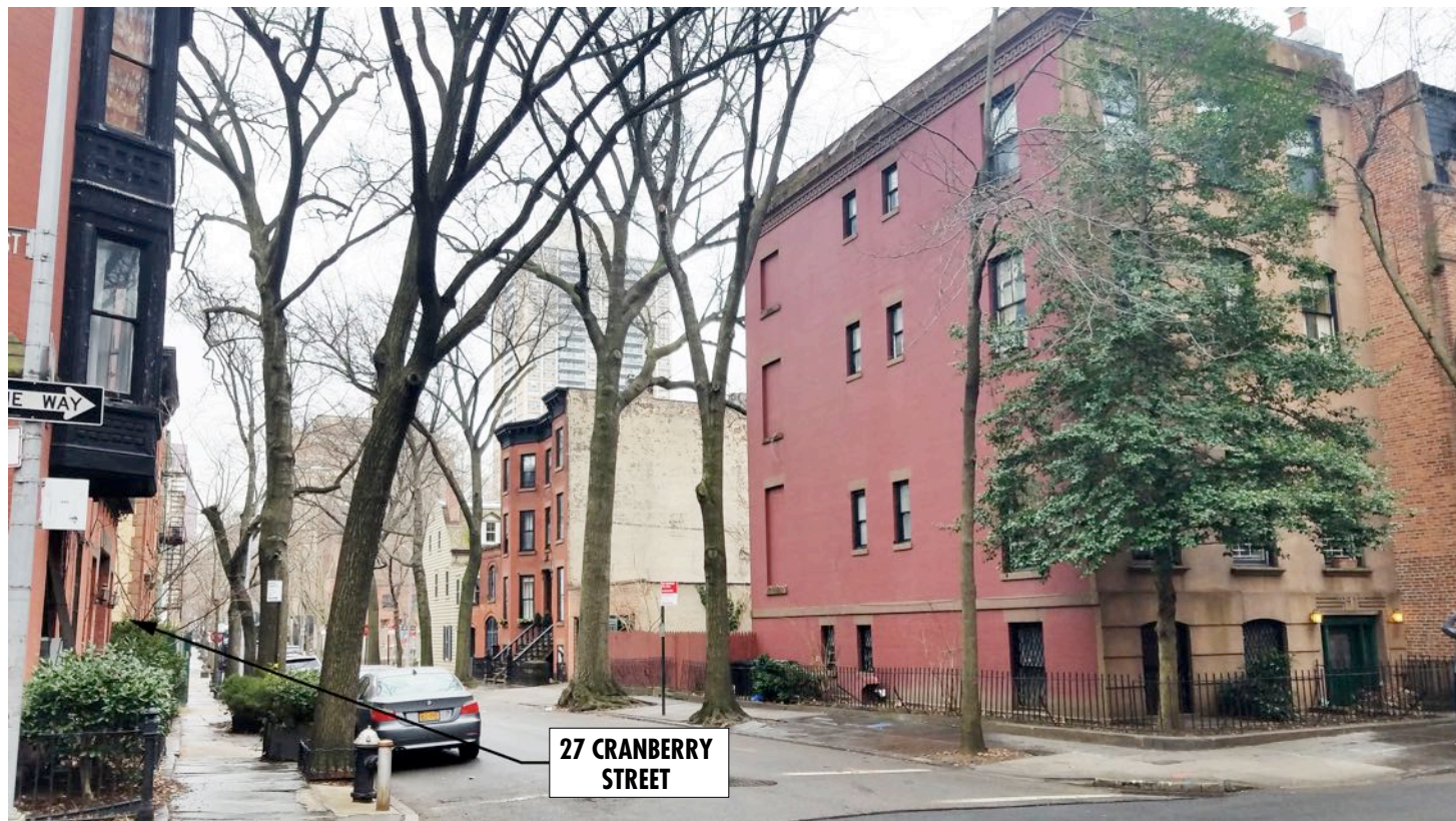
VIEW 2 - CORNER CRANBERRY STREET & WILLOW STREET SOUTH SIDE
