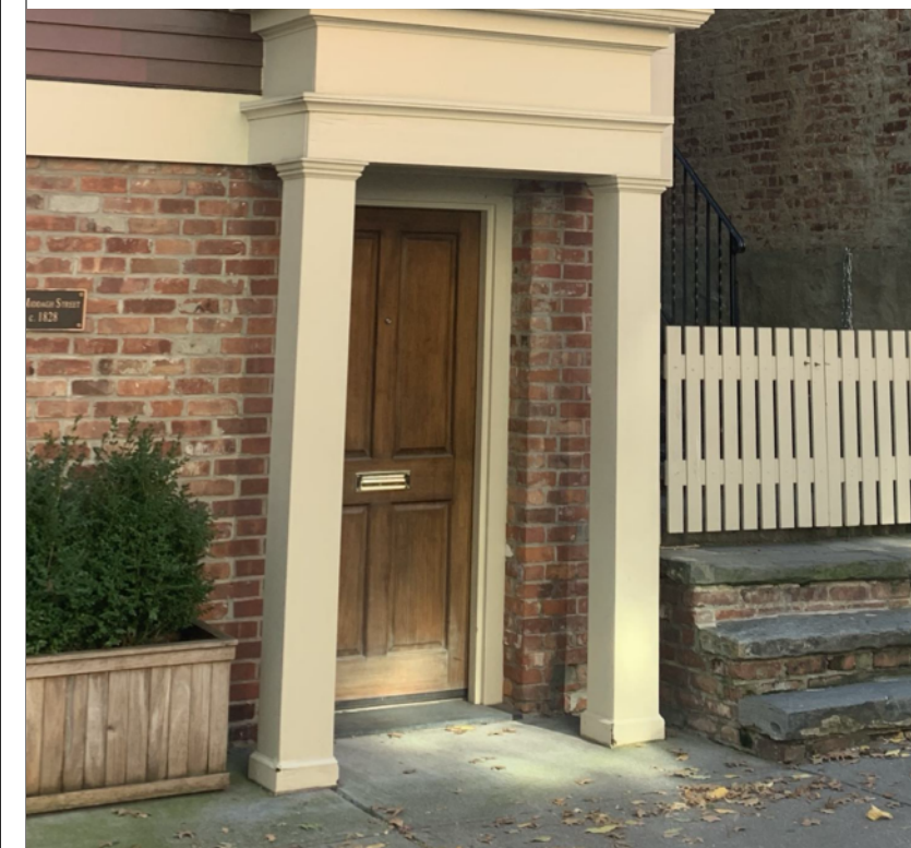
MIDDAGH STREET, COLUMN FRAMING ENTRANCE
