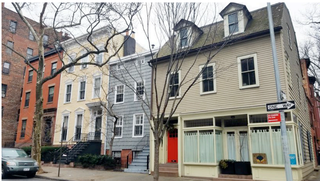
VIEW 3 - HICKS STREET
