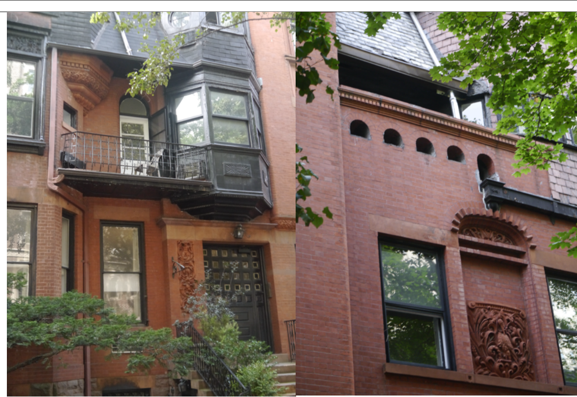
WILLOW STREET ATYPICAL BALCONIES, ROOF TERRACES
