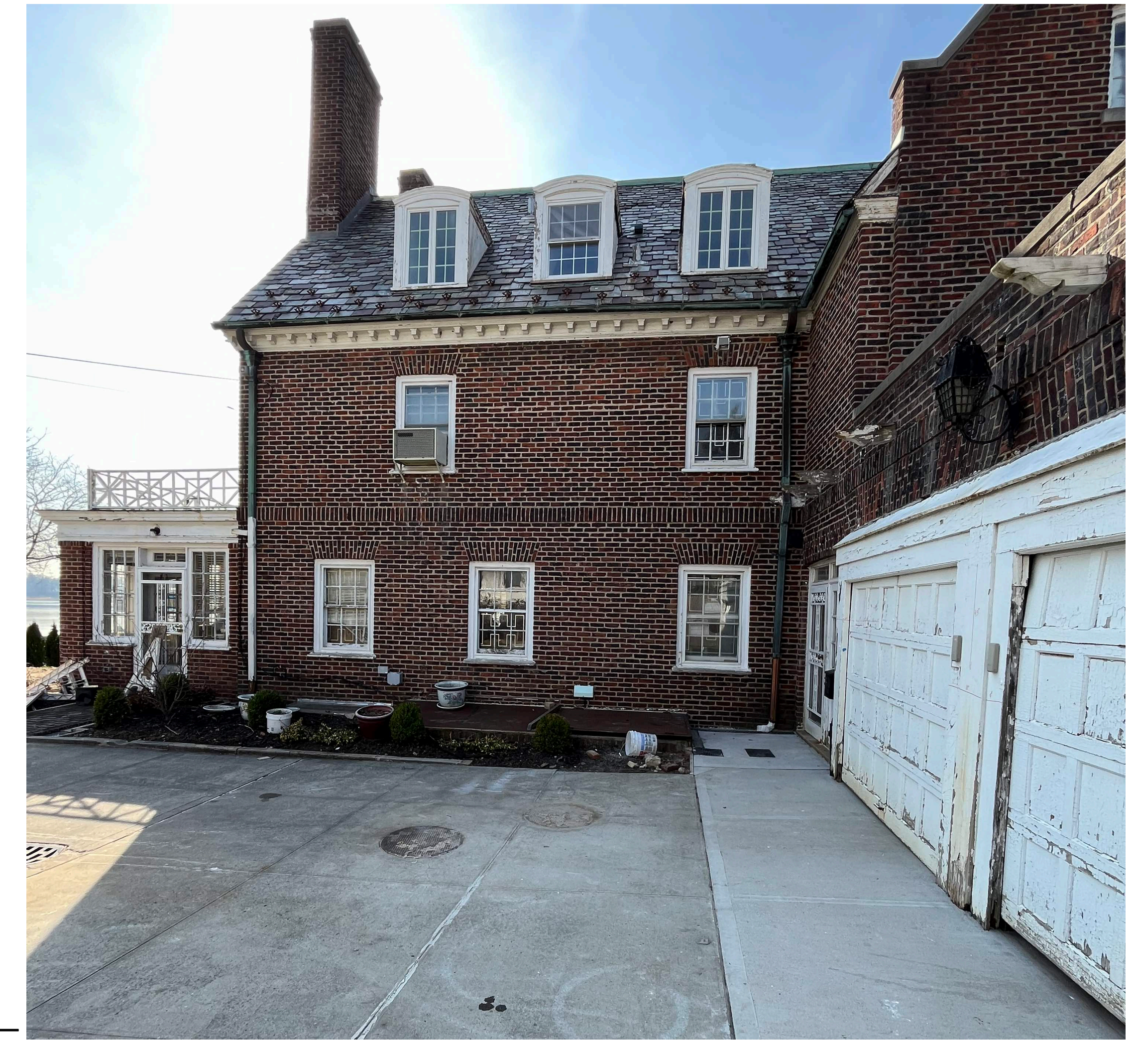
EXISTING CONDITIONS EAST FACADE FACING DRIVEWAY
