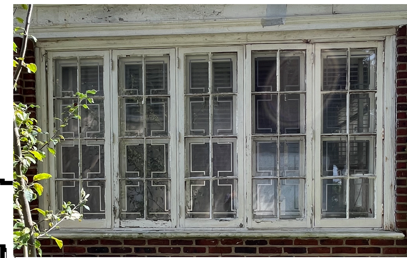
EXISTING FIVE SASH CASEMENT WINDOW
