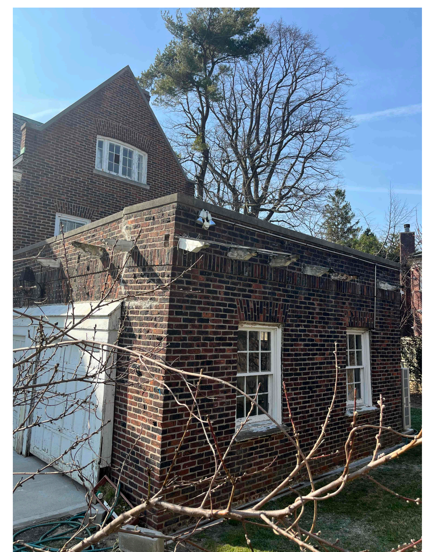
EXISTING CONDITIONS EAST FACADE GARAGE WING
