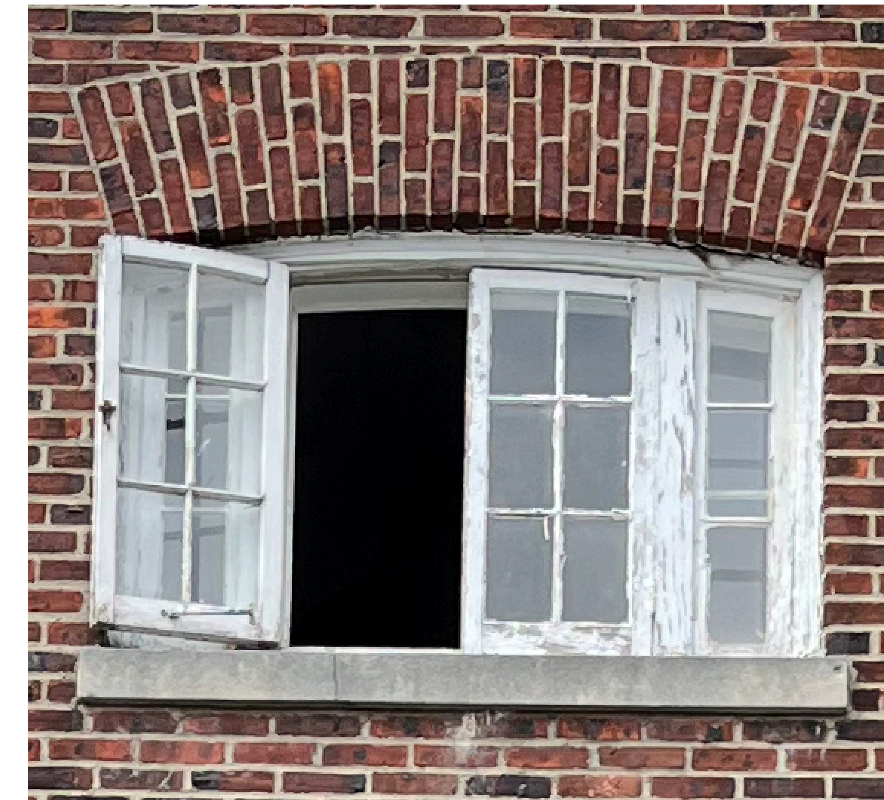
EXISTING CASEMENT ATTIC EAST ELEVATION
