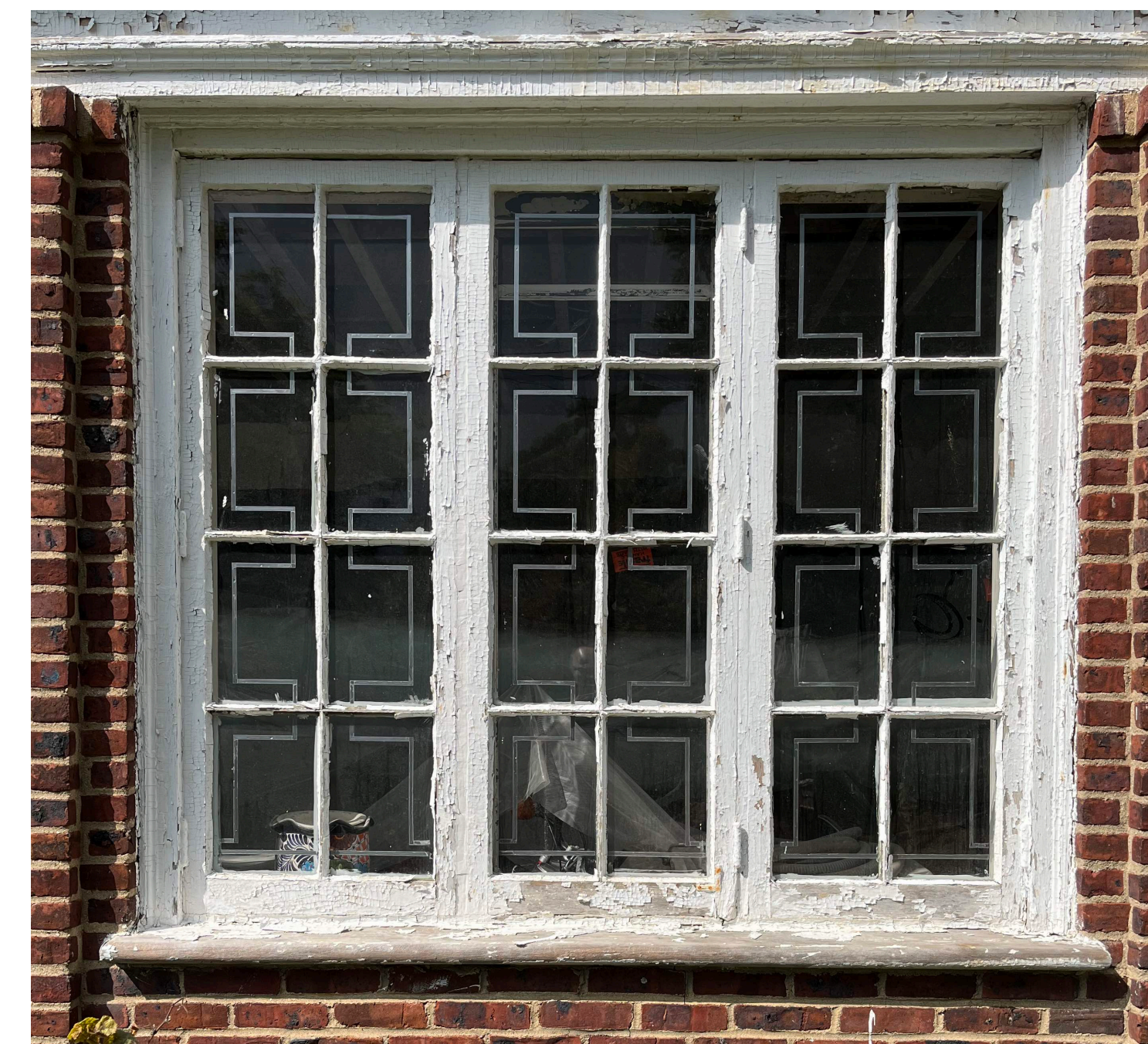
TYPICAL THREE SASH CASEMENT WINDOW - EXISTING CONDITIONS
