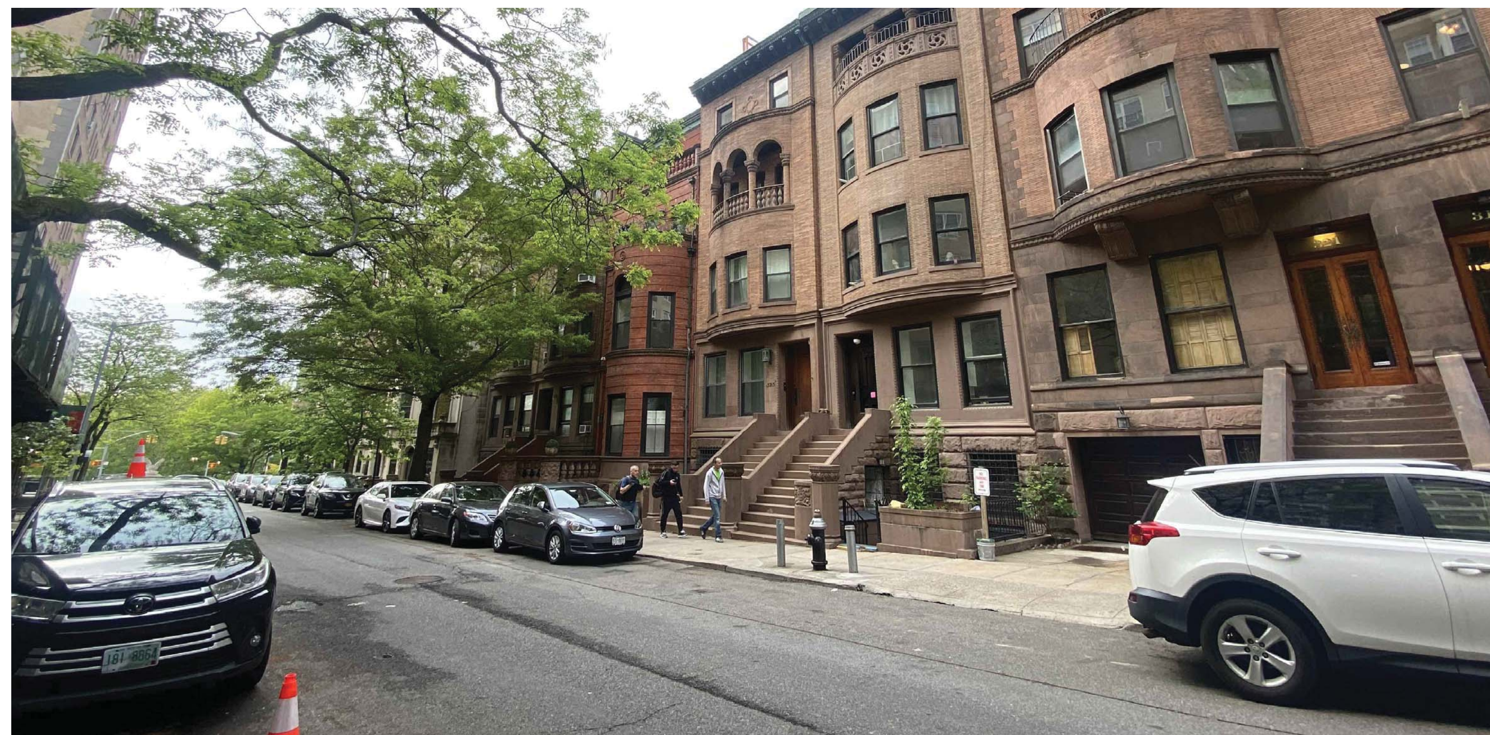
327 WEST 76TH STREET - LOOKING WEST
