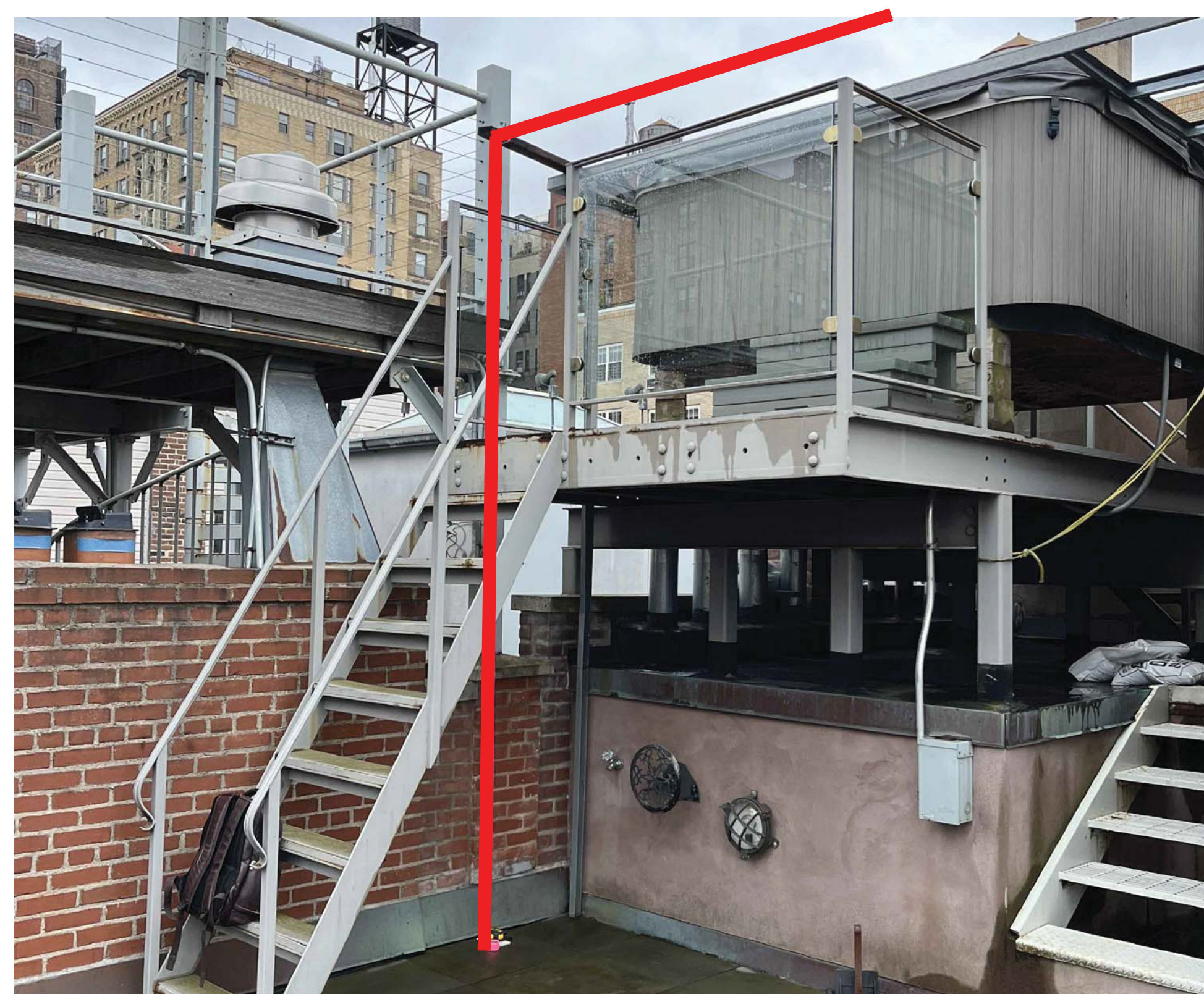
PENTHOUSE MOCKUP SOUTHEAST CORNER VIEW
