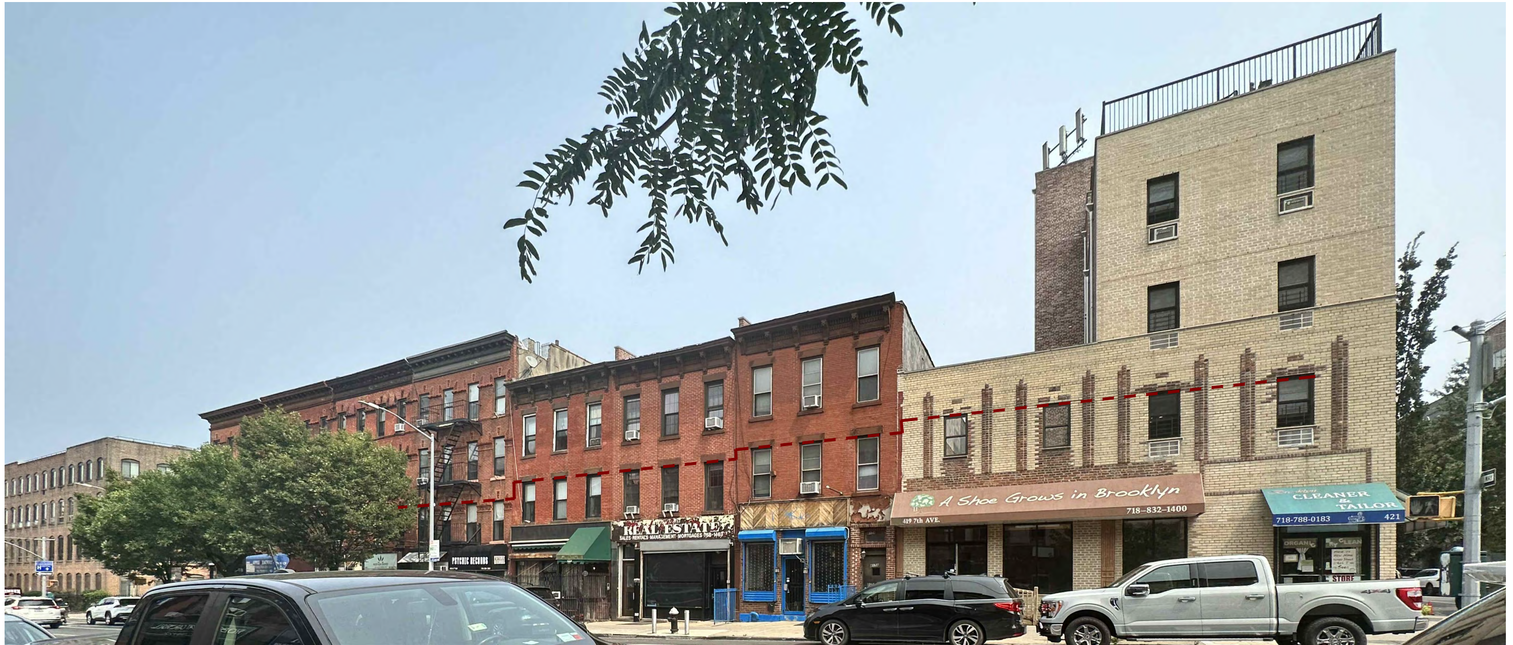
STREET VIEW FROM 7TH AVE BLOCK: 1100 VIEW A
