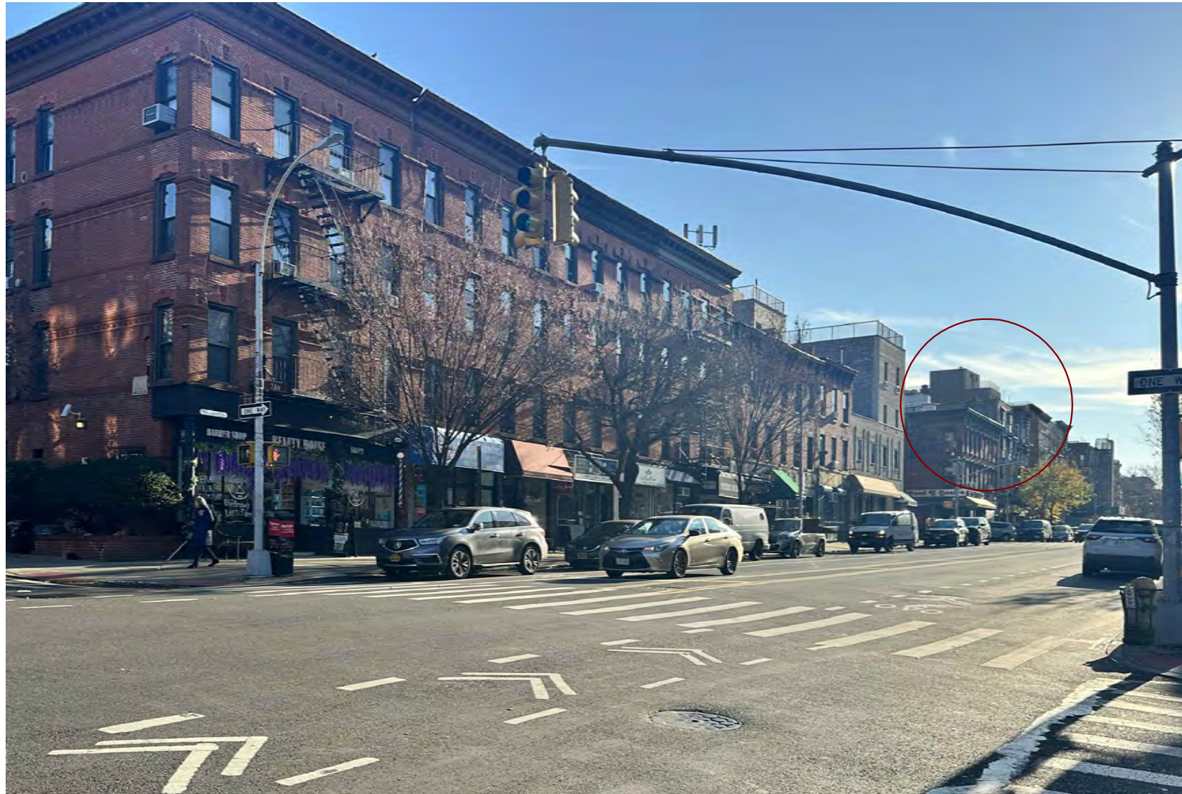
VIEW FROM INTERSECTION AT 13TH STREET AND 7TH AVE
