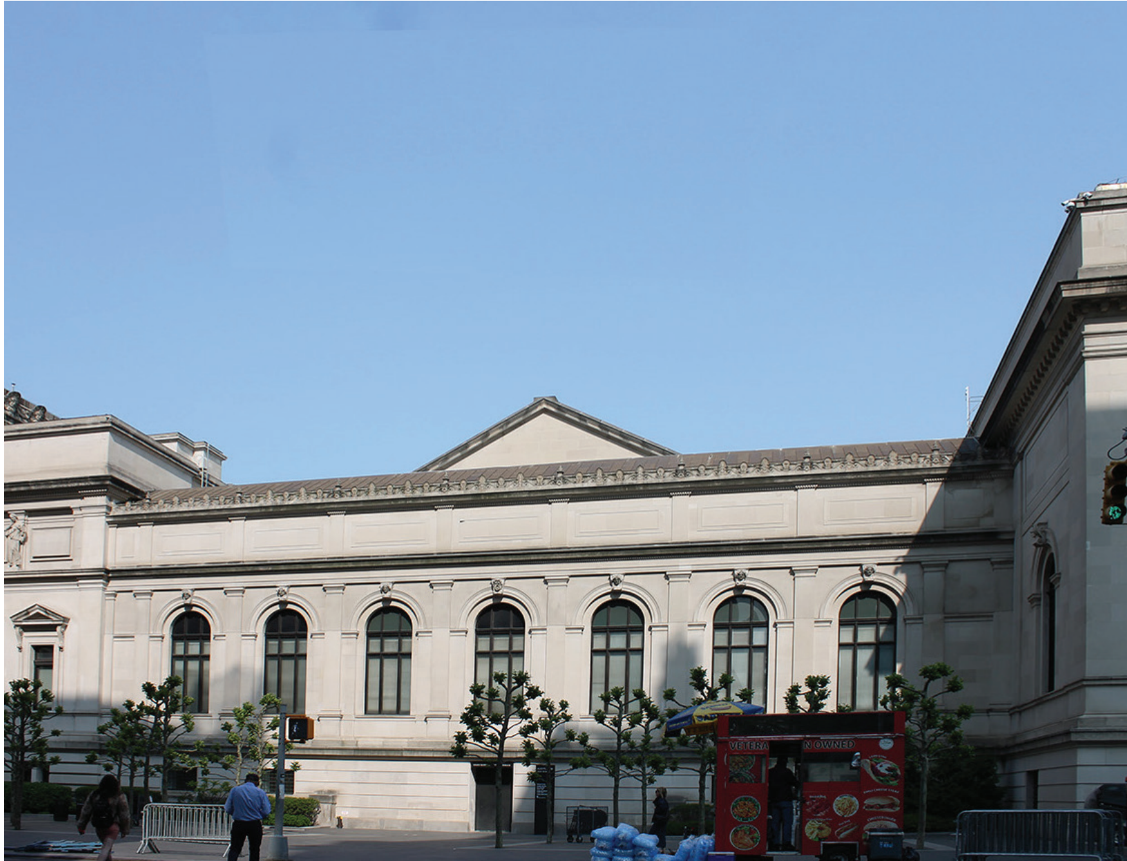
EXISTING CONDITION PHOTO - WING J EXTERIOR
