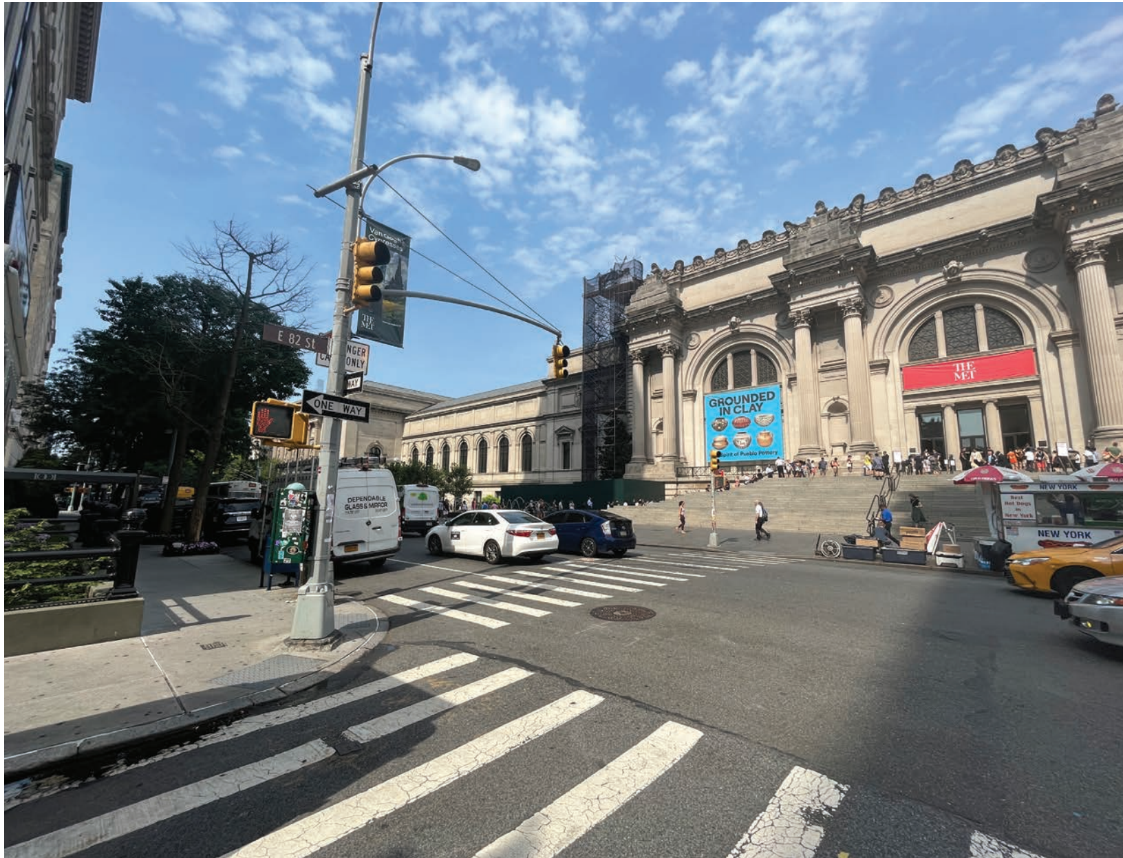
EXISTING CONDITION PHOTO - WING J EXTERIOR
