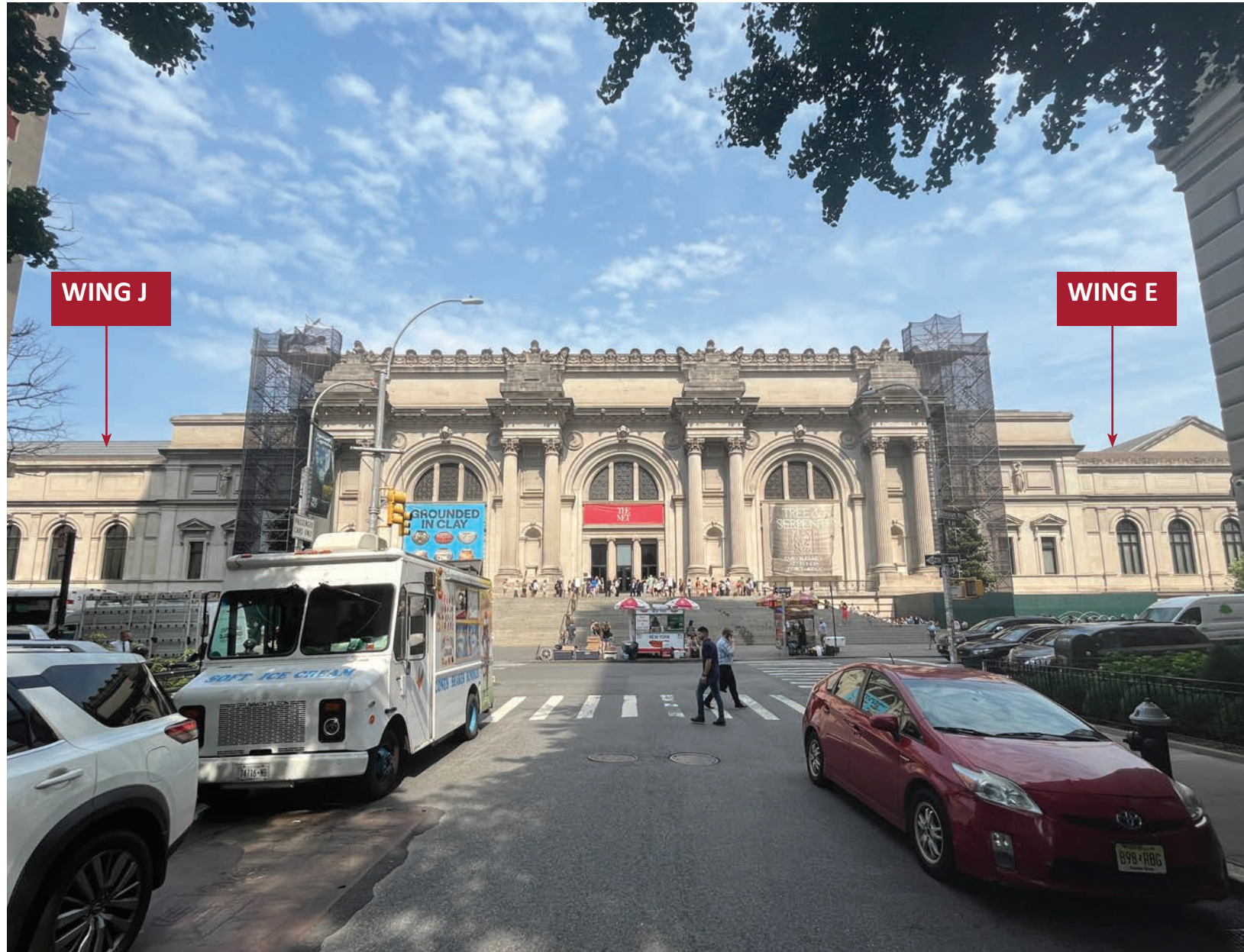
EXISTING CONDITION PHOTO WINGS J AND E
