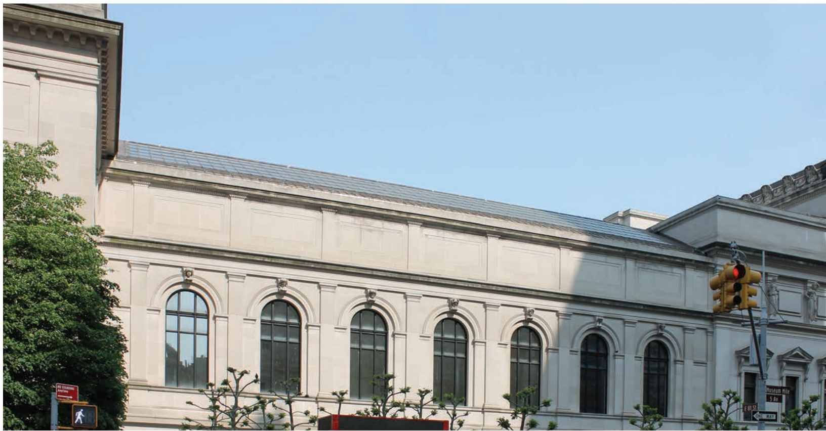
EXISTING CONDITION PHOTO - WING J SKYLIGHT
