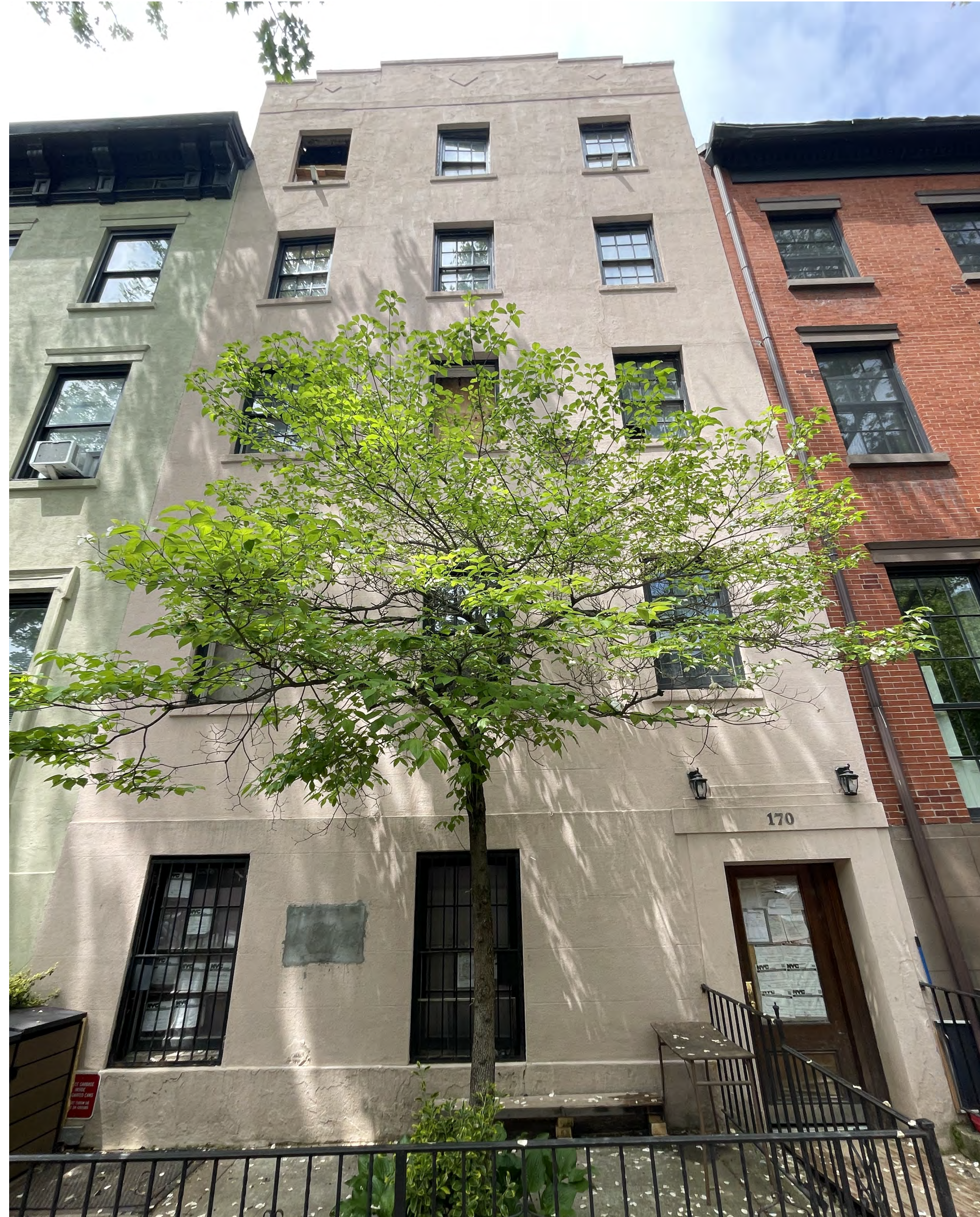
EXISTING FRONT FACADE
