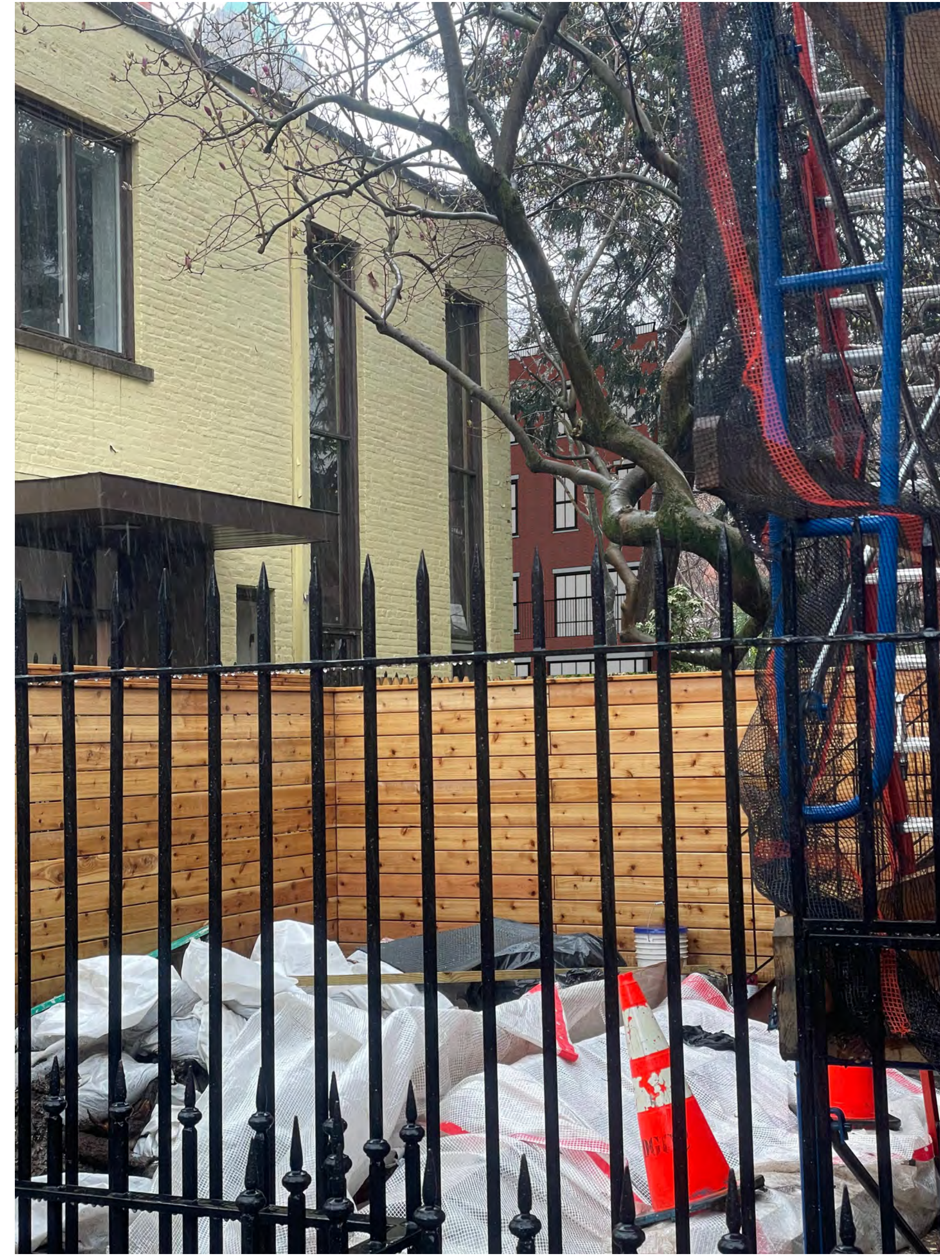
VIEW OF PROPOSED REAR FACADE FROM SIDNEY PLACE. VIEW OBSTRUCTED BY EXISTING VEGETATION
