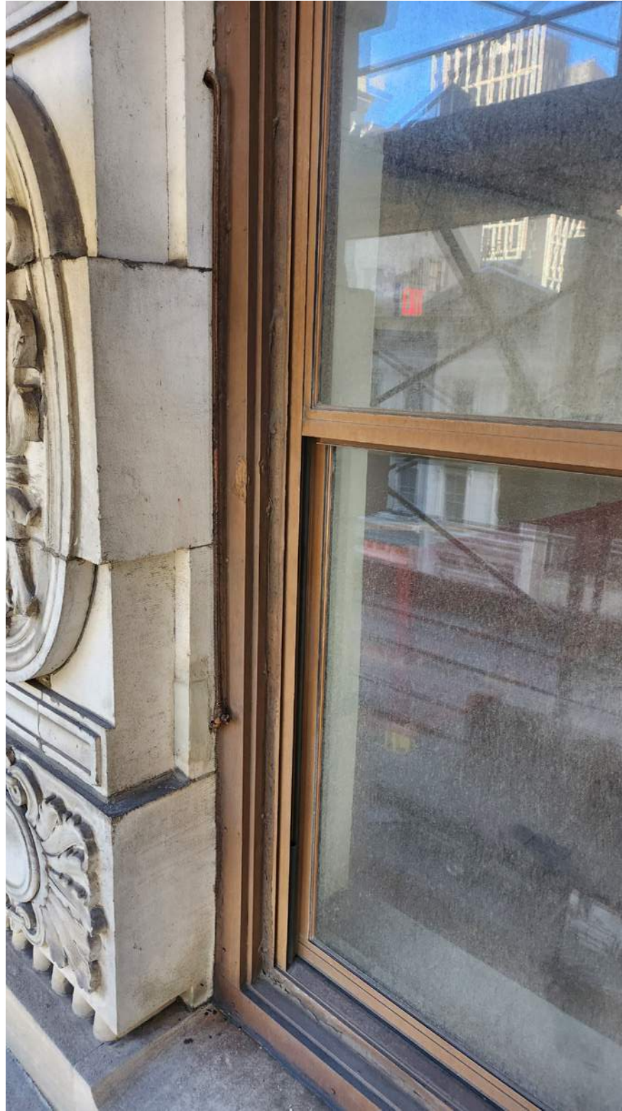
(A) TYPICAL WINDOW PHOTO - 2004 DOUBLE HUNG ALUMINIUM WINDOW REPLACEMENT
