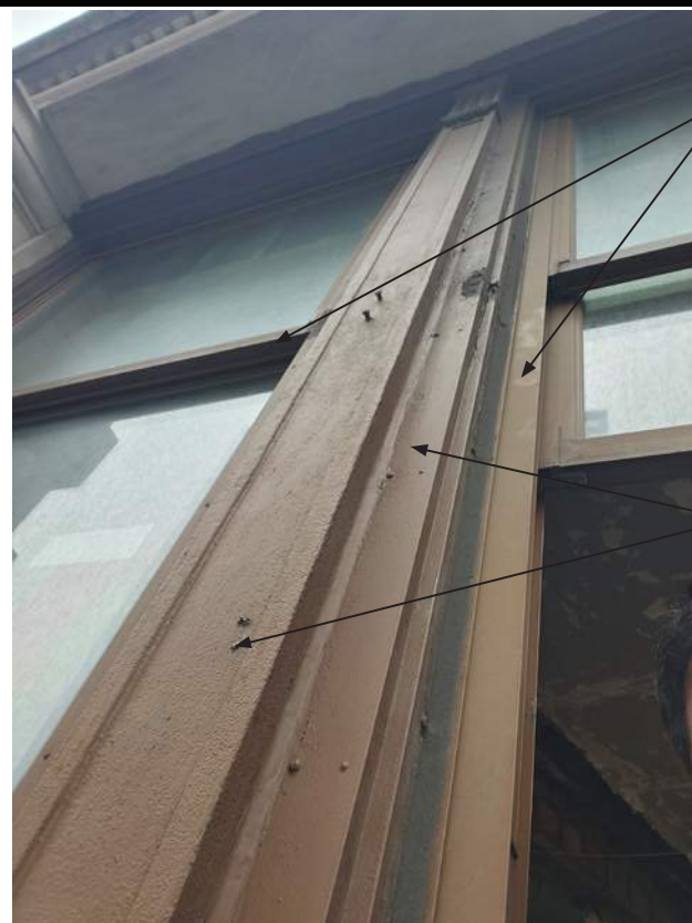
② JAMB DETAIL - EXISTING 2004 DOUBLE HUNG WINDOW
