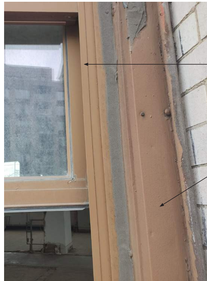
② JAMB DETAIL - EXISTING 2004 DOUBLE HUNG WINDOW
