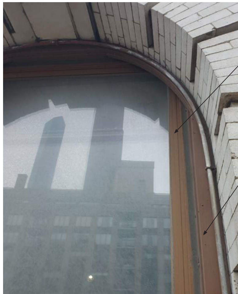
① HEAD DETAIL - EXISTING 2004 DOUBLE HUNG WINDOW
