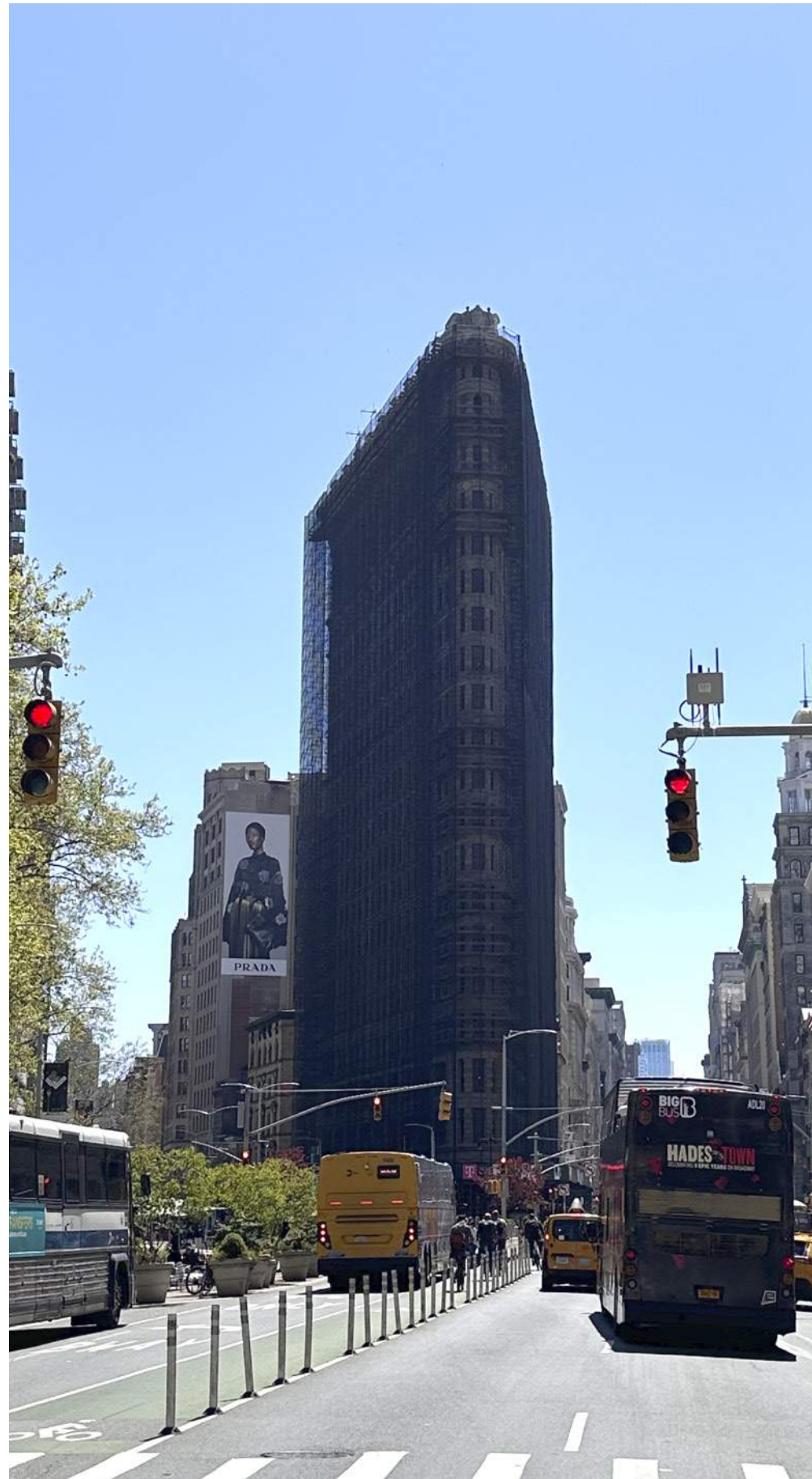
VIEW 5 2024 ROOFTOP MOCKUP
