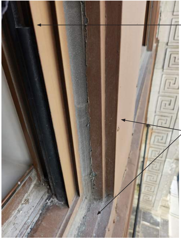
② JAMB DETAIL - EXISTING 2004 DOUBLE HUNG WINDOW
