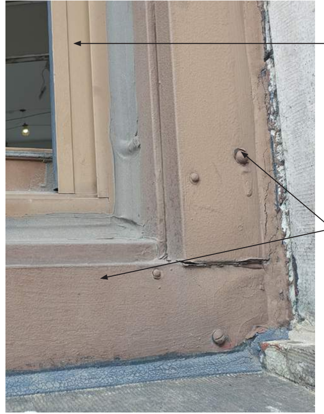
③ SILL DETAIL - EXISTING 2004 DOUBLE HUNG WINDOW
