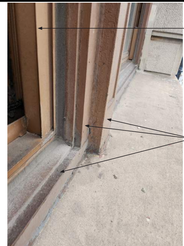
③ SILL DETAIL - EXISTING 2004 DOUBLE HUNG WINDOW
