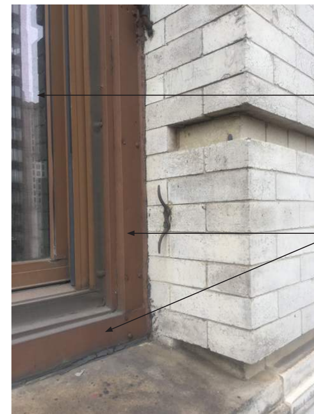
③ SILL DETAIL - EXISTING 2004 DOUBLE HUNG WINDOW
