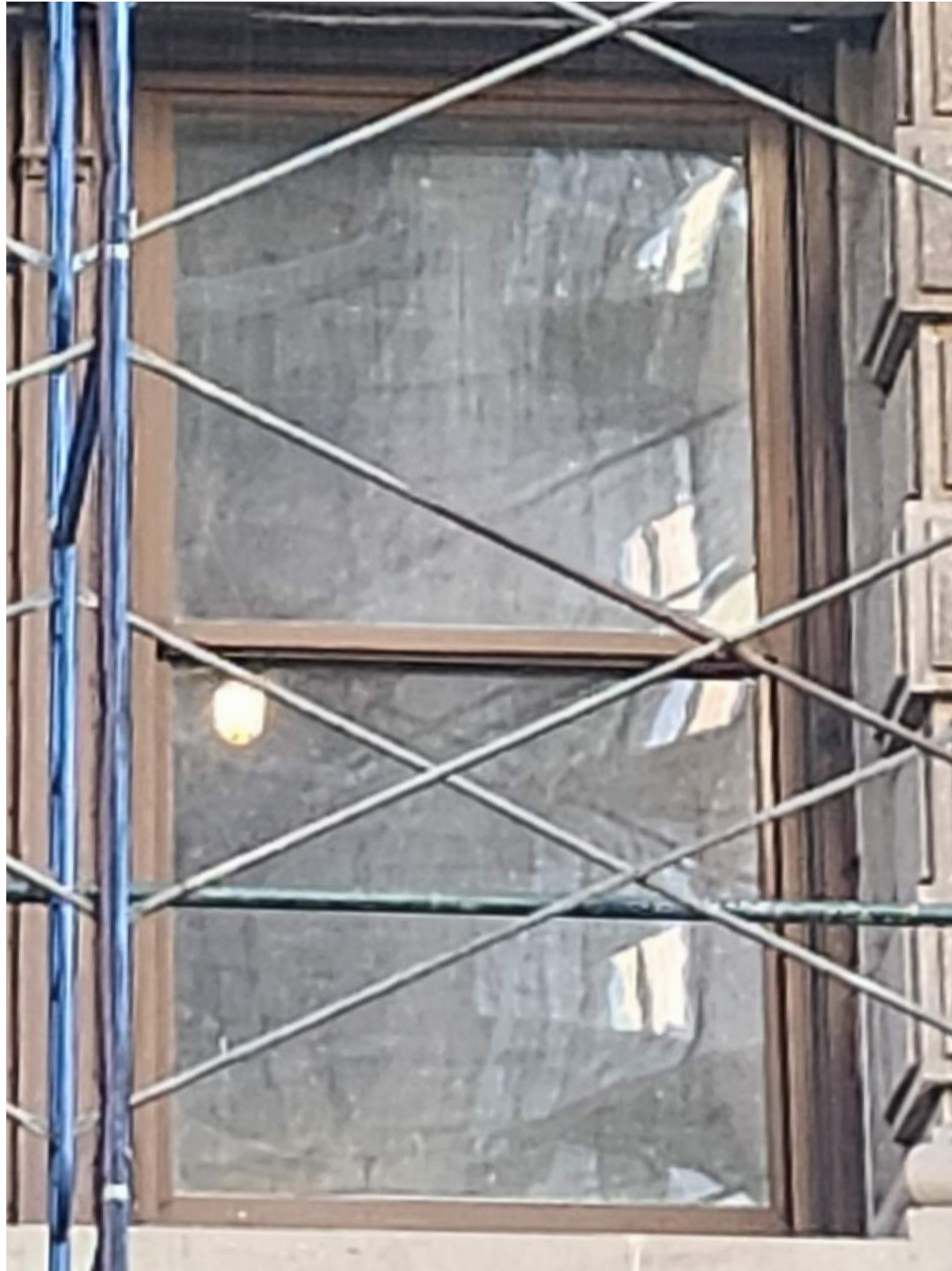
EXTERIOR VIEW FROM BROADWAY
