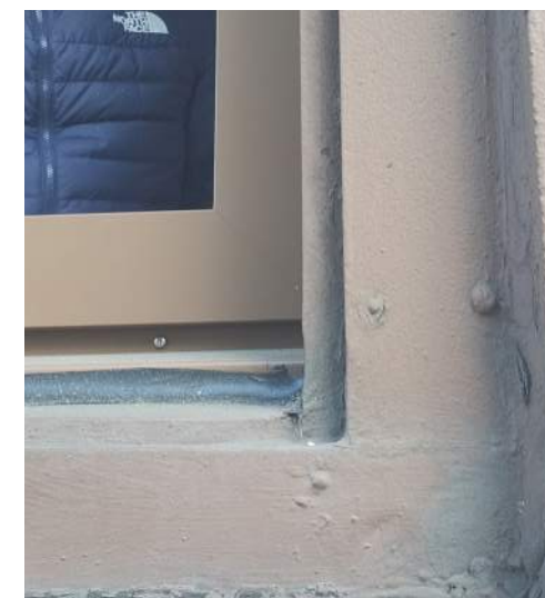
EXTERIOR CLOSE-UP VIEWS
