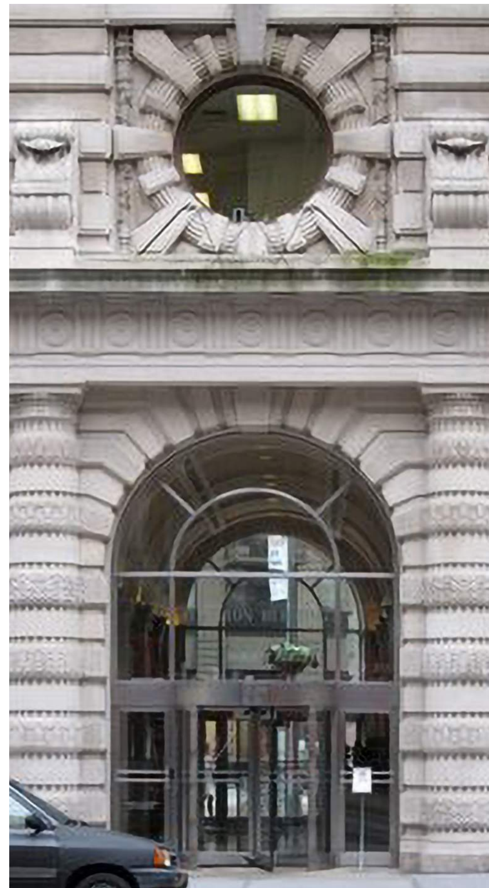
5TH AVENUE ENTRY (1986)
