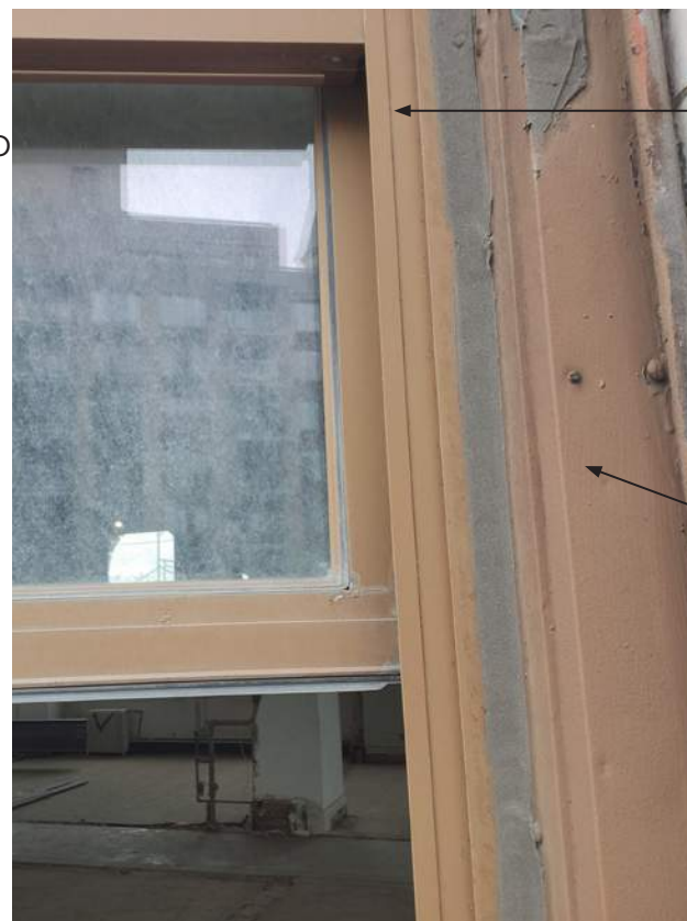
② JAMB DETAIL - EXISTING 2004 DOUBLE HUNG WINDOW
