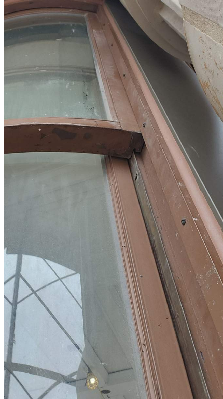
(B) TYPICAL WINDOW PHOTO - 1902 ORIGINAL DOUBLE HUNG WINDOW
