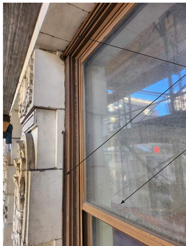
① HEAD DETAIL - EXISTING 2004 DOUBLE HUNG WINDOW
