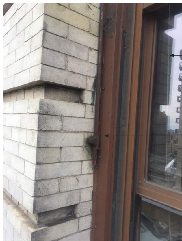
② JAMB DETAIL - EXISTING 2004 DOUBLE HUNG WINDOW
