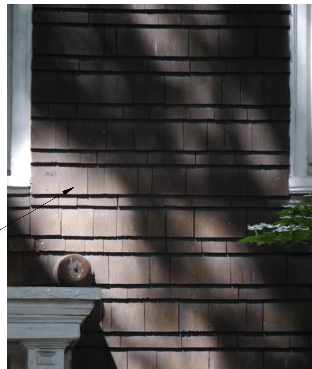
FRONT FACADE 25 CRANBERRY STREET
