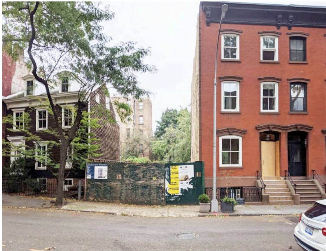
VIEW 1 - 27 CRANBERRY STREET
