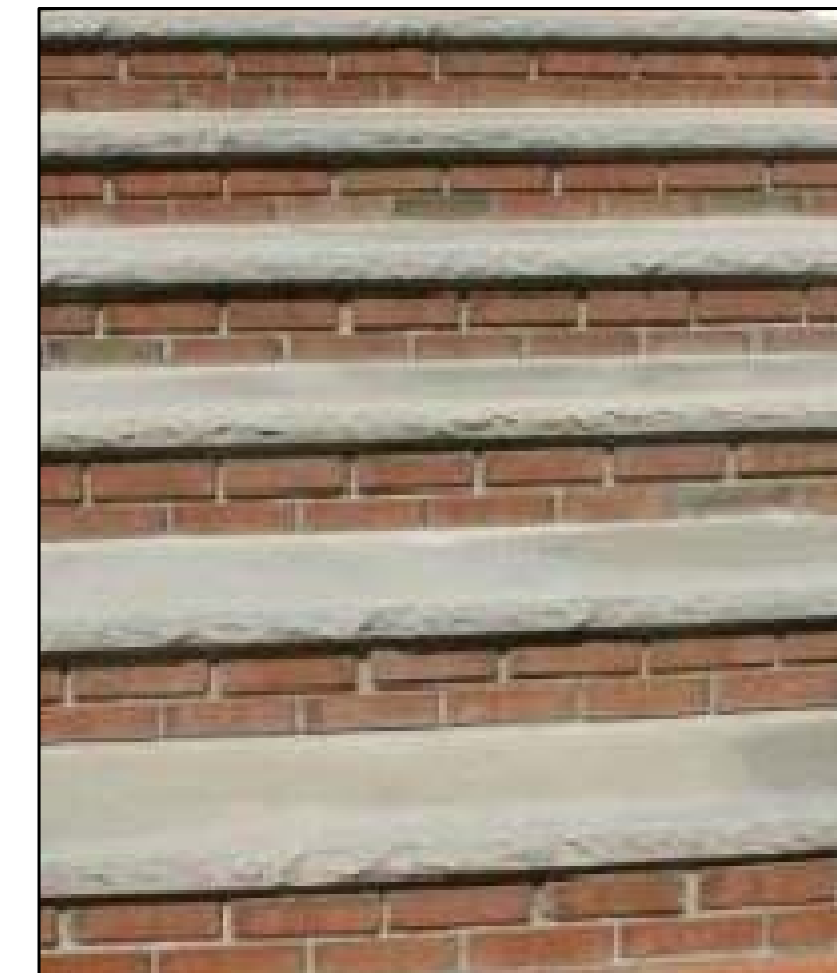
LIMESTONE STEP TREADS @ HOLLYWOOD AVE
