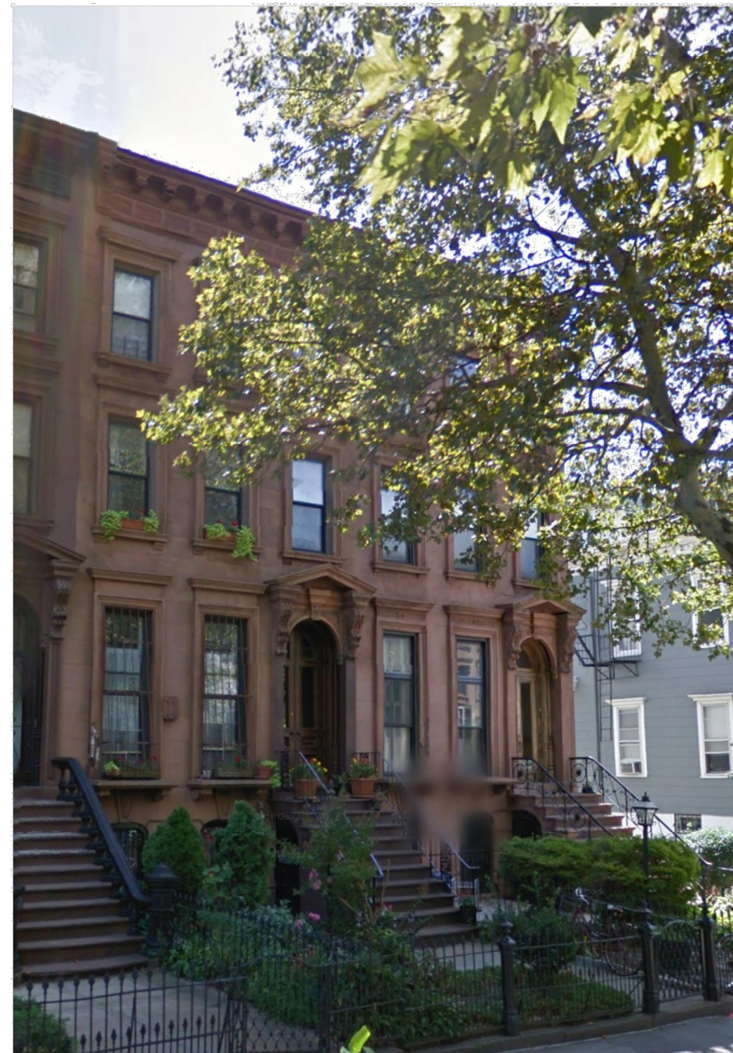
EXISTING FRONT FACADE - NO WORK
