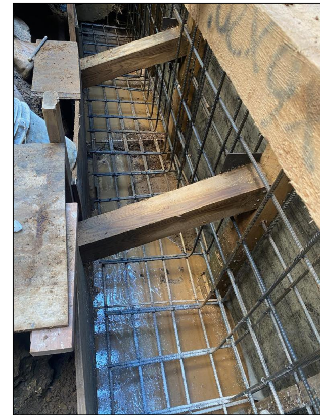
PHOTO OF EXCAVATION AT CELLAR. THIS IS 100% COMPLETED
