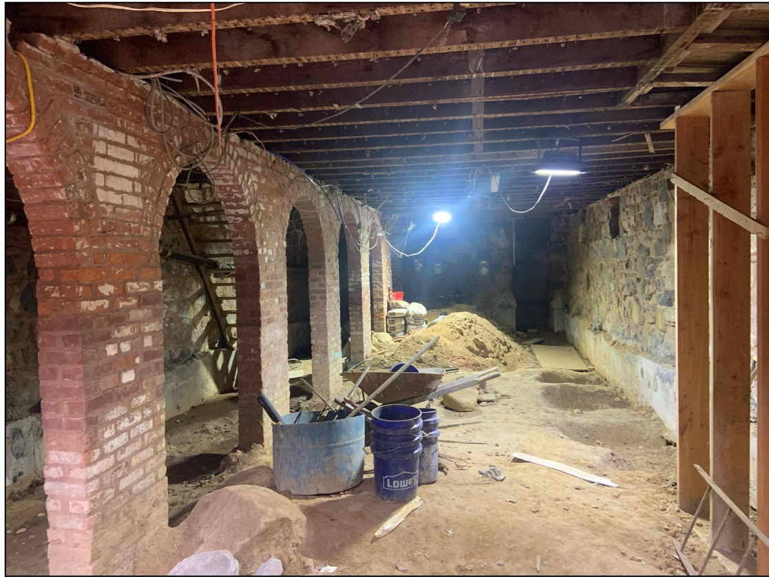
PHOTO OF EXCAVATION AND UNDERPINNING AT CELLAR: THIS IS 100% DONE
