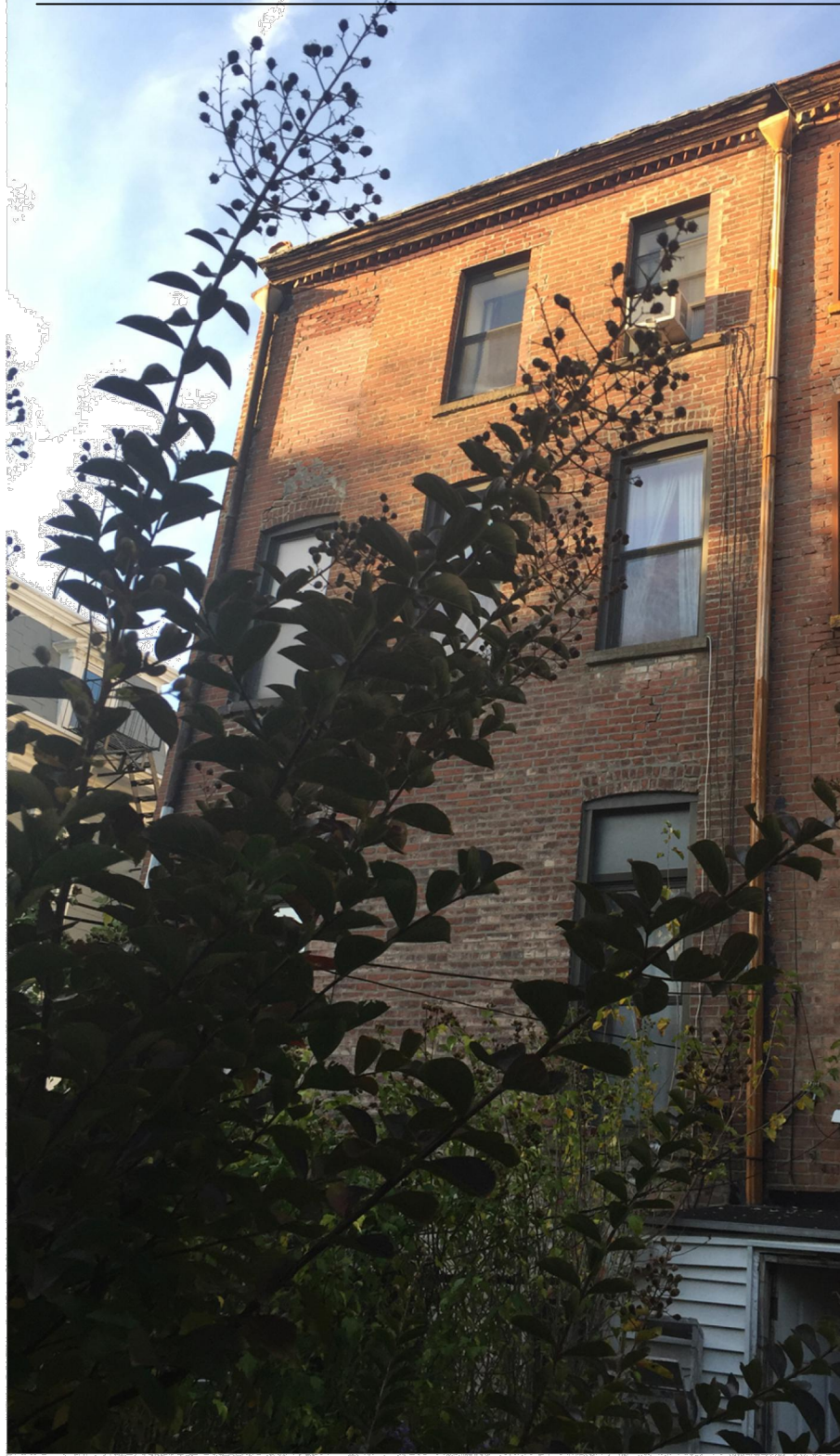
EXISTING REAR FACADE AT 344 MACDONOUGH ST.
