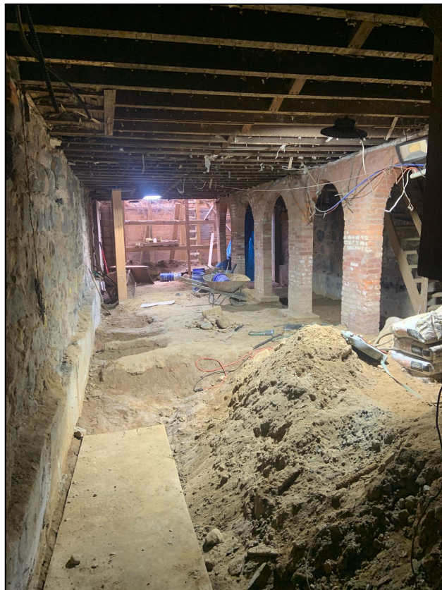
PHOTO OF EXCAVATION AND UNDERPINNING AT CELLAR: THIS IS 100% DONE
