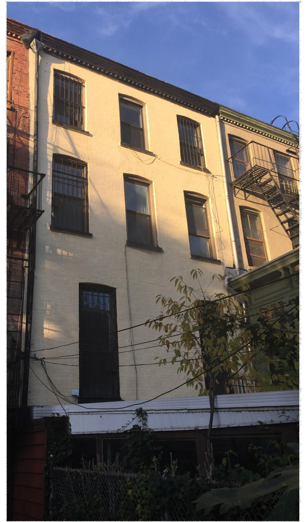
EXISTING REAR FACADE AT 348 MACDONOUGH ST.
