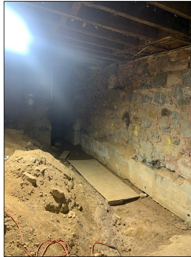
PHOTO OF UNDERPINNING AT CELLAR: THIS IS 100% DONE
