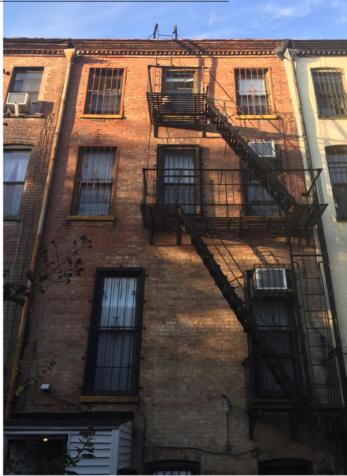
EXISTING REAR FACADE AT 346 MACDONOUGH ST.
