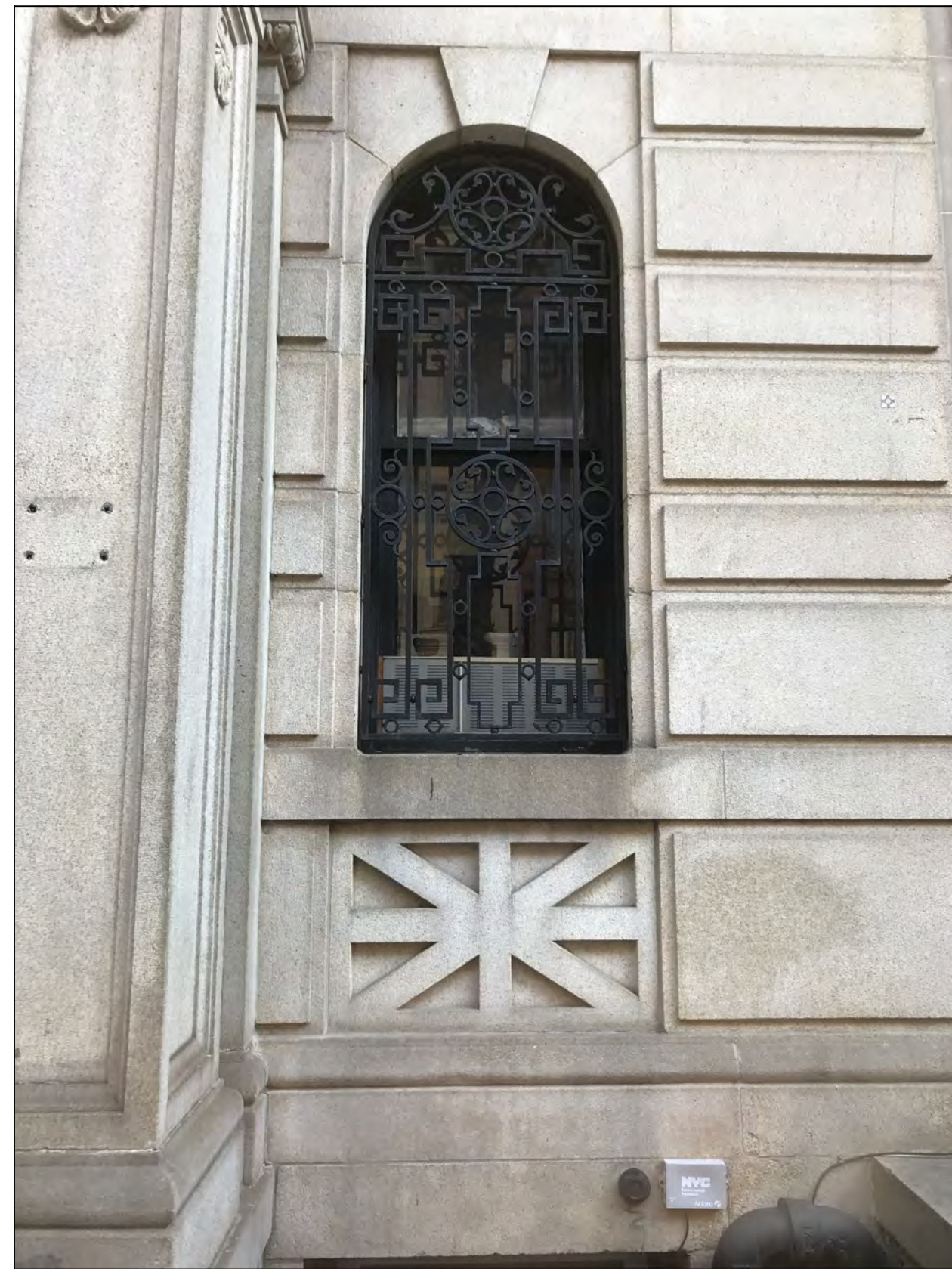
PHOTO OF 1ST FLOOR WINDOW
