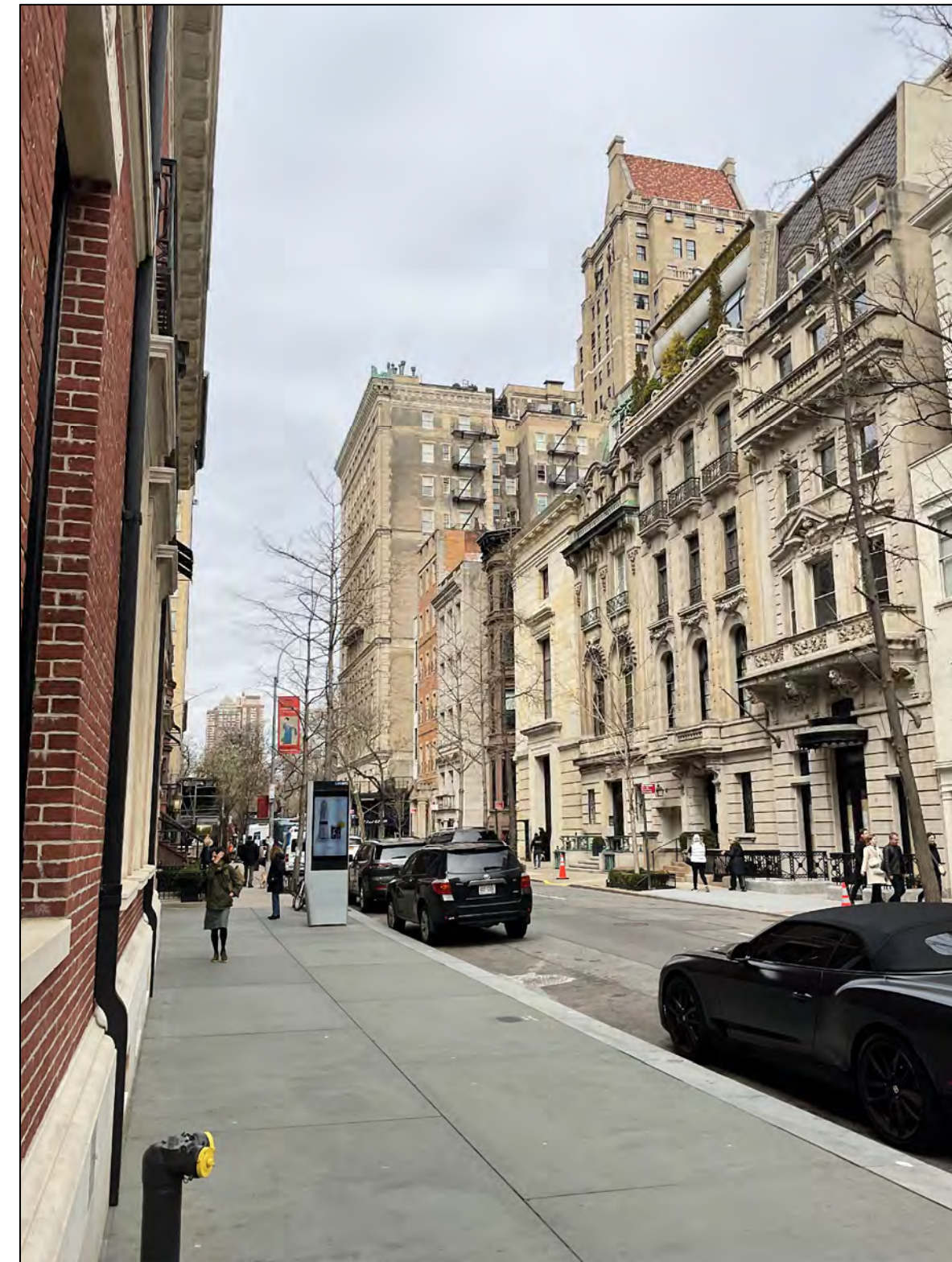
PHOTO 4 - VIEW FROM SOUTHEAST CORNER OF EAST 63RD STREET - BULKHEAD NOT VISIBLE
