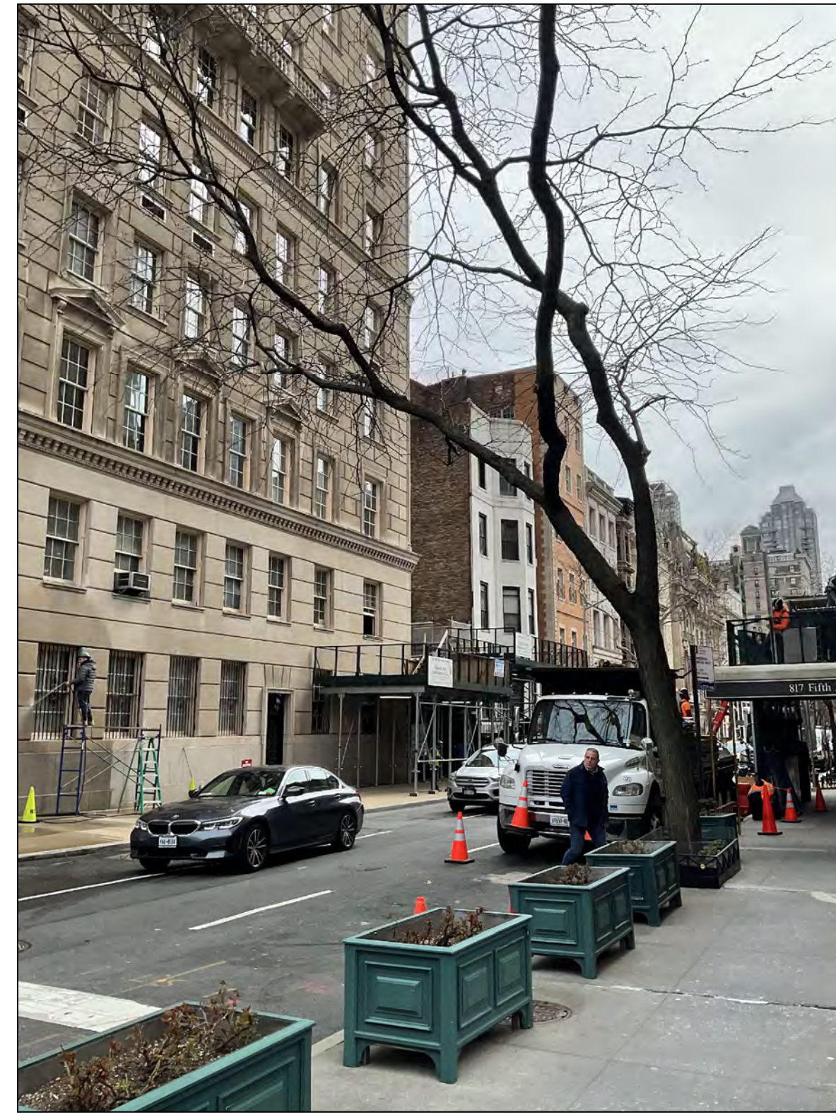
PHOTO 3 - VIEW FROM SOUTHWEST CORNER OF EAST 63RD STREET
