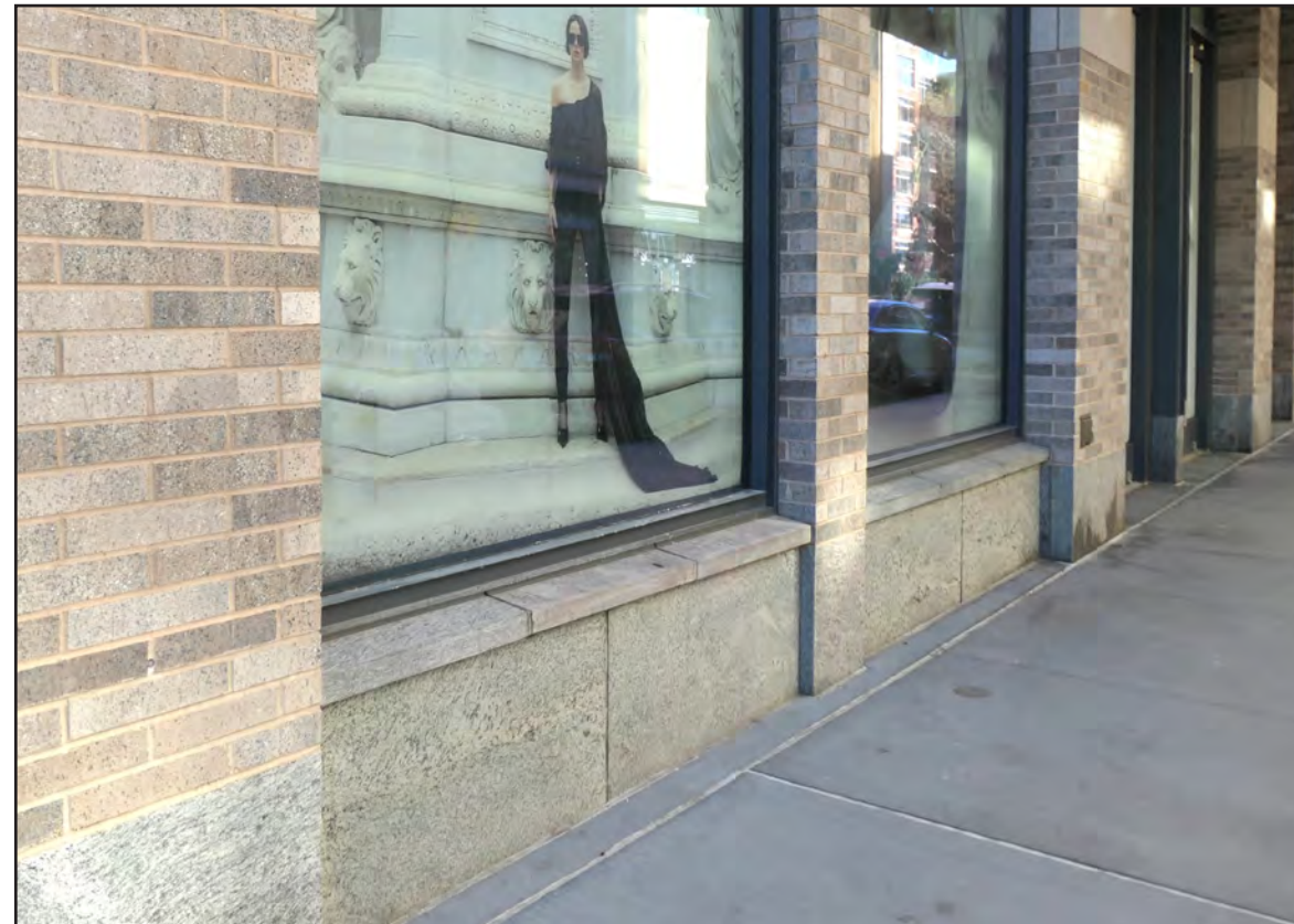
STOREFRONT DETAIL ALONG WASHINGTON STREET
