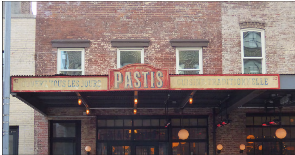
52 GANSEVOORT STREET, PANEL SIGNAGE, APPROVED 2019
