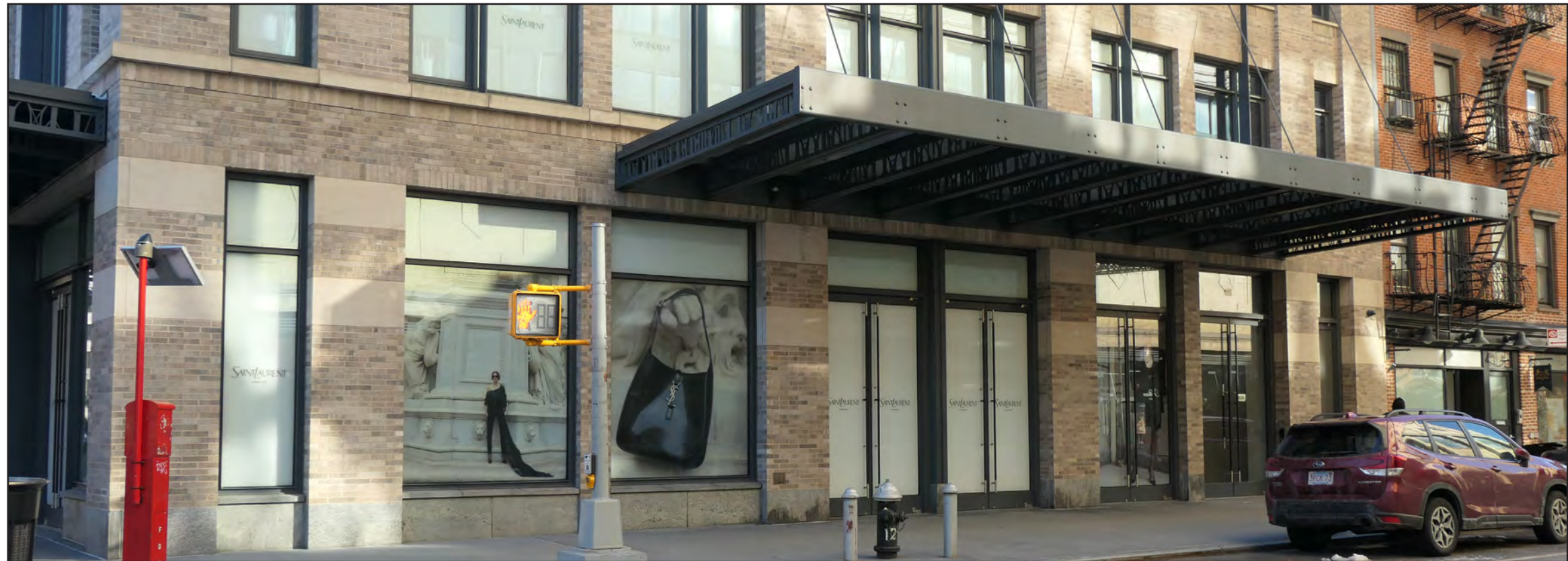
WASHINGTON STREET FACADE - EXISTING CONDITION
