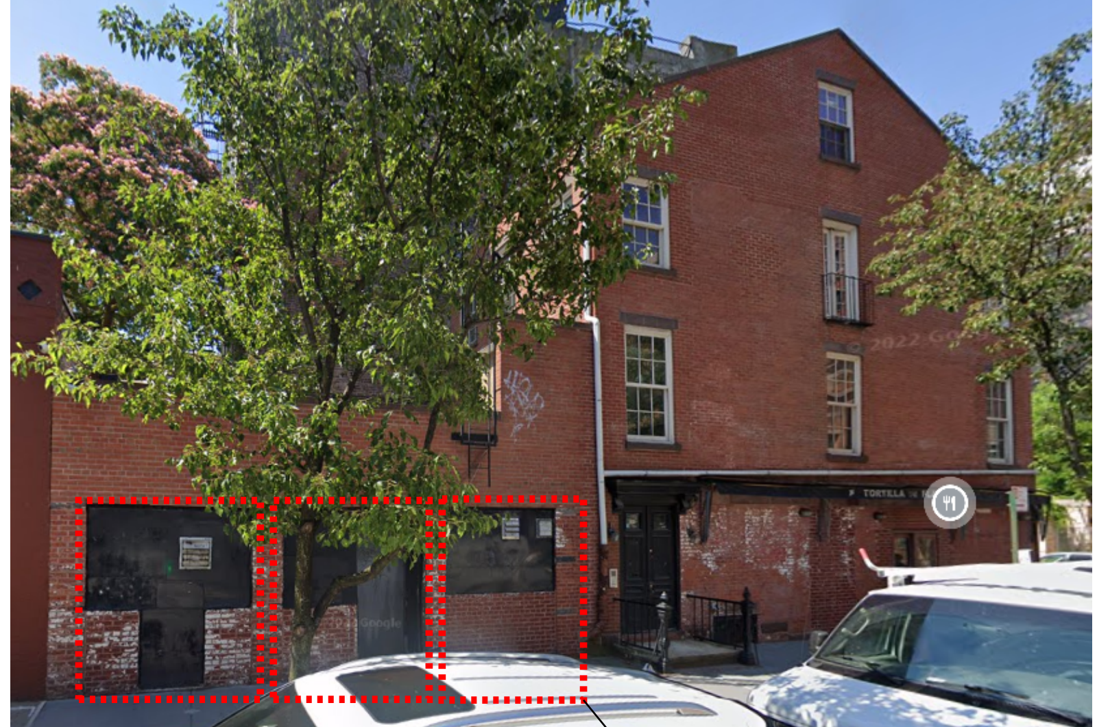
Infill masonry and steel panels previously approved for removal, under #CNE-132234
