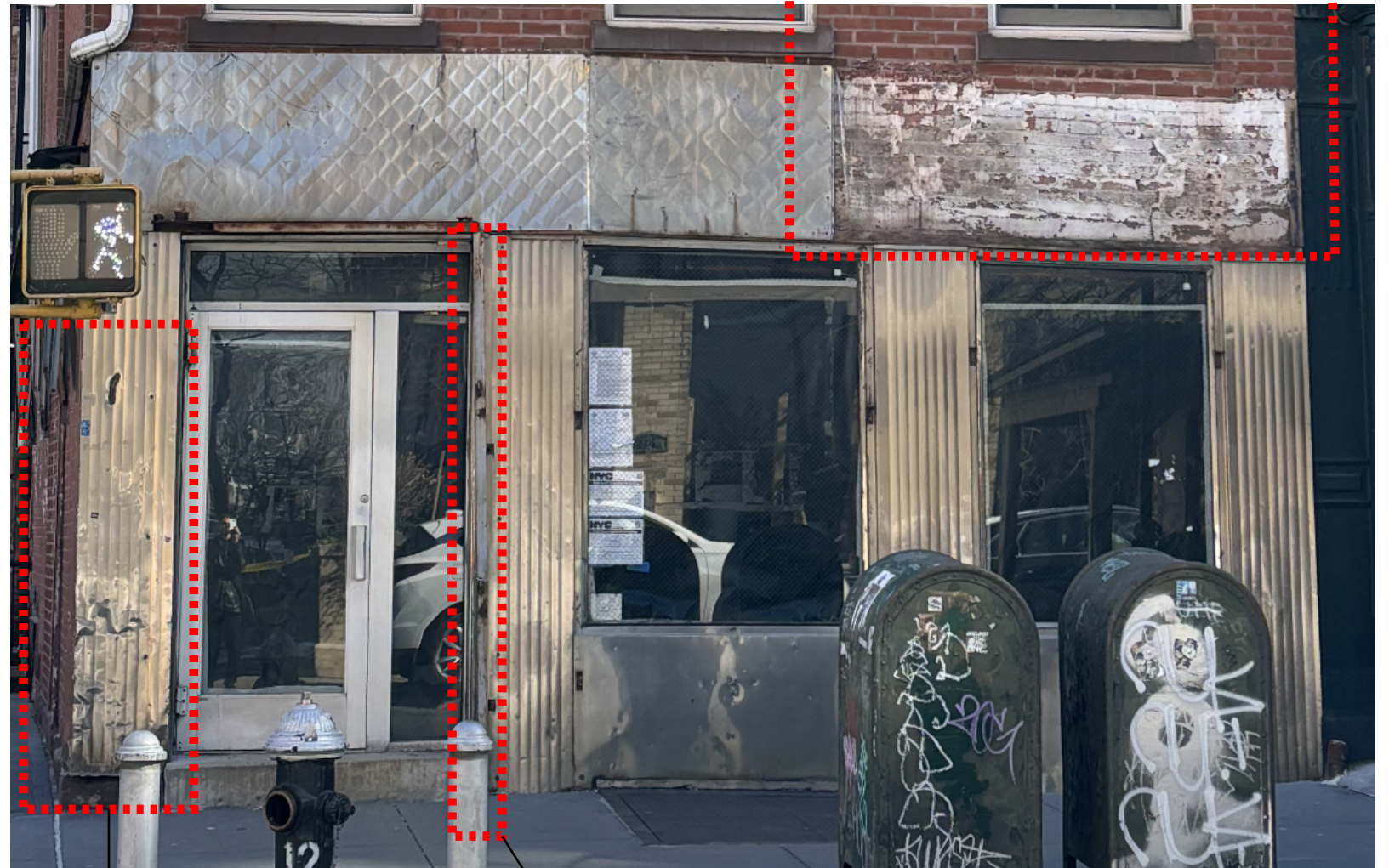
Stainless steel cladding severely dented, with exposed fasteners and missing base trim in potentially hazardous condition
