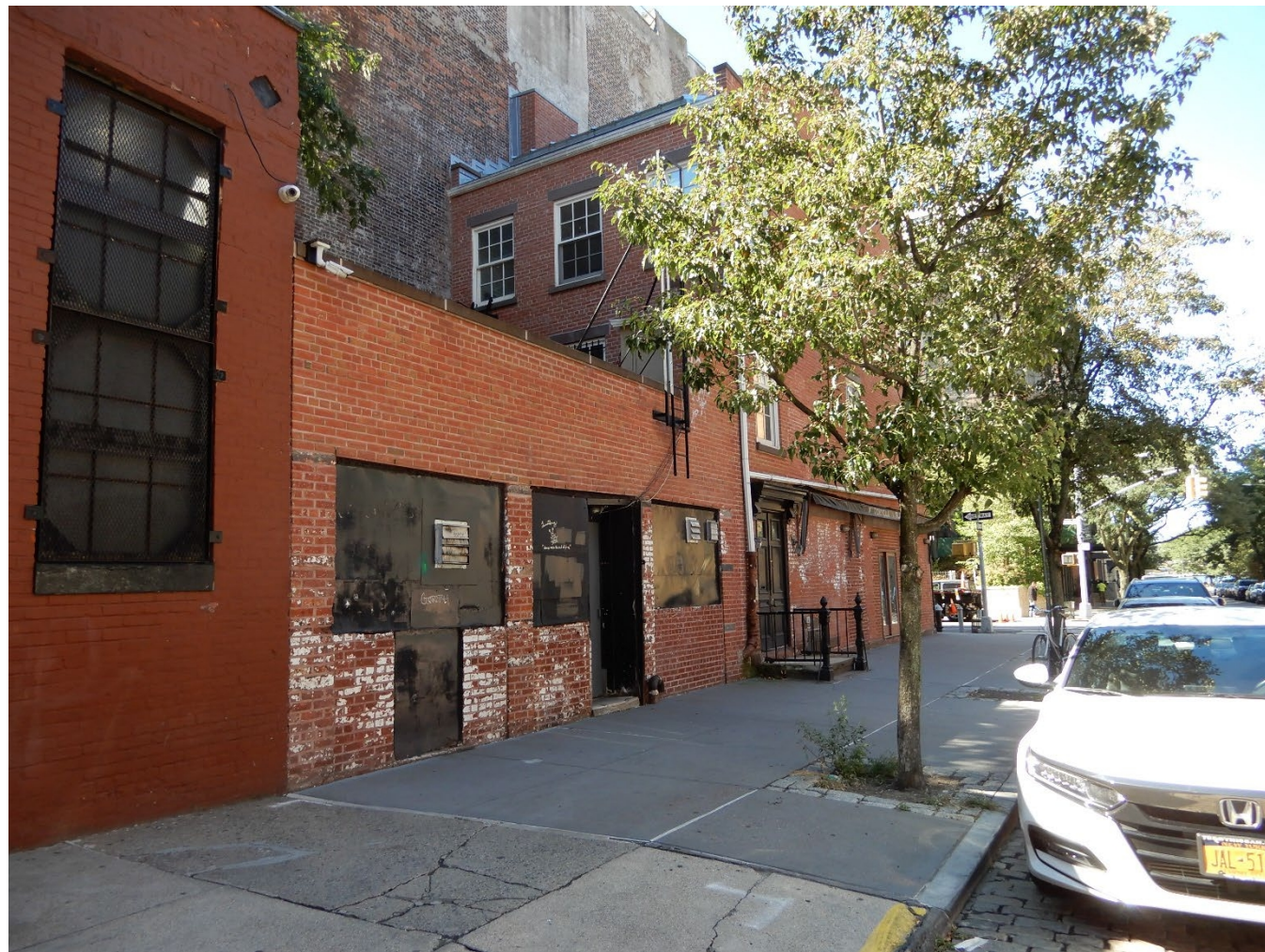
West 12th Street, Looking West
