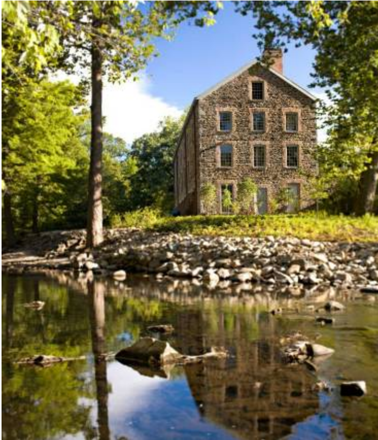
Restoration of the Lillian and Amy Goldman Stone Mill, a historic, pre-Civil War industrial building.
