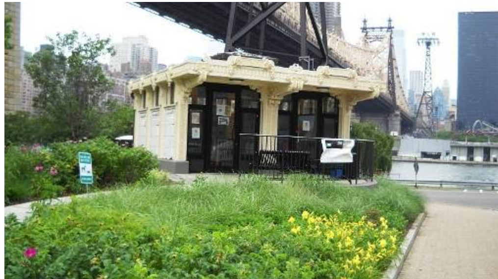
Newly-Restored Roosevelt Island Historical Society Visitors Kiosk, which stripped away a layer of century-old paint to reveal cast iron and copper materials
