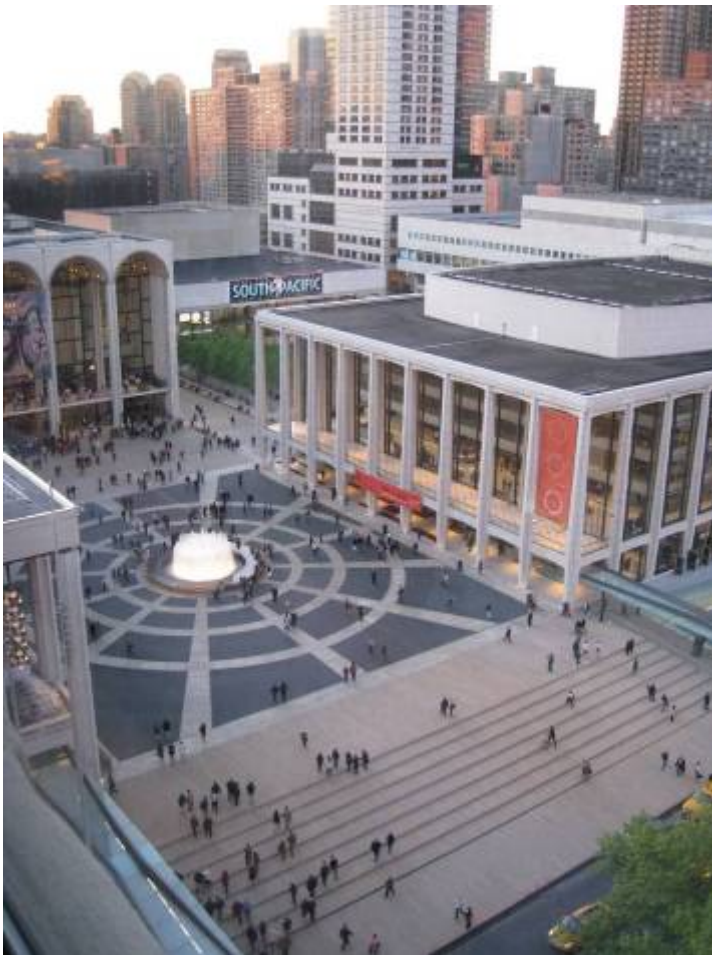
The Lincoln Center Campus Renovation is near complete. The aim was to open and update the space to the general public.
